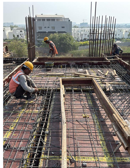
sunken shuttering work in progress
