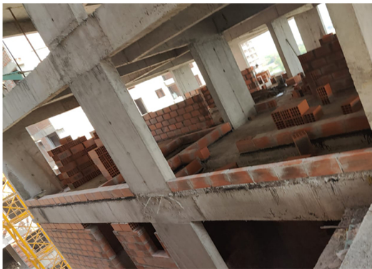
block work on the 9th floor sill
