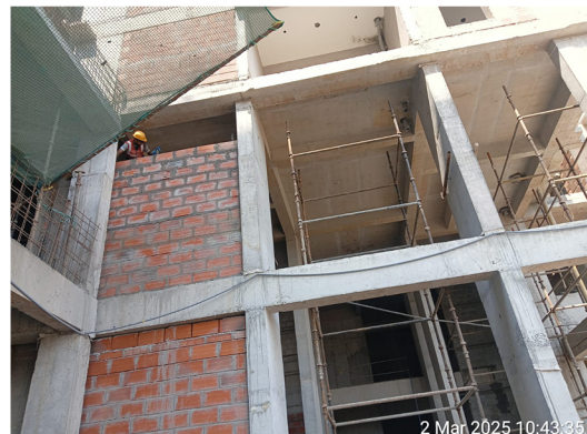
double height area block work have been completed
