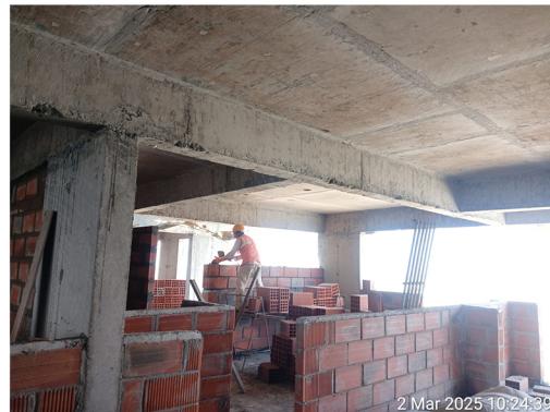
block works for all the flats in the 9th floor
