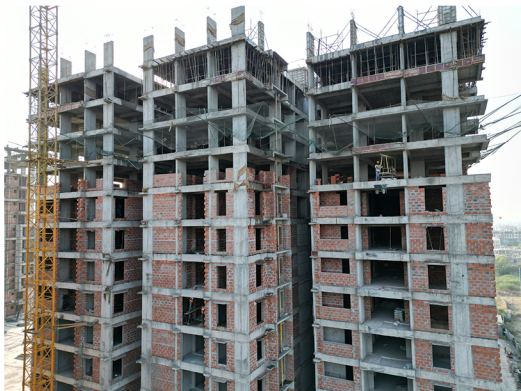
the structure is taking shape with the block work clearly visible across all floors.
