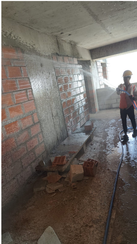
curing of the block works
