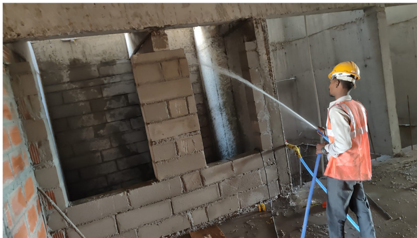
curing of the completed portion of corridor
