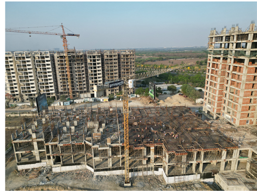
shuttering for columns for 1st floor slab in tower
