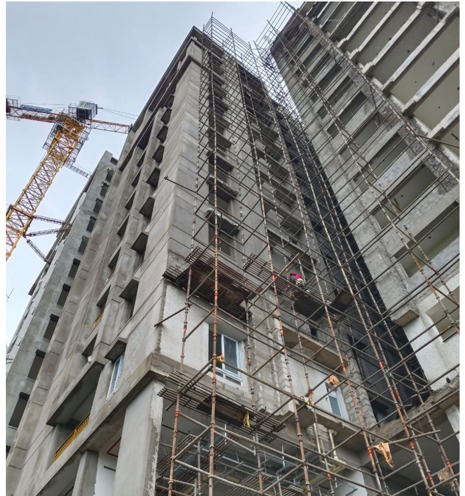
North side external plastering work is in progress.
