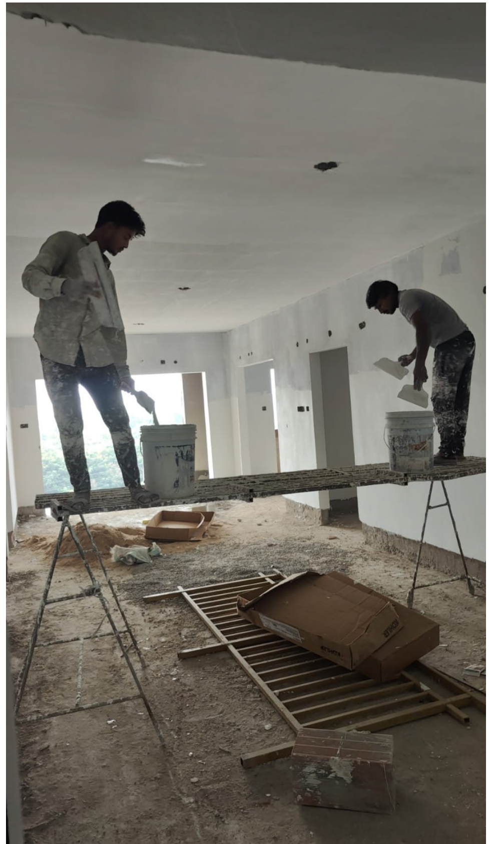
Putty works and 2nd coat of painting is going on in the 11th Floor flats.
