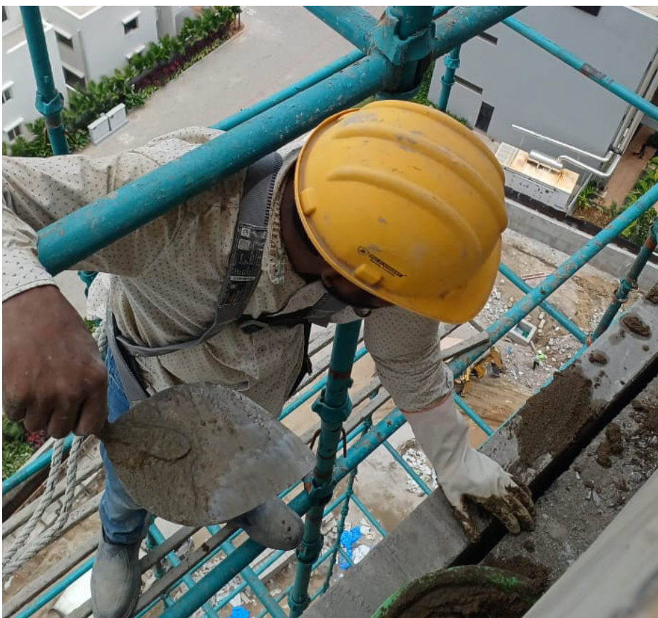
External pin brick work is in progress.
