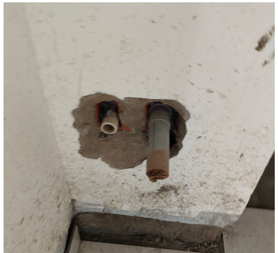
Packing of the plumbing lines, gas pipeline and the skirting packing is being done.
