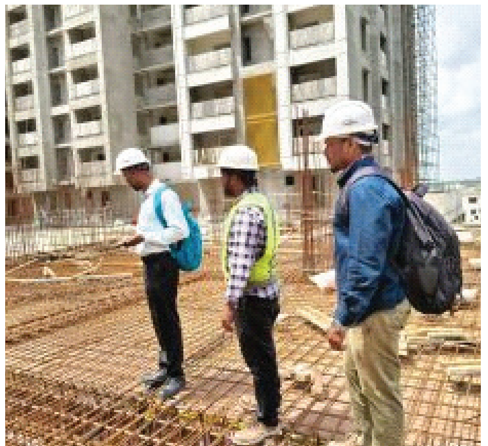
A QC check is being carried out on the reinforcement before concreting the slab and PT beams at the upper slab level.
