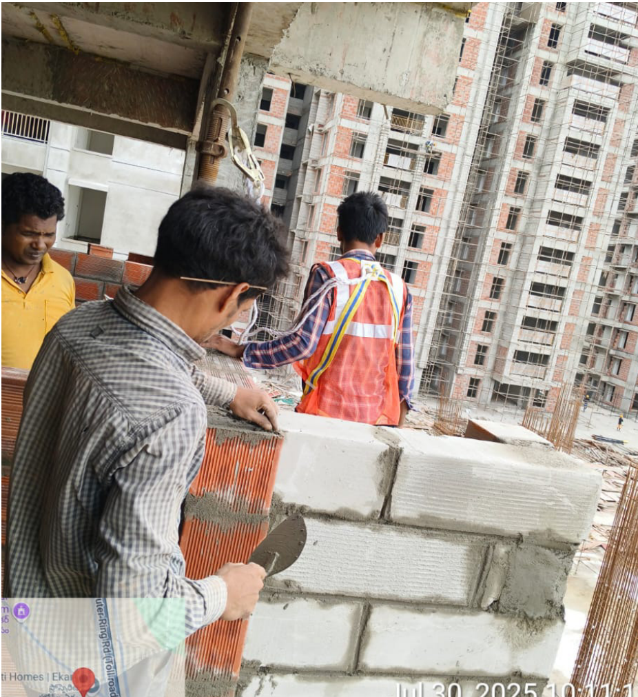
Sill level brick work in progress in 3rd floor.
