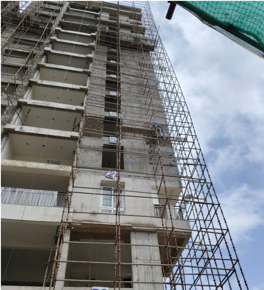
Coarse external plastering work is in progress.
