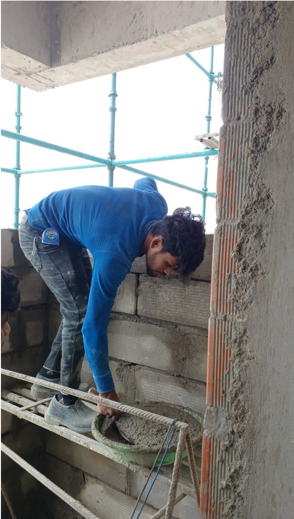
Internal plastering works in Utility area is in progress.
