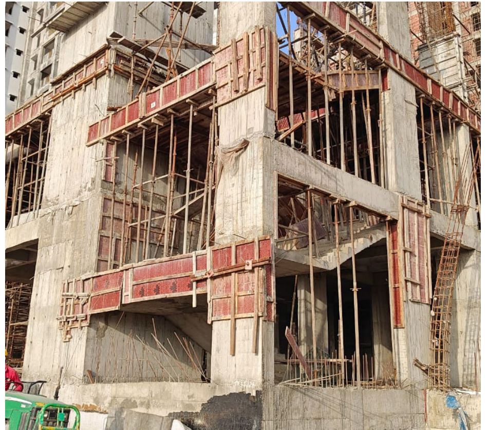
Shuttering works are going on for the wall of the fire lift.
