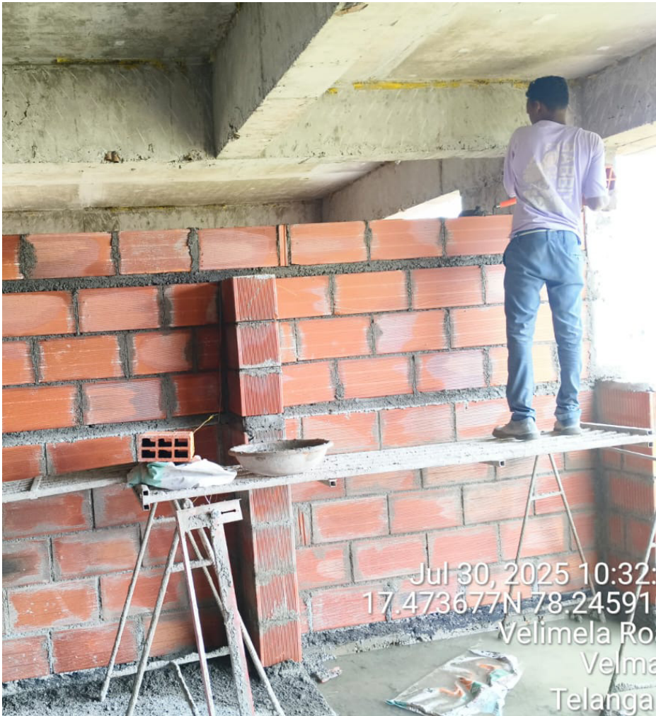
Above sill work in progress.
