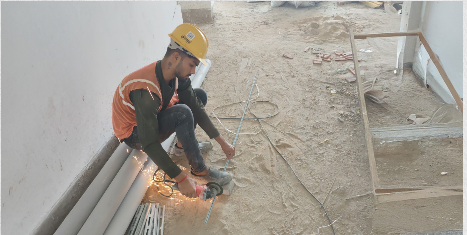
Workers are using handheld angle grinders to cut steel wires and rods in preparation for plumbing installations.
