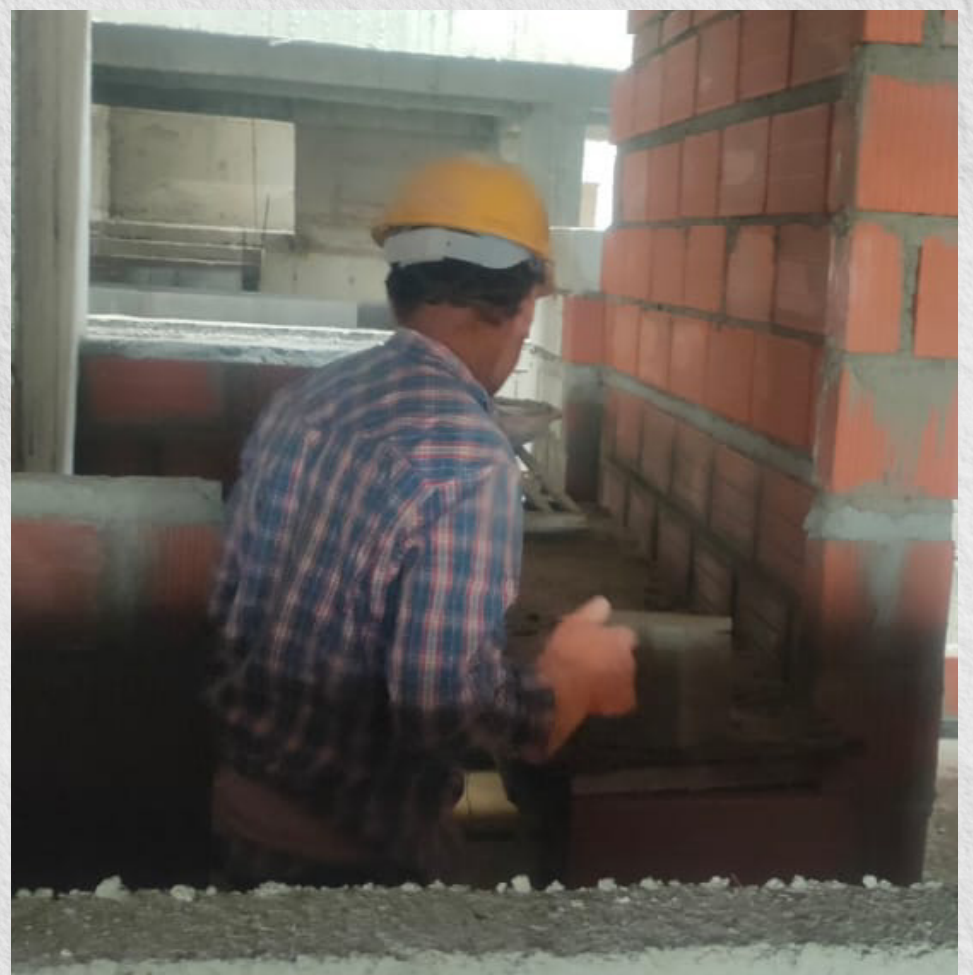
7th Floor flat sill work level block work in progress.
