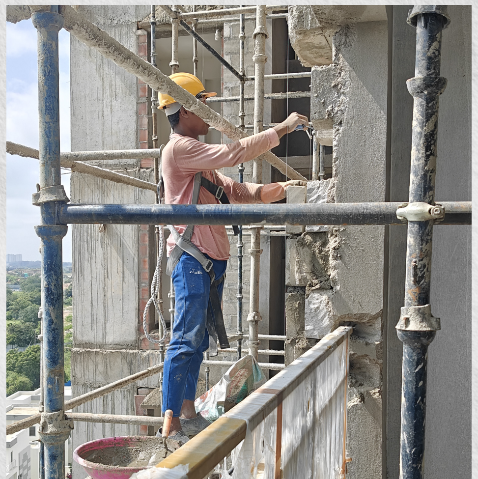
South side elevation pins brick work in progress.
