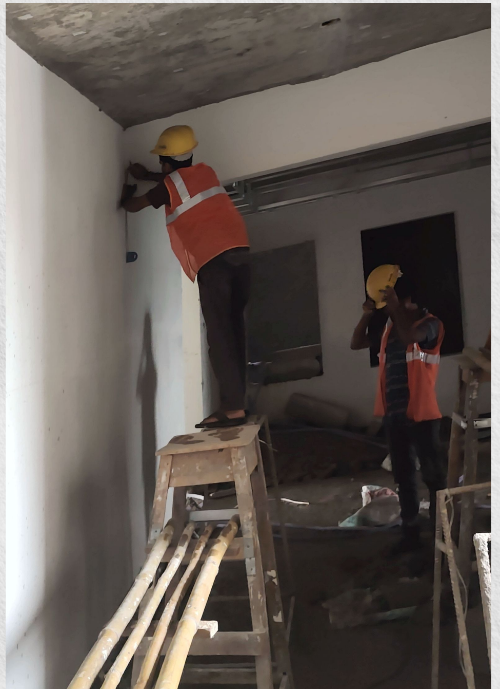
Walls and ceilings are being prepared to route electrical wiring for upcoming electrical fixtures and gadgets.
