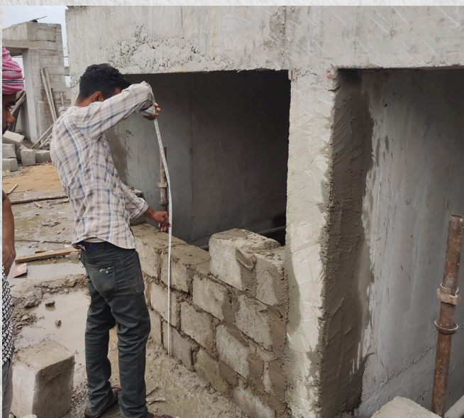
Plastering works on the lift shaft walls at the terrace level are in progress.
