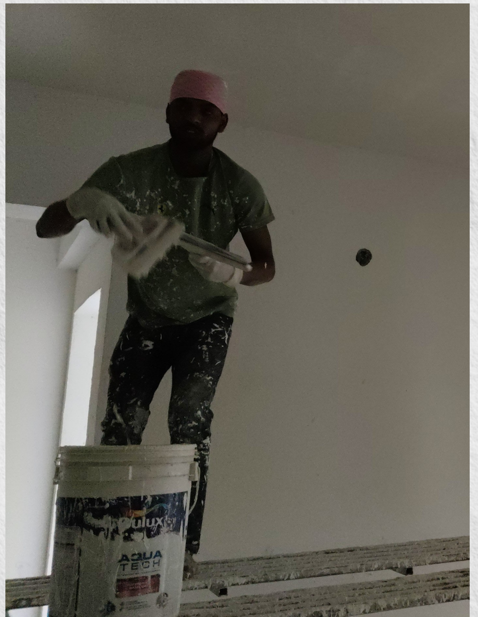
2nd coat of putty work in progress.
