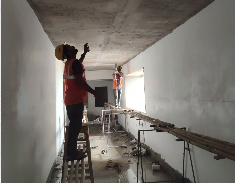
Mapping the ceiling in the corridor to accommodate electrical fittings and fixtures.
