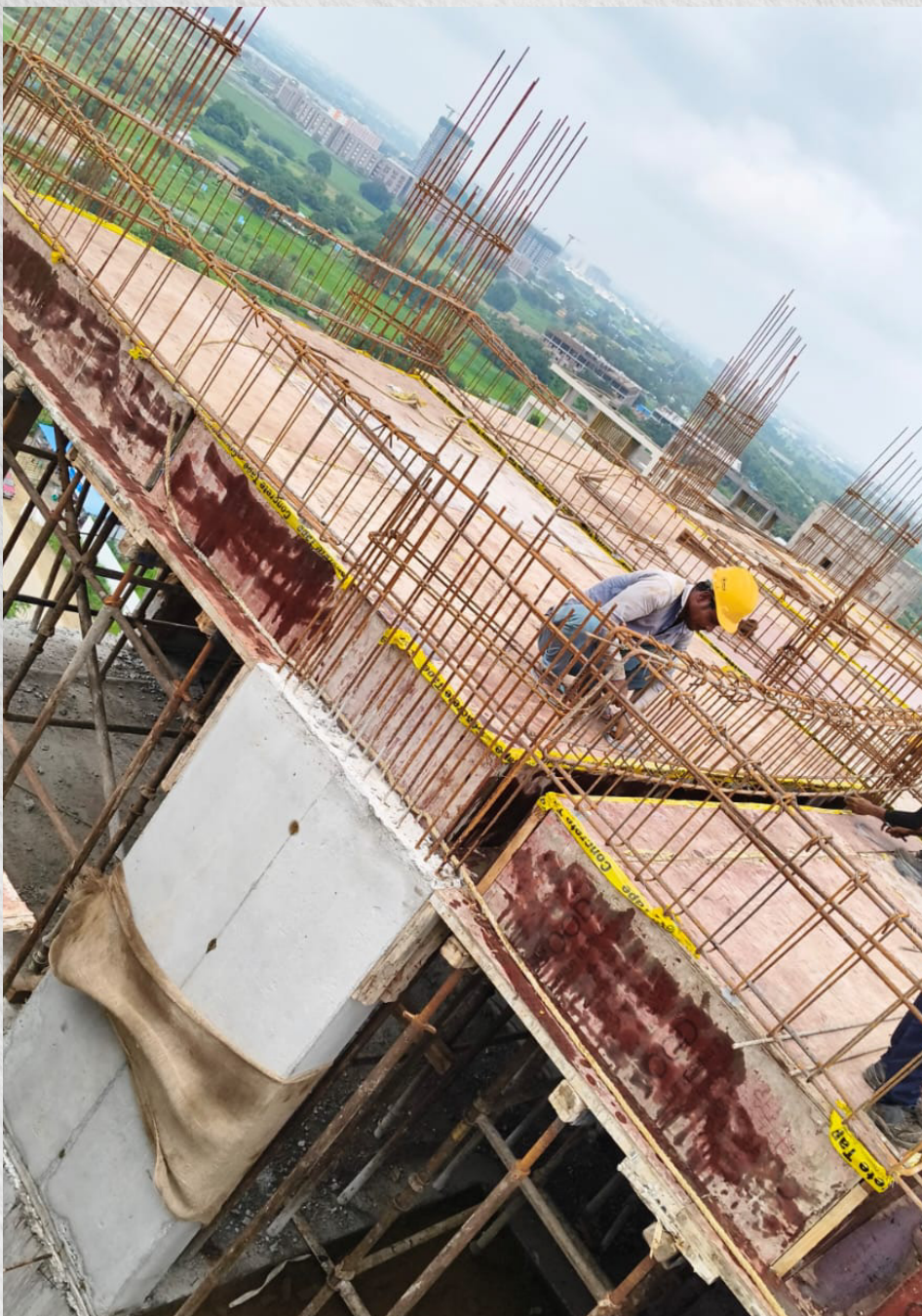
Slab reinforcement work in progress.
