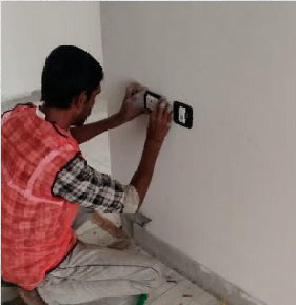
Wiring and Installation of Electrical Switchboards in Progress.
