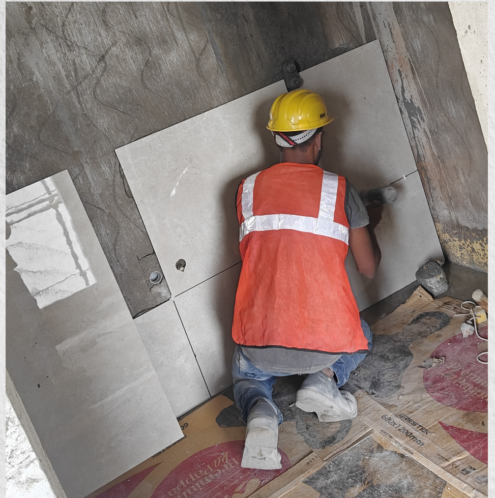
Tiling works in progress in the bathrooms.
