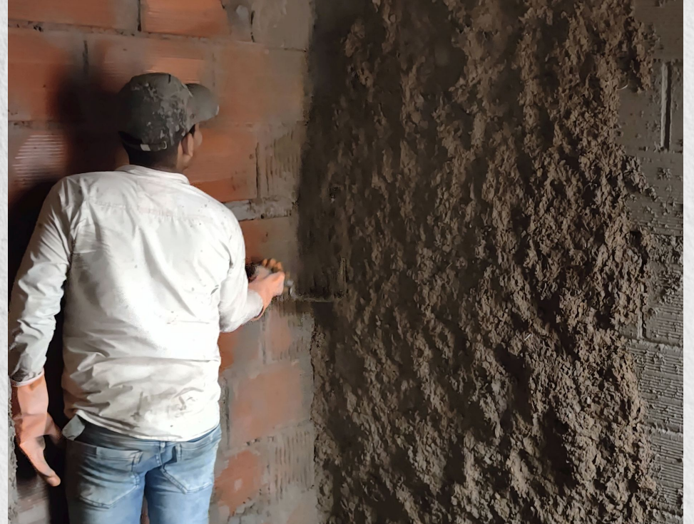
Internal Plastering work is going on in a few flats.
