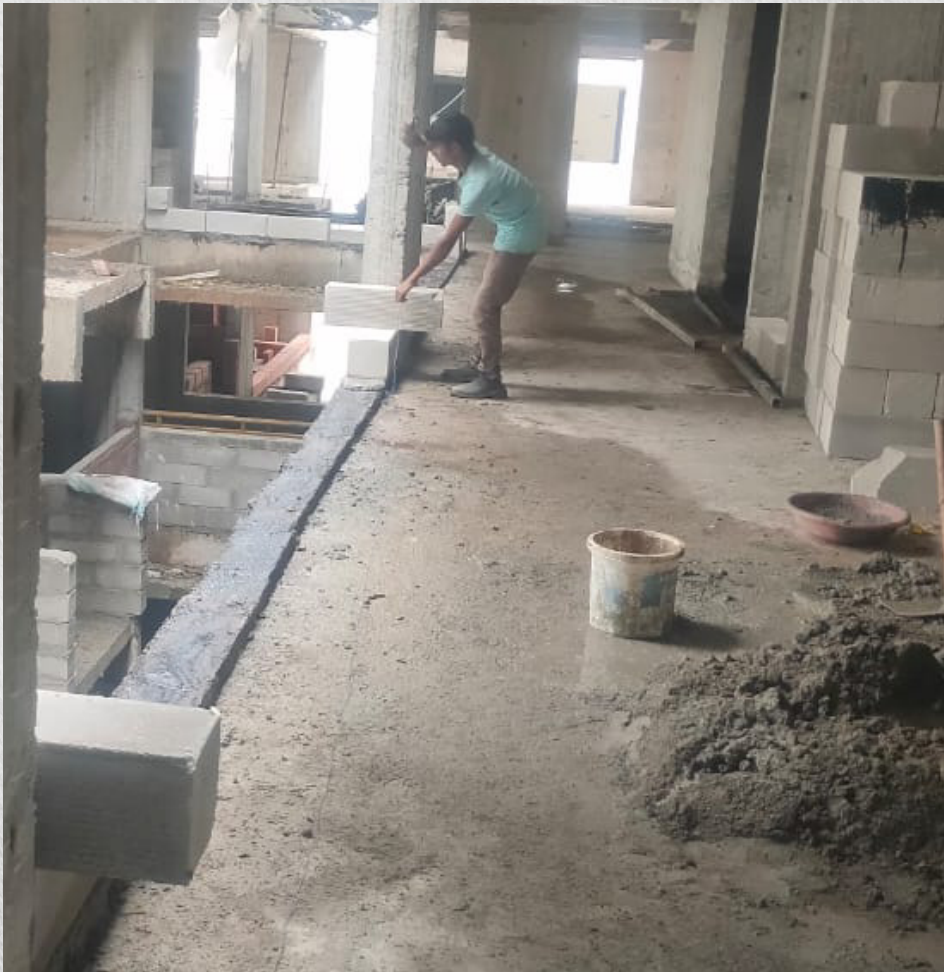
Layout marking for 8th floor corridor area.
