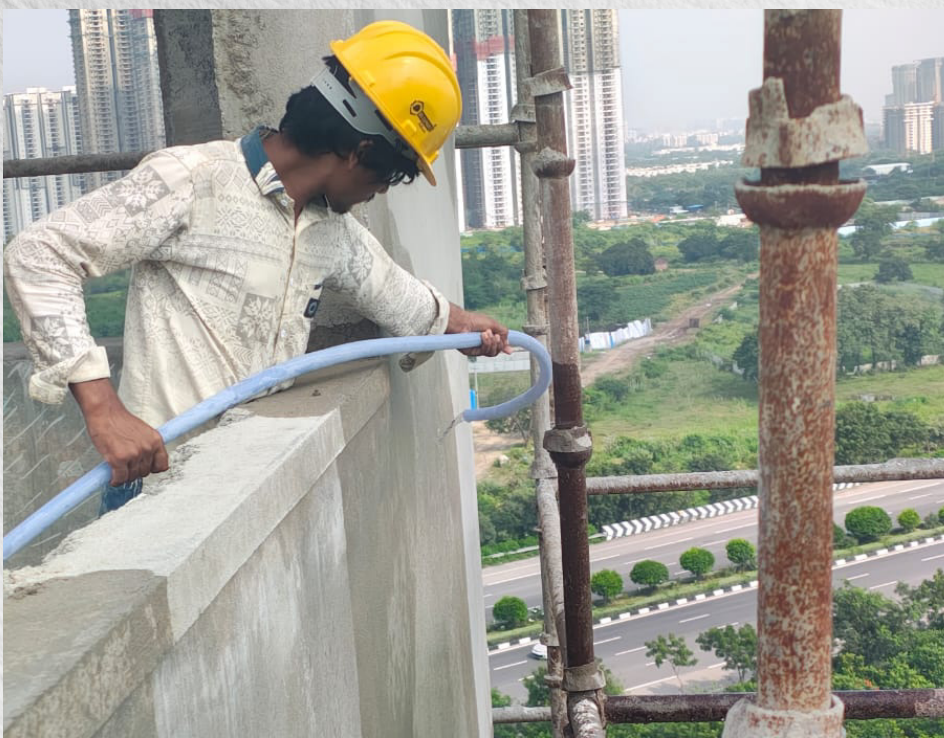
Curing of South Face external Plastering.
