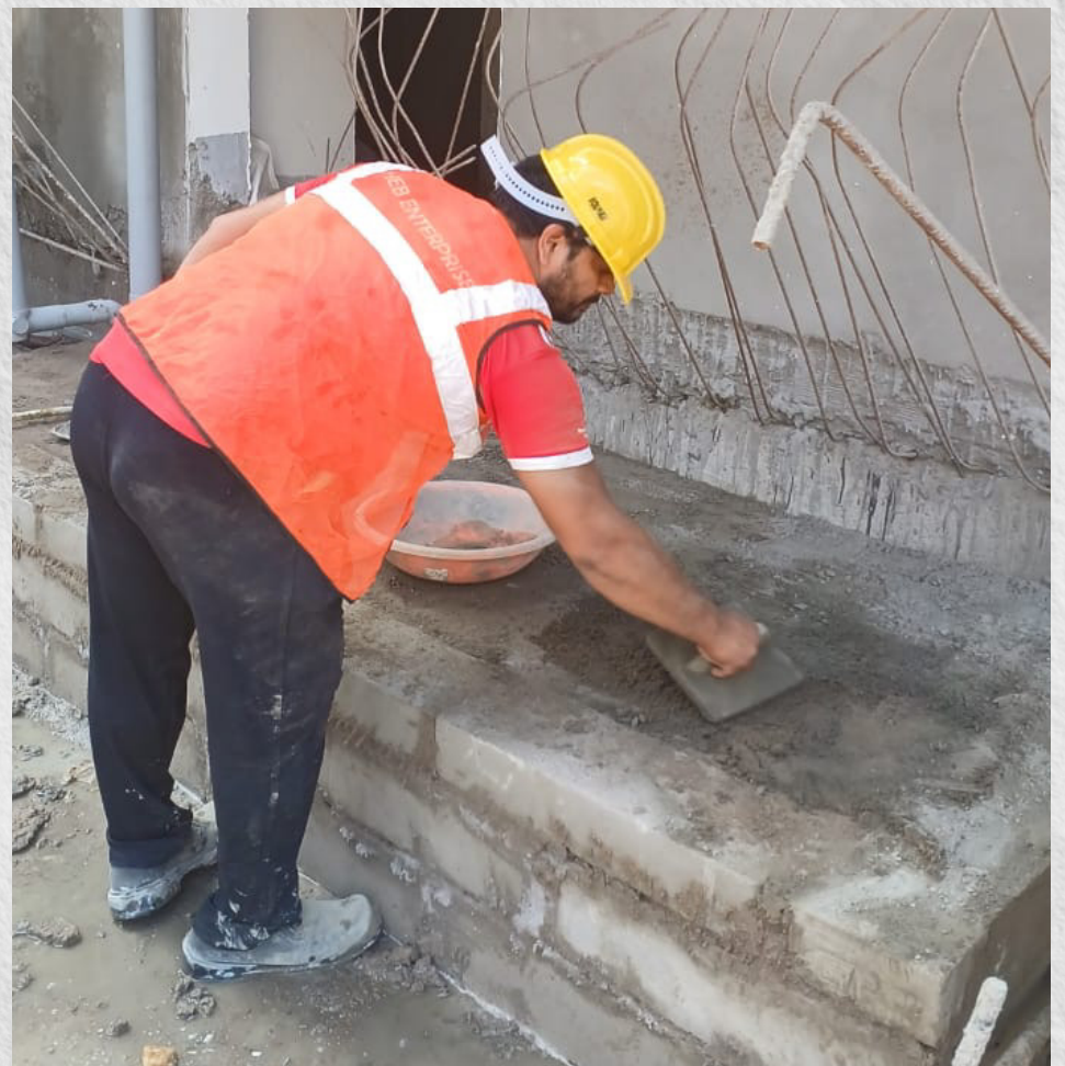
Brick work is going on in the first Floor Balcony area.
