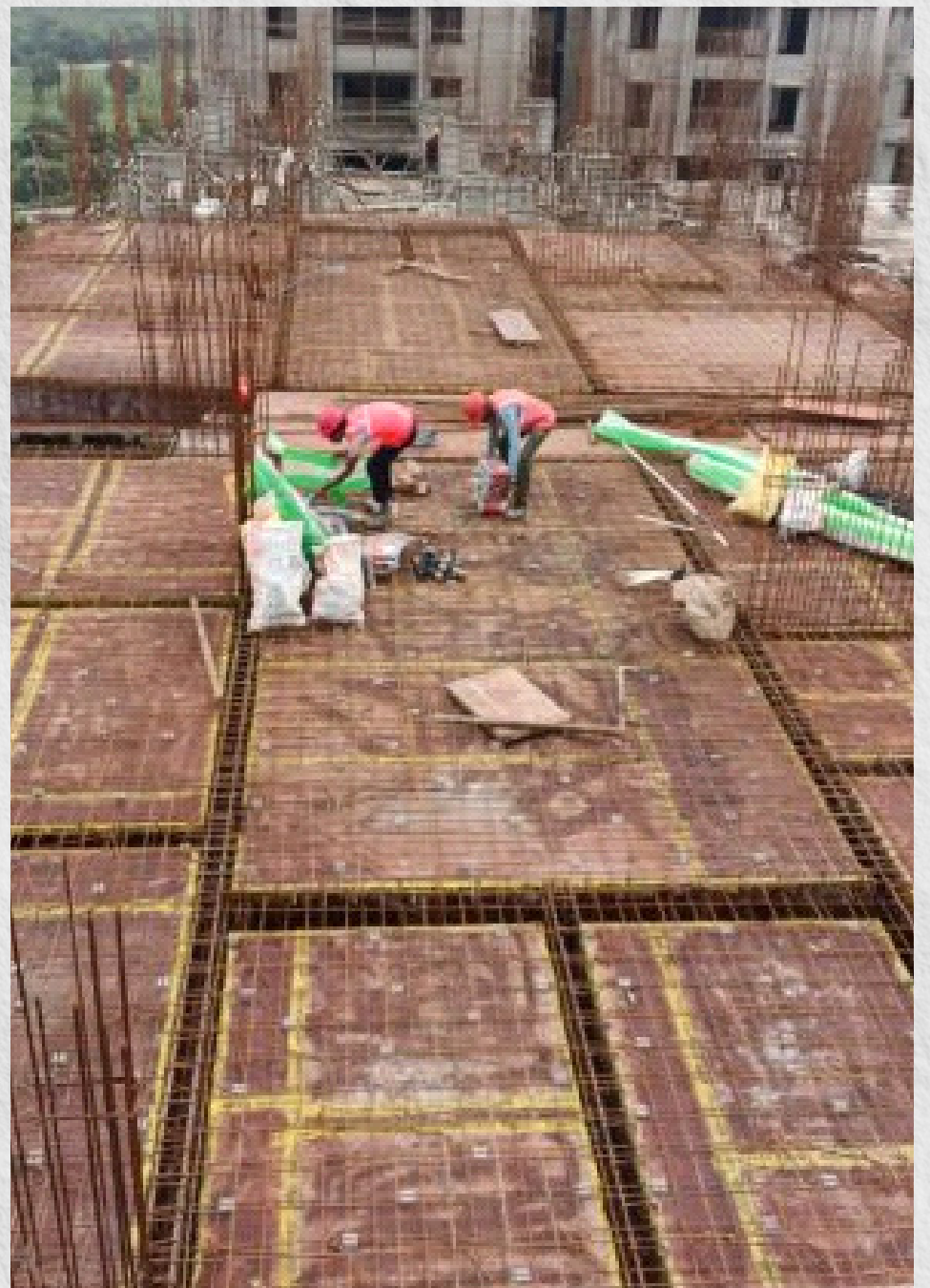
Slab conduits working in progress.
