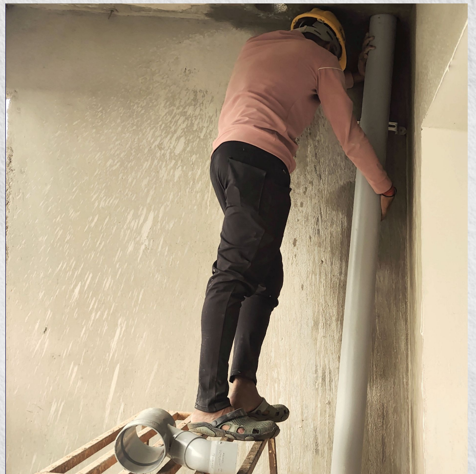
Plumbing lines in the Utility area are installed.
