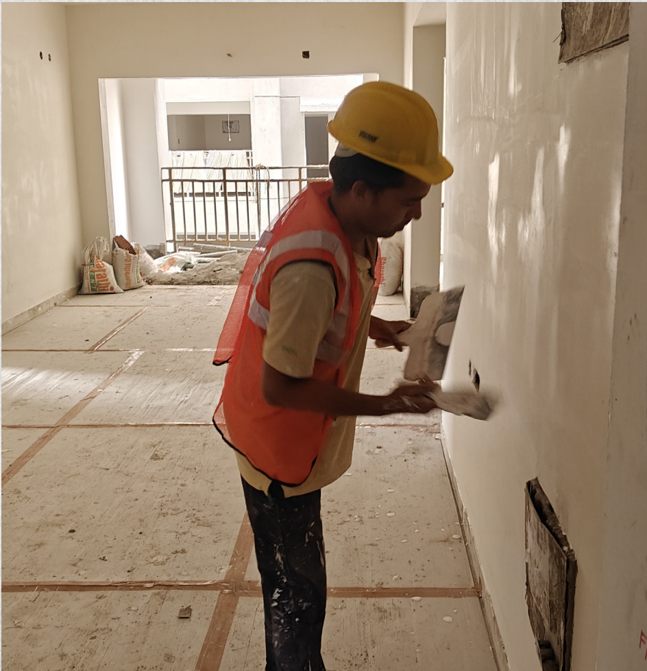
Walls are being marked for electrical switchboard installation.
