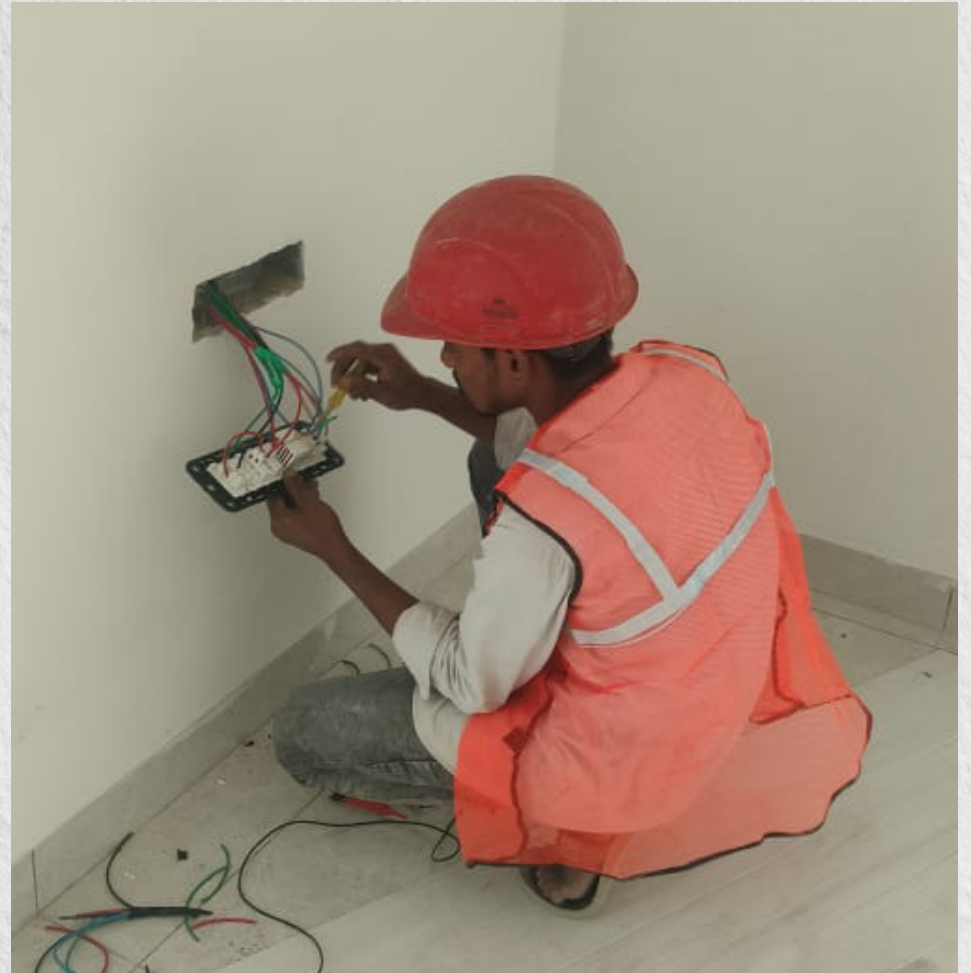
Wiring and Installation of Electrical Switchboards in Progress.
