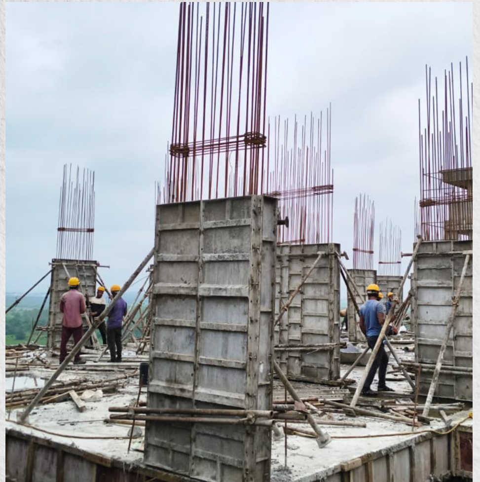
Pour-03 column shuttering work in progress.
