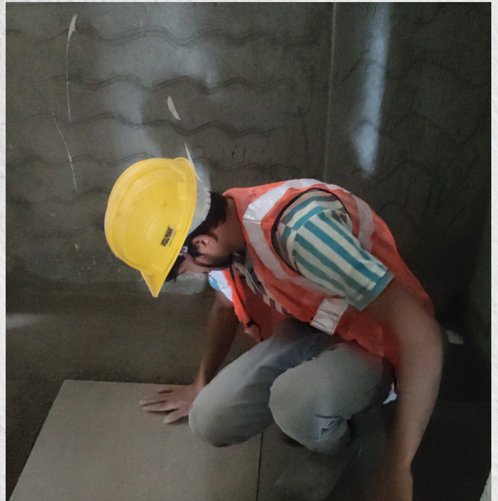
Laying tiles in the toilet.
