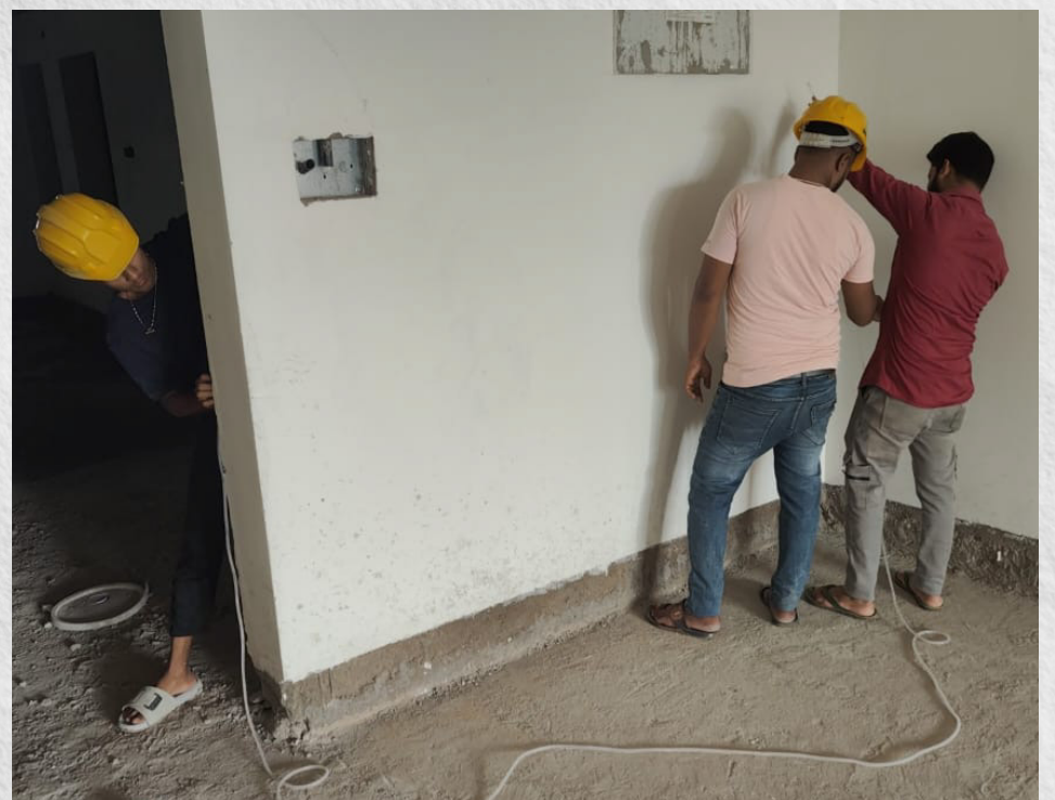
Marking walls for precise tile installation.
