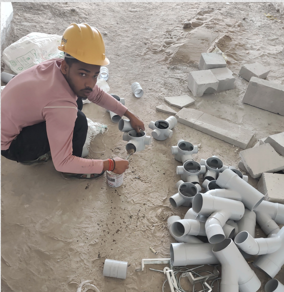
90° elbows and U-bend pipes are being sorted for upcoming plumbing installations
