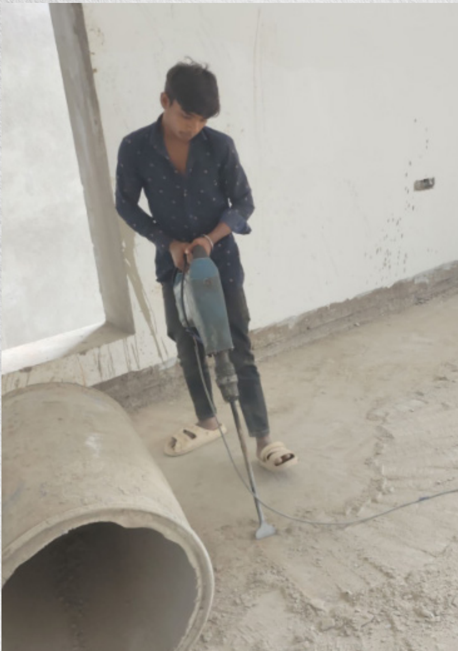
Chipping and cleaning the dry mortar off the floor to lay the floor tiles.
