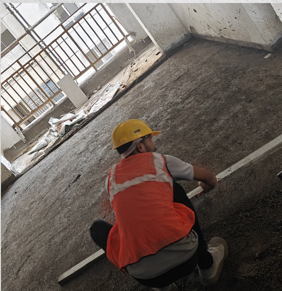
Levelling the surface before laying the floor tiles.
