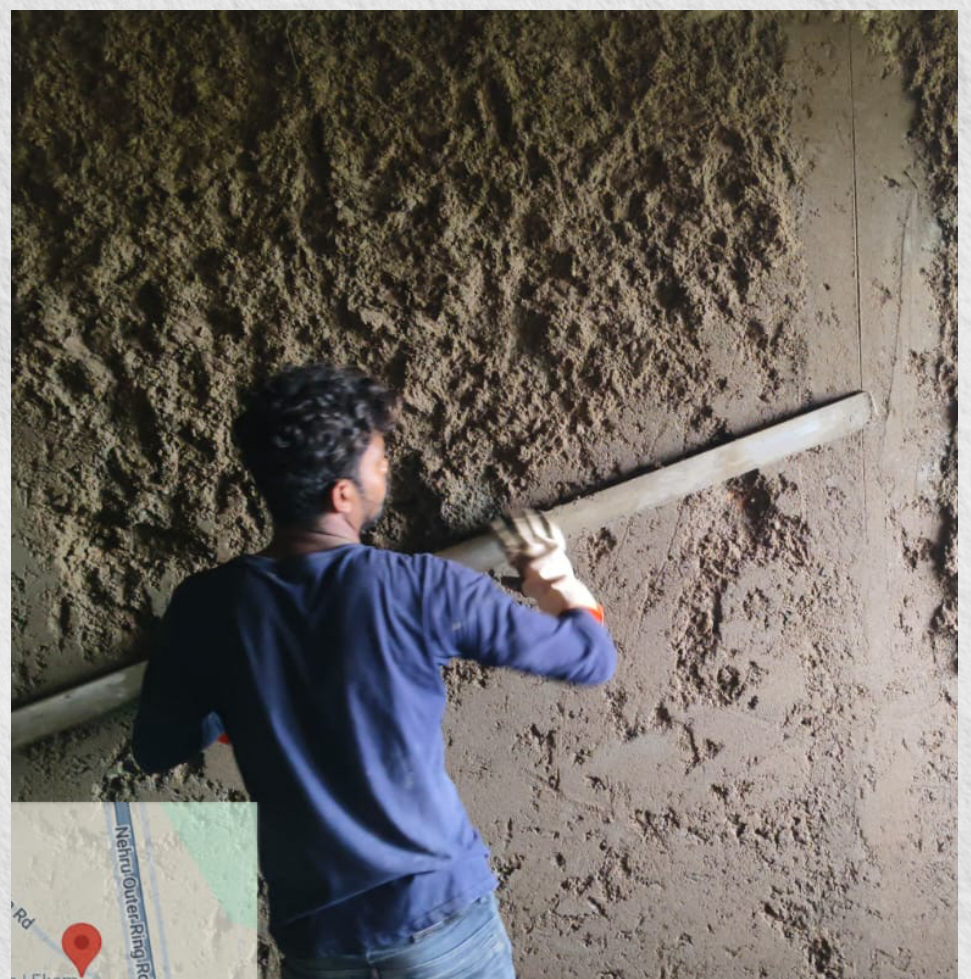
Internal Plastering in 2 different flats in the 4th floor.
