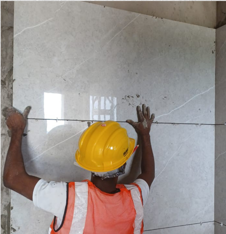
Dado tiles are being fixed on the walls in toilet areas.
