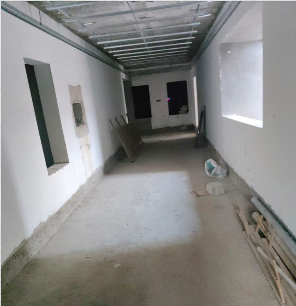
Corridor chipped and cleaned for laying tiles.
