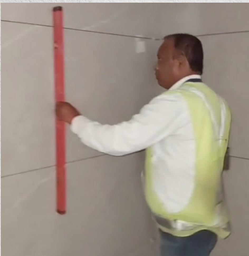
Checking the quality of tile work.
