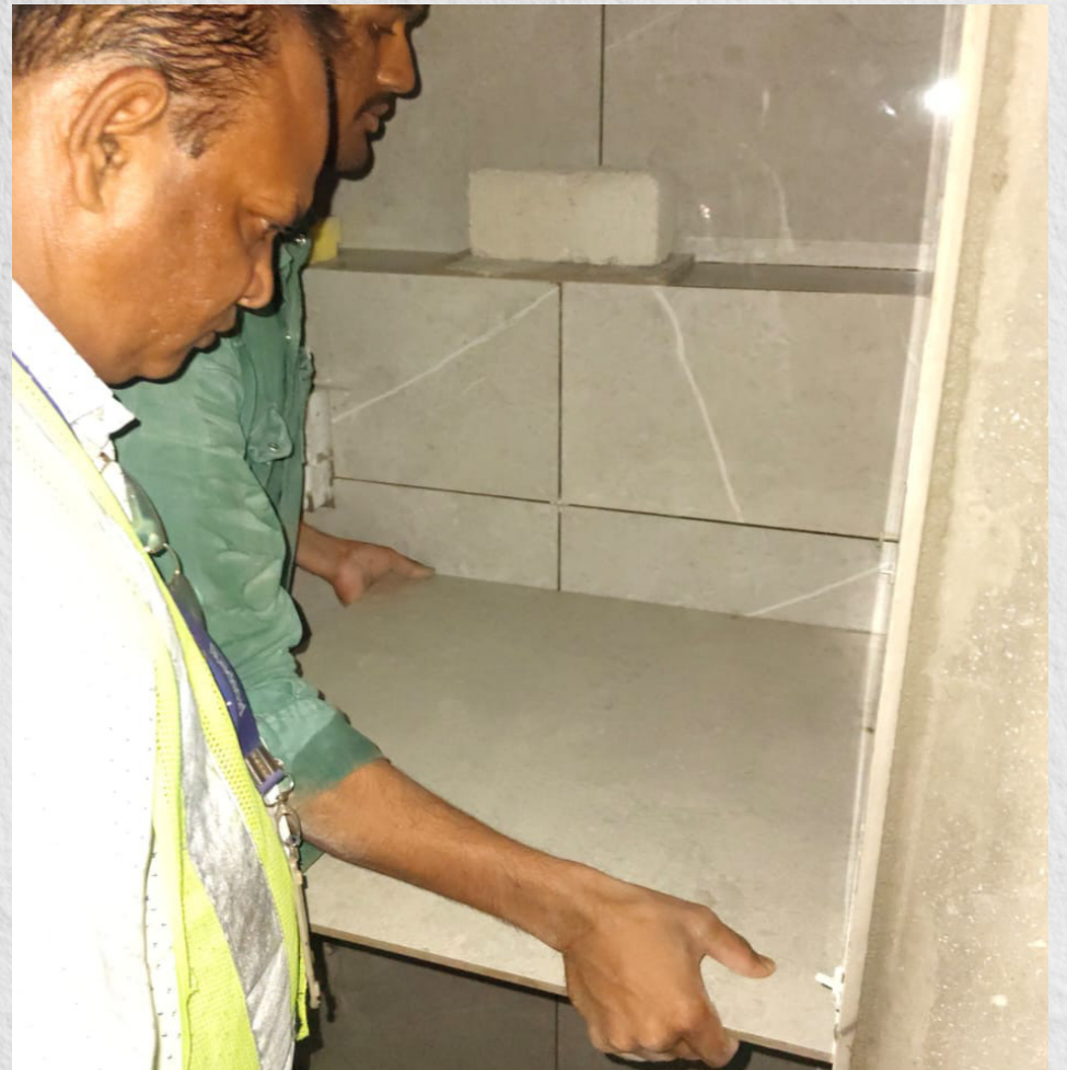
Inspection of tile laying is being done by our Senior Site Coordinator.
