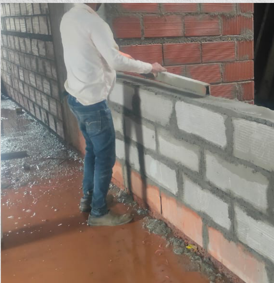
7th Floor corridor area block work in progress.
