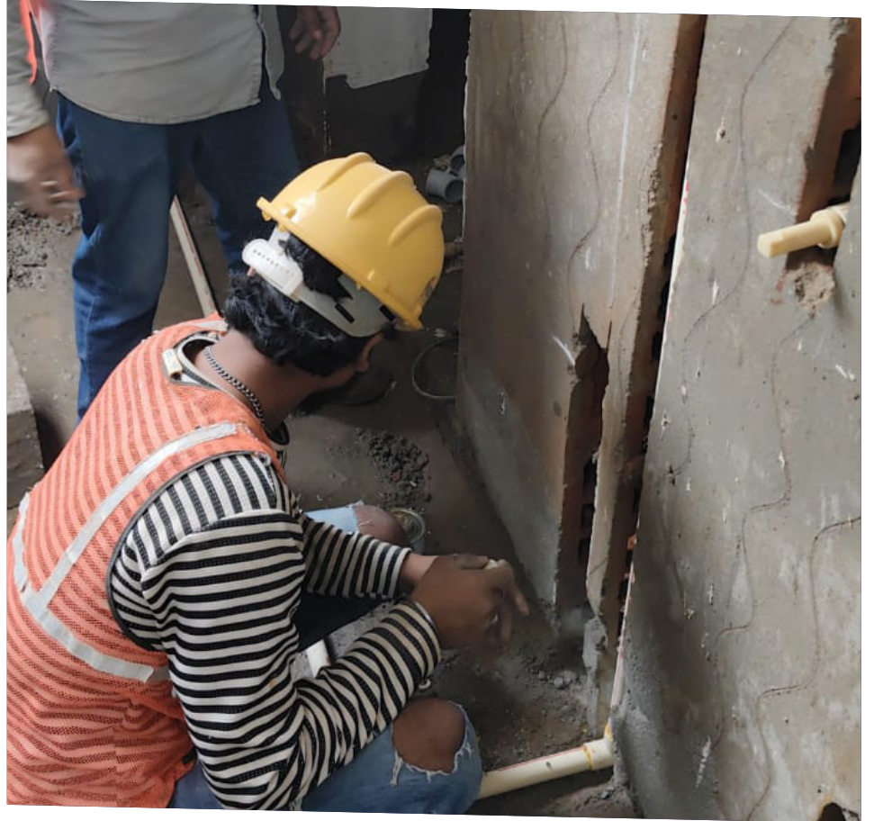
Plumbing work in progress in the Utility area.
