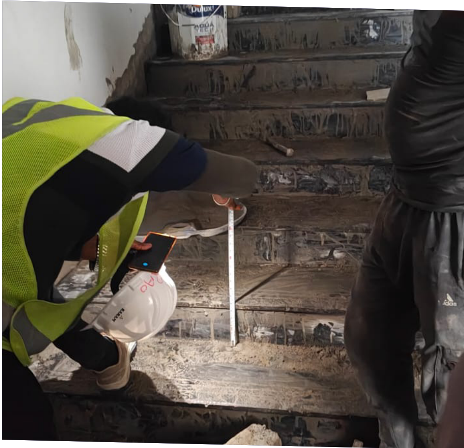
Granite tiling work is in progress for the Tower 2 staircase.
