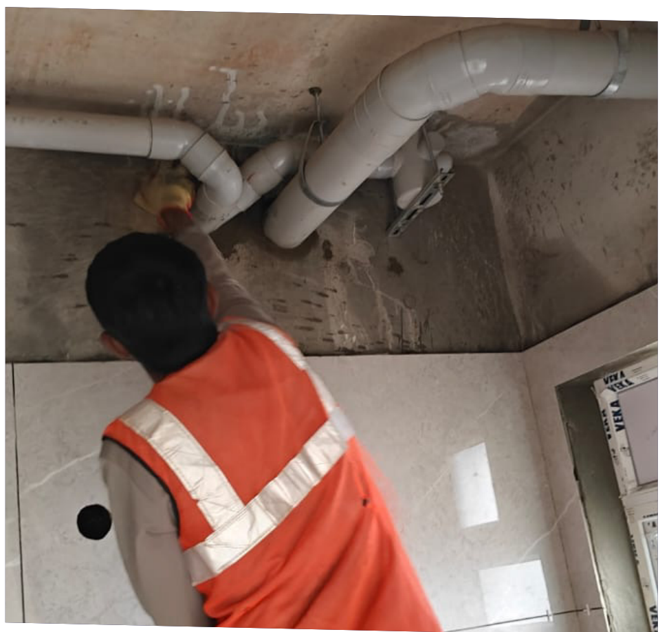
10 th floor – Installation and gp2 packing of plumbing lines in progress.
