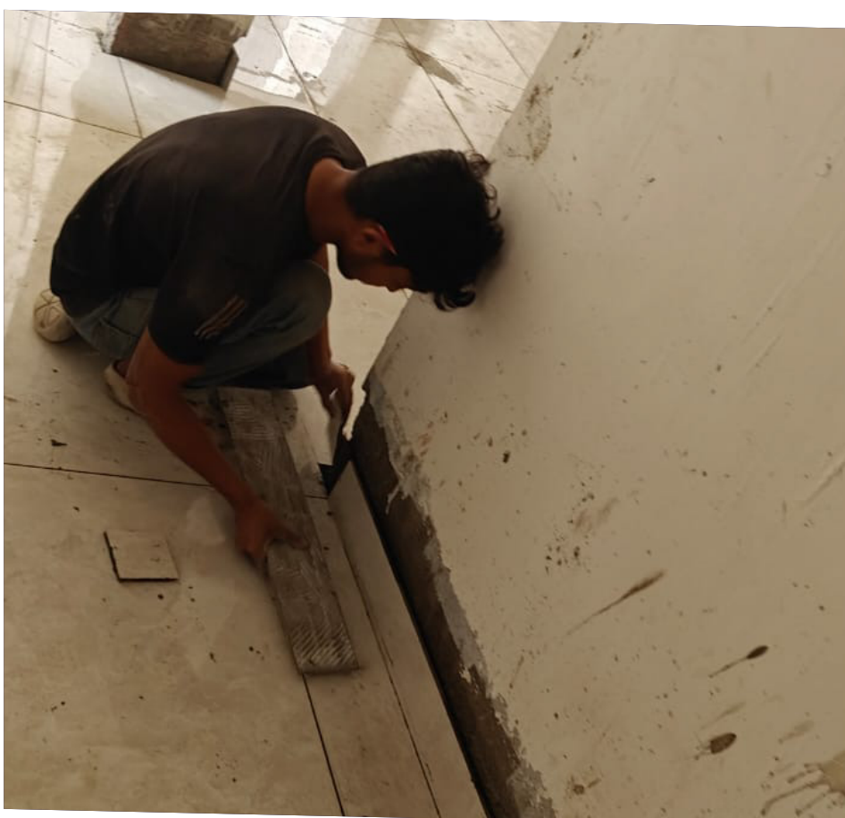
Skirting tile works are in progress across the 8th-floor flats.
