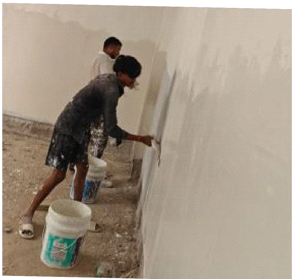
Wall putty works are in progress in the 12th-floor flats.
