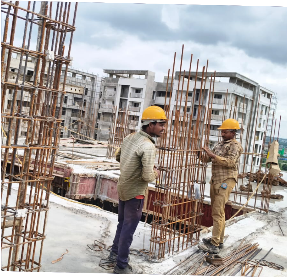
Reinforcements columns for 11th floor slab works.
