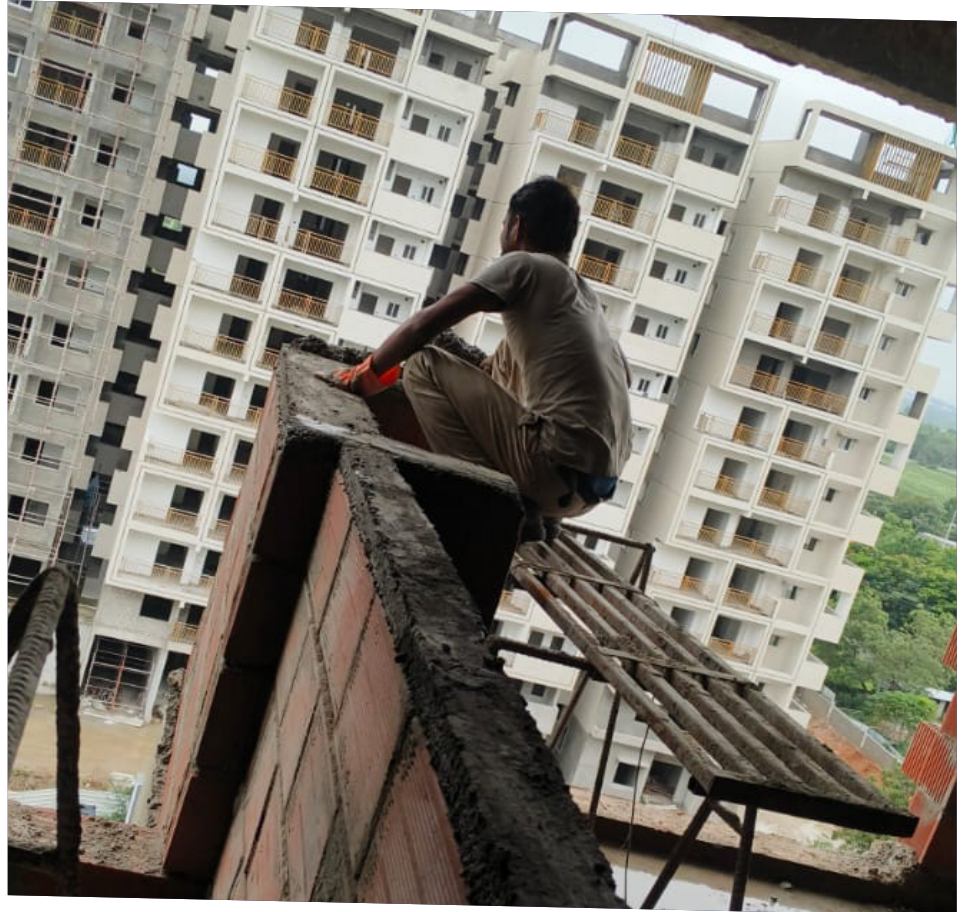
Sill level brick work in progress on the 6th floor.
