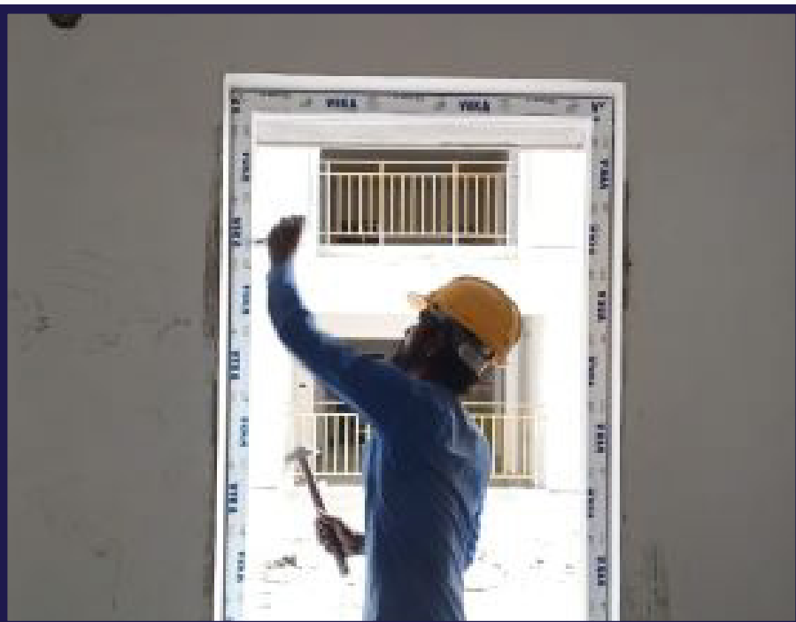
Fixing of UPVC window in progress.
