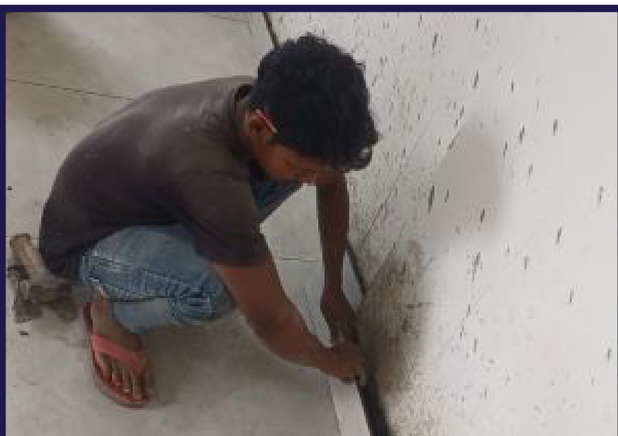
Skirting work in progress in 6 th series.
