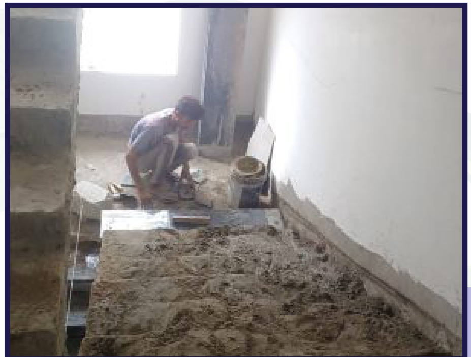
Laying of granite slabs on staircase no: 2 in work in progress.
