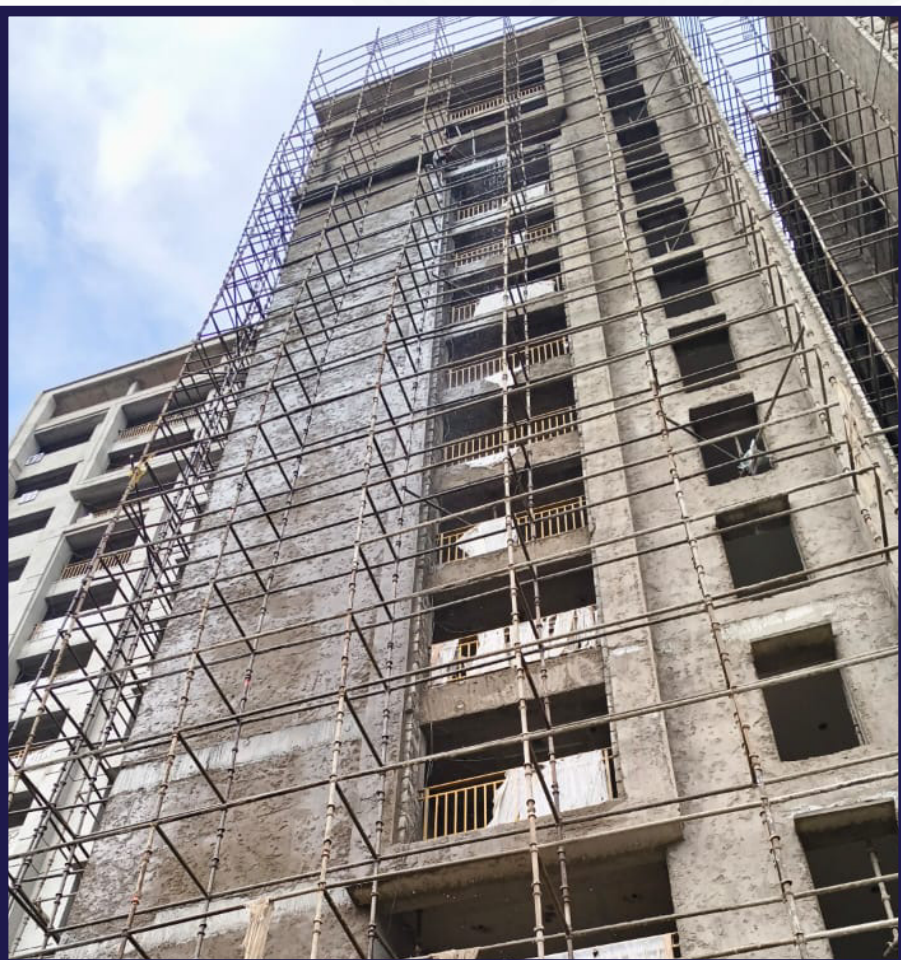
Curing of external Plastering on the East side of Tower -1.
