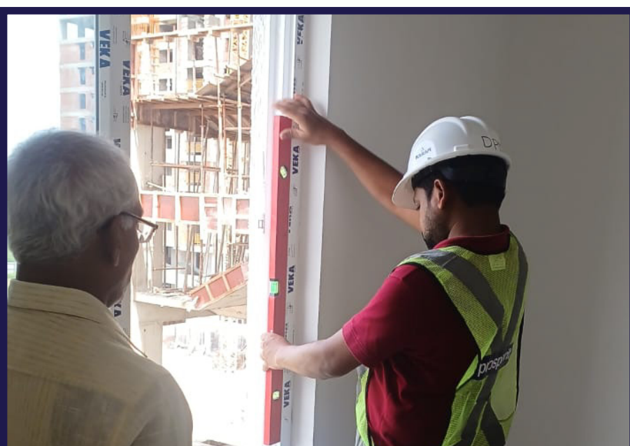
Checking the alignment of Window frame is in progress.
