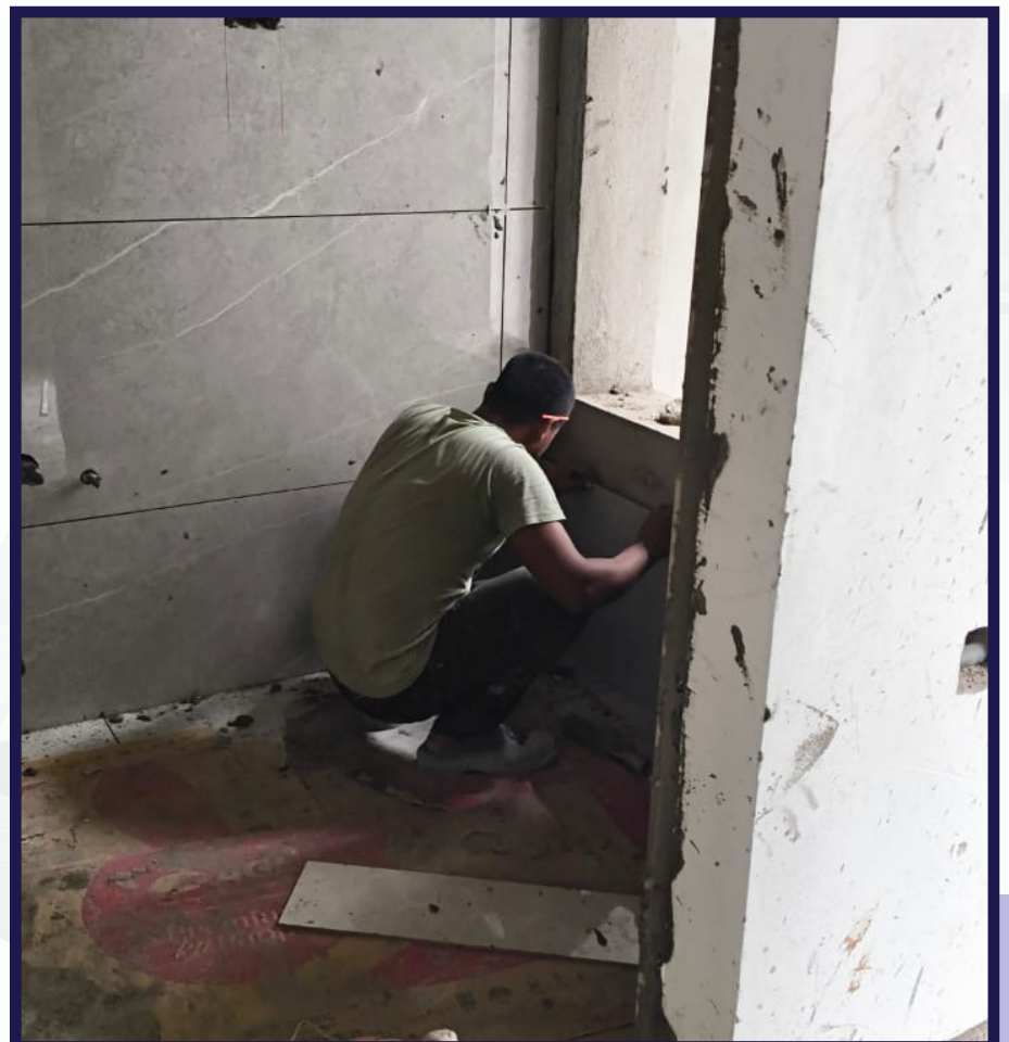
Laying of tiles in the toilets is going on.
