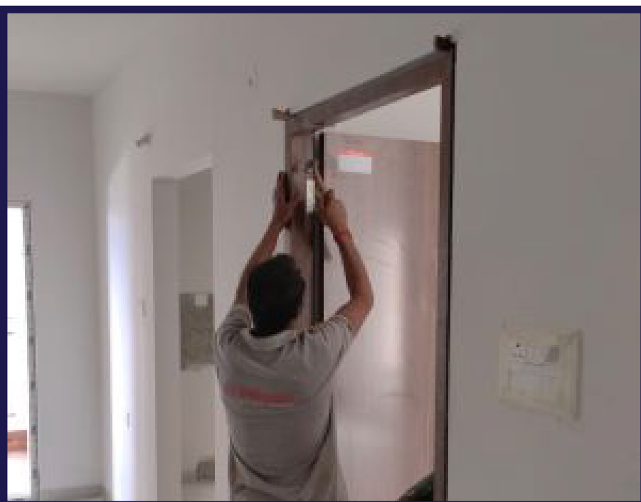
Internal door frames are being installed and fixed.
