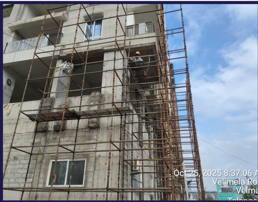
External pin block work on the north Side is in progress.
