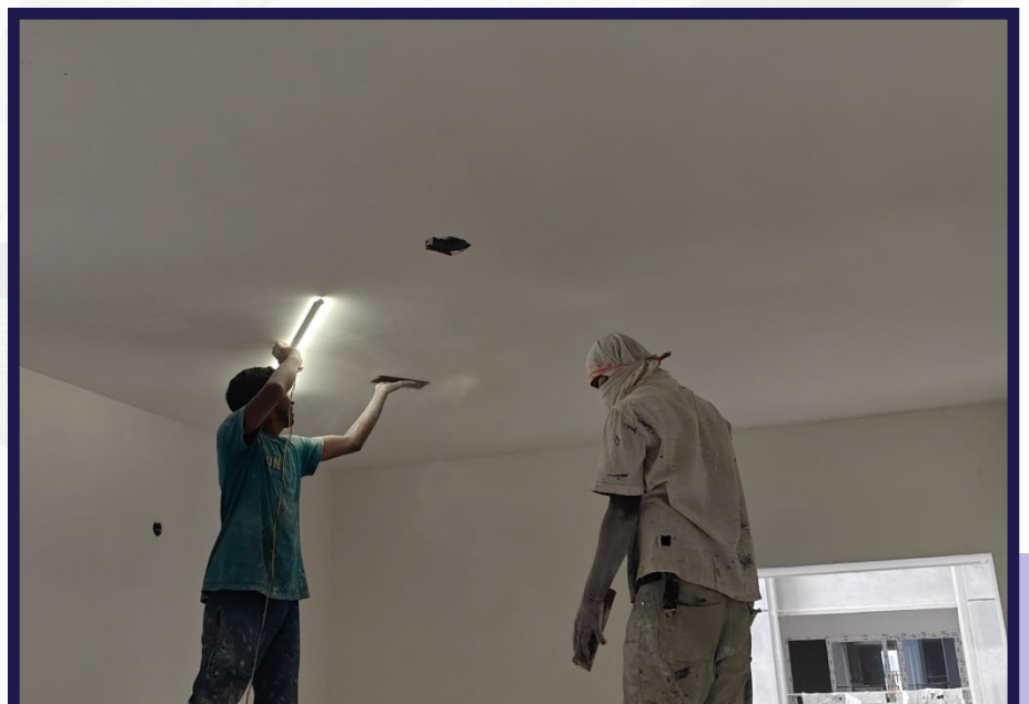
Sanding the putty wall for smooth finish is in progress.
