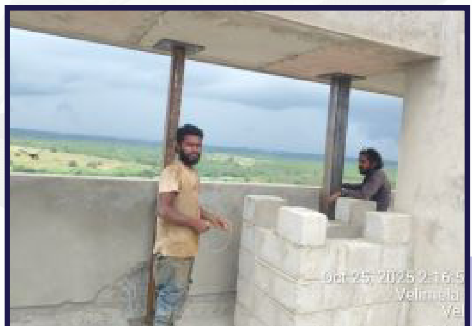
Construction of MS channel along the Pergola is in progress.
