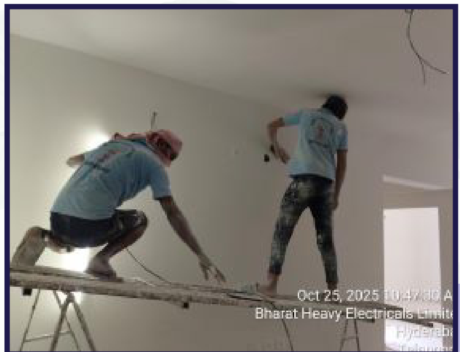
Sanding of the putty on the walls is in progress.
