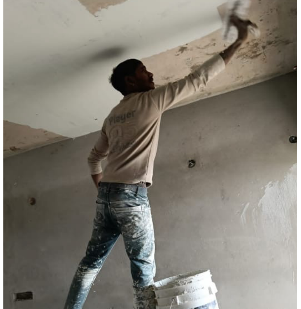
Application of coarse putty on the ceilings 7th floor flats are in progress.
