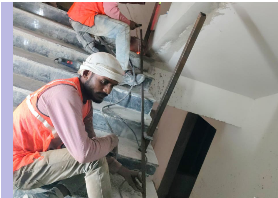
Welding works on railing for Staircase – 1 is in progress.
