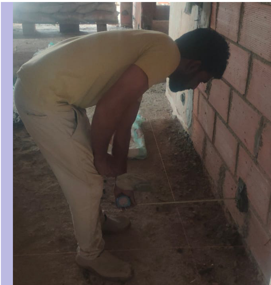
Fixing of Bull marks is in progress in 8th floor.
