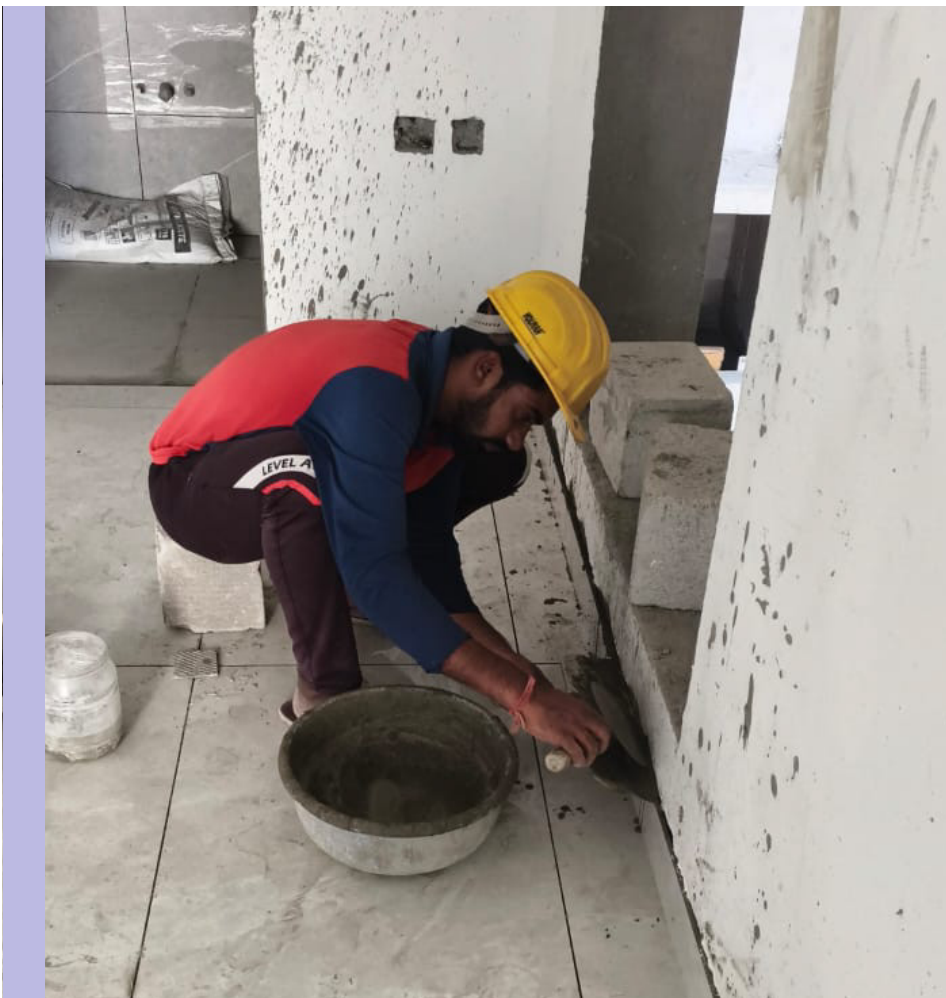
Skirting packing of tiles is in progress.
