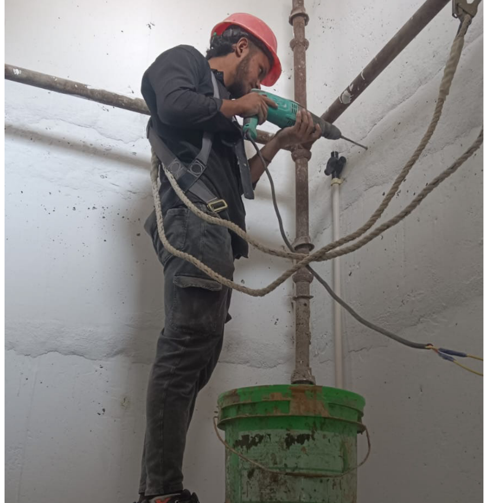
Installation of lift shaft lights, 4m metal boxes, and 25 mm PVC pipes are in progress.
