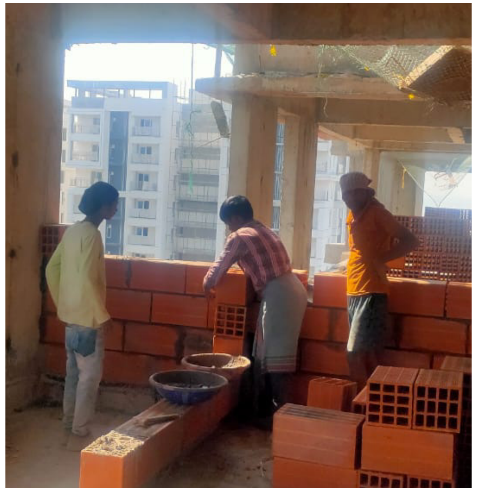
Sill Level block work is in progress in 10th floor flat.
