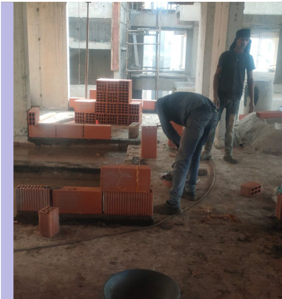
Layout marking in progress in the 11th floor.
