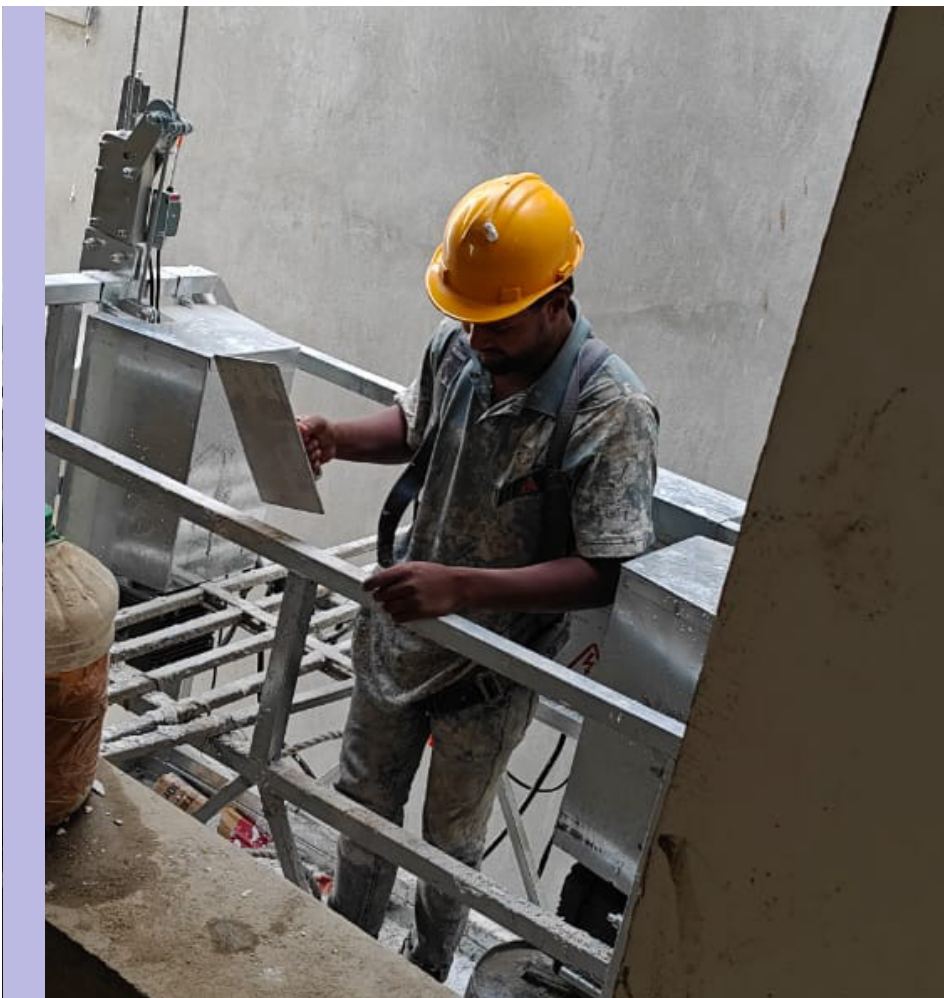
External Texture Application in the OTS Area is in Progress.
