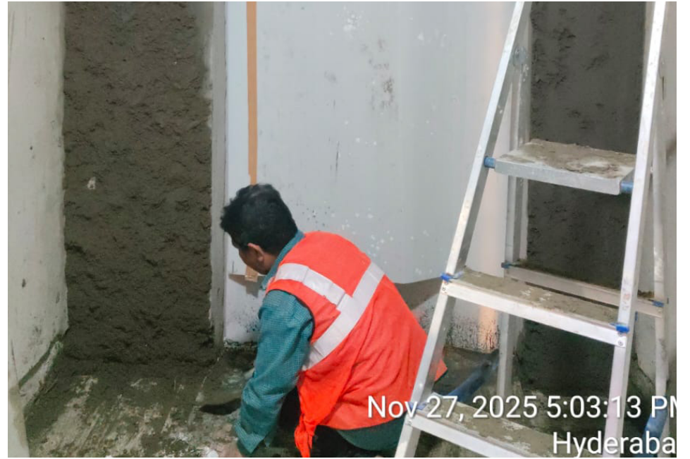
Plastering work on external pin is in progress.
