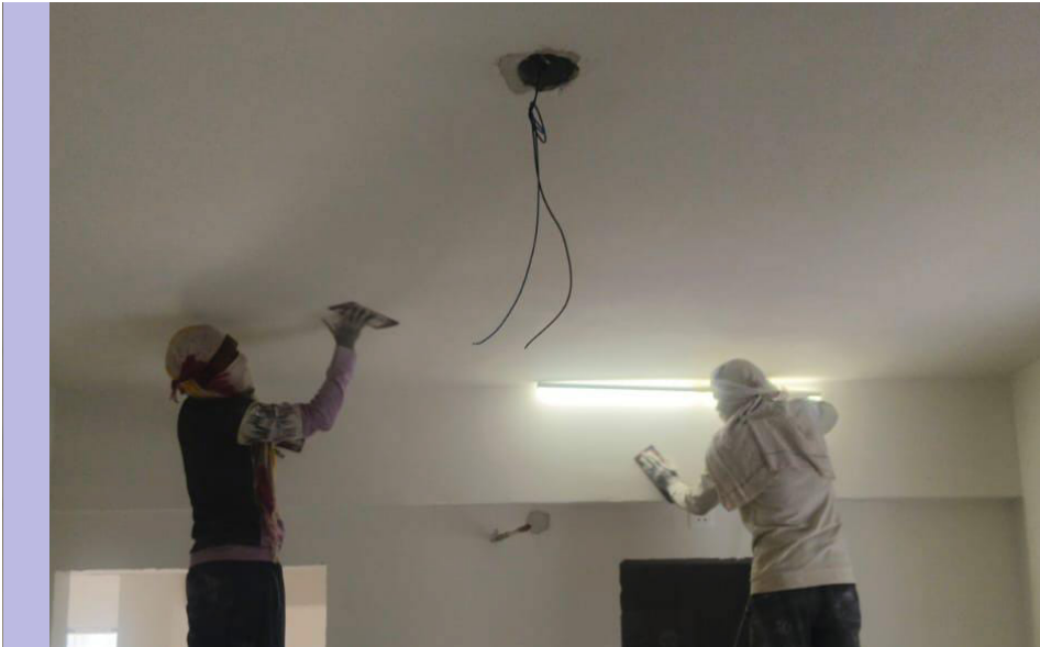
Sandpapering Work in the 11th flats is in Progress.
