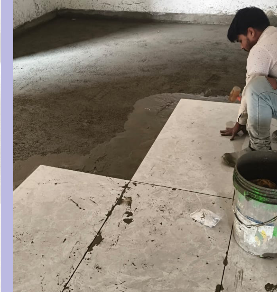
Internal tile laying work is in progress.
