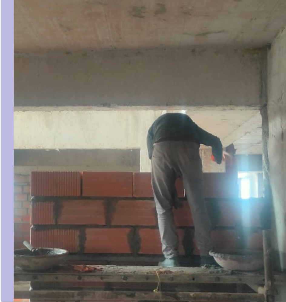
10th Floor Above-Sill-Level Block Masonry is in progress.
