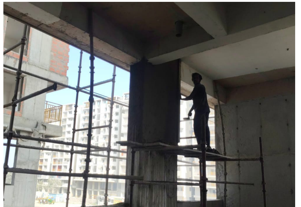
Plastering work on external pin is in progress.
