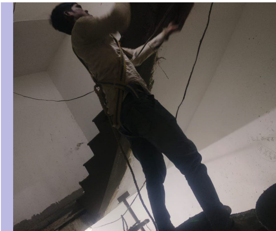
Granite side packing and plastering work is in progress on staircase - 1.
