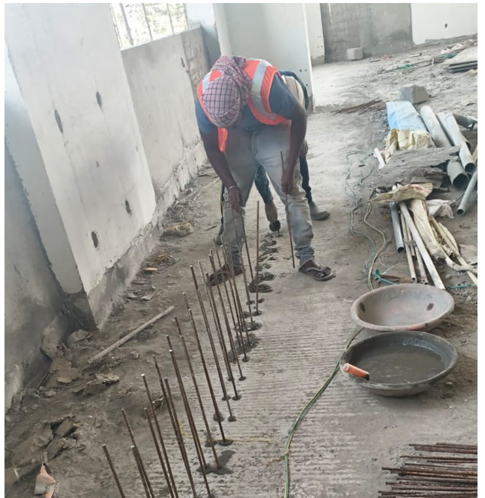
Sleeper wall steel grouting in the podium floor landscaping zone is currently underway.
