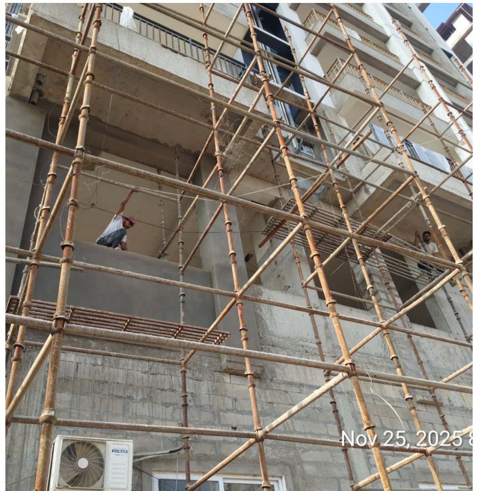
North side external pin plastering work in progress.
