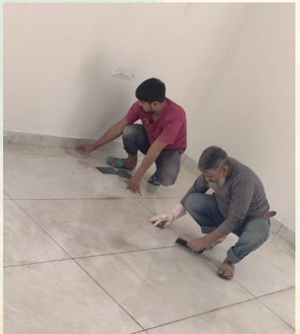
Preparing the tile floor for grouting in the 4 series flats.
