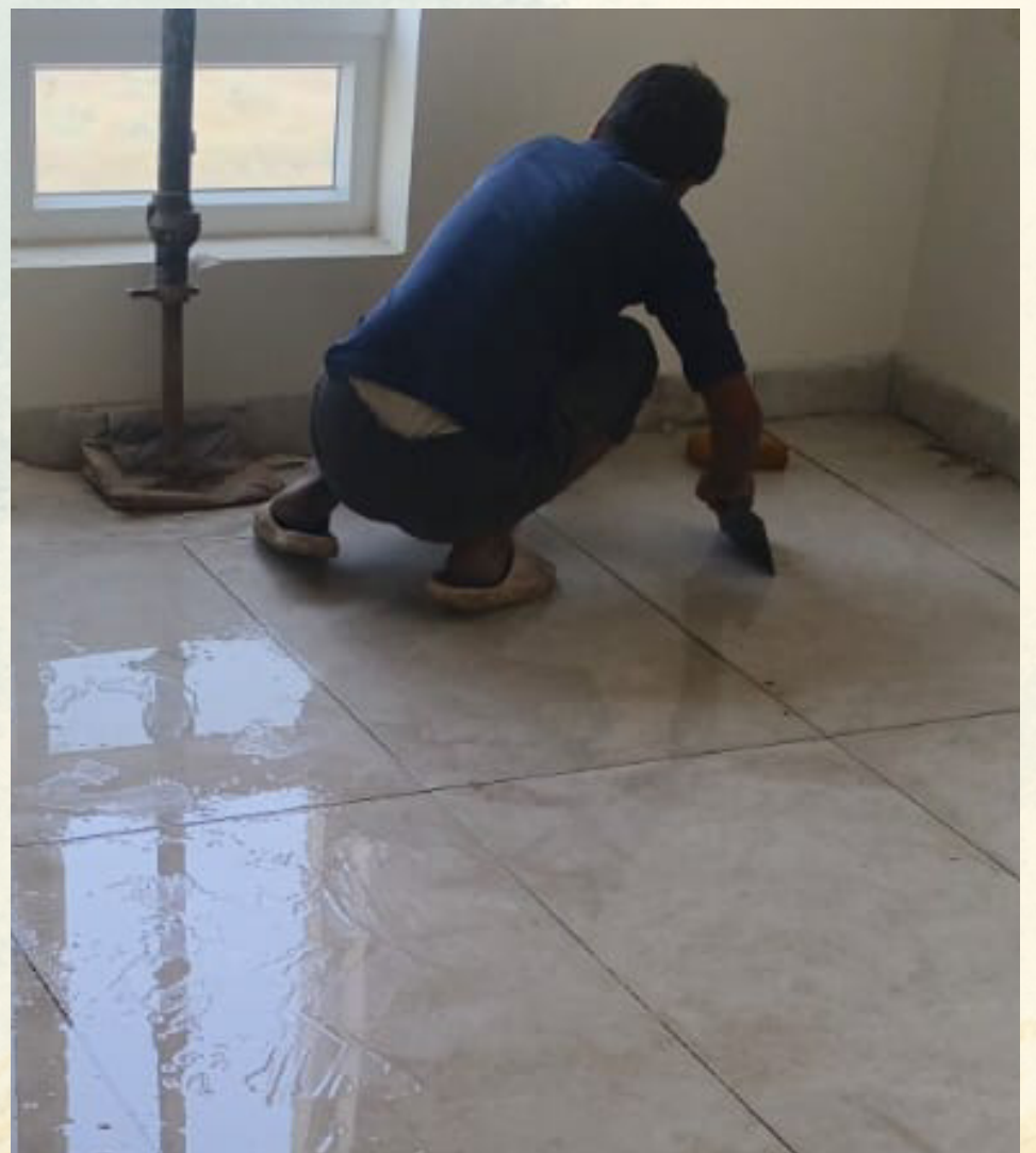
Preparing the tile floor for grouting purpose.
