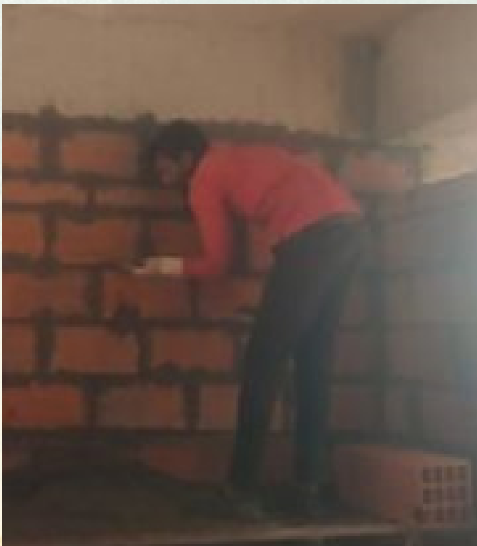
Above-sill blockwork is currently in progress in the 12th floor.
