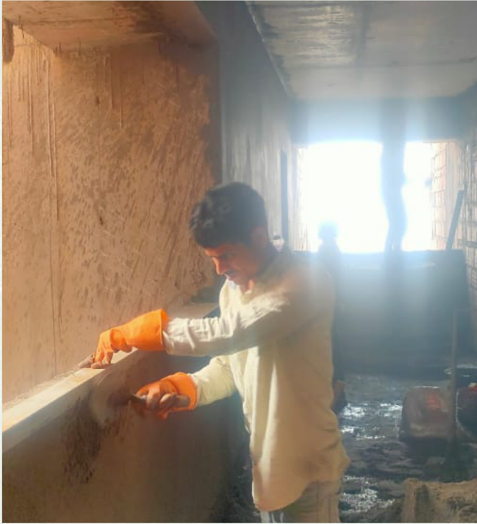
Plastering works are underway in the 8th-floor corridor.
