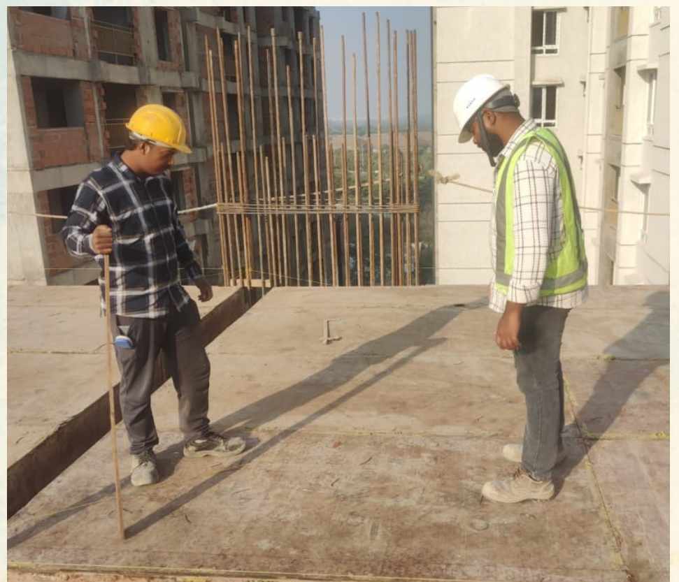
Clubhouse fifth-floor slab-level shuttering quality checks are currently in progress.
