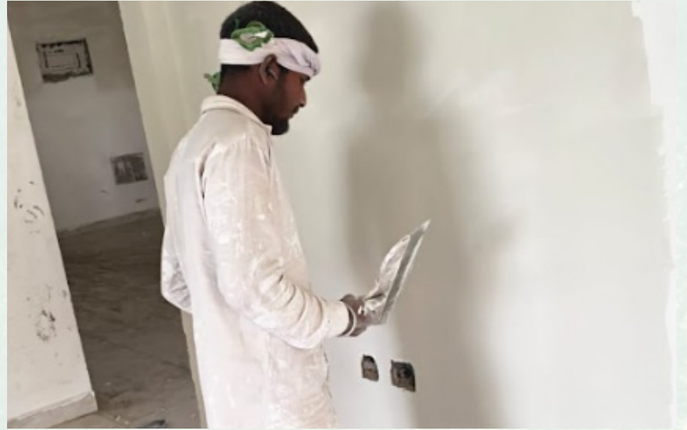
Hollow sound checking work is in progress in a Flat on the 11th floor.
