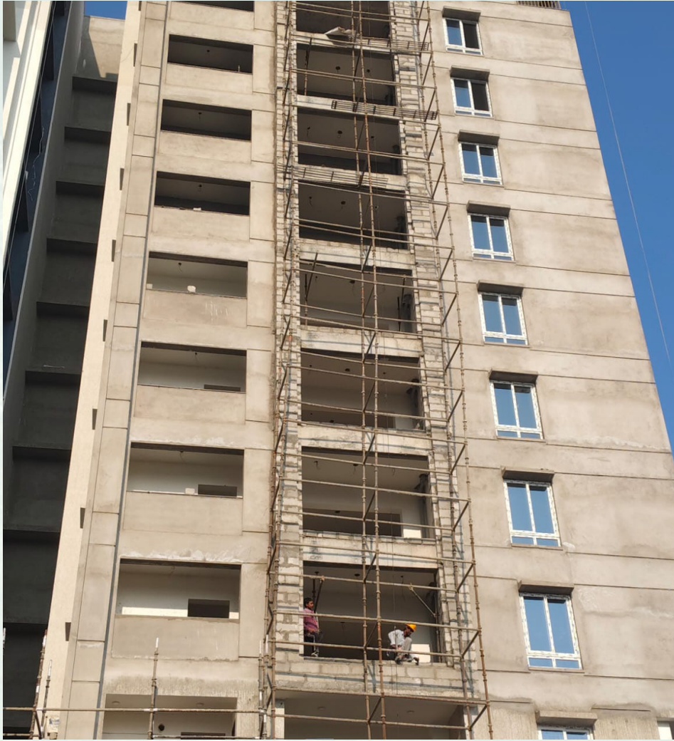
External bull marking work for pin plastering of the 1st series is in progress.
