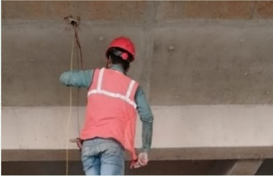
Expansion joint TPE tape fixing work is in progress at the podium level.
