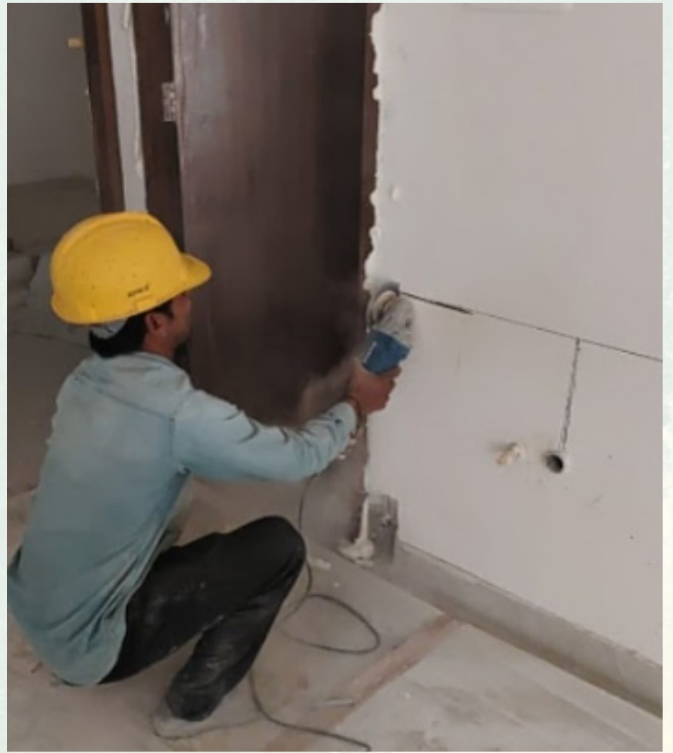
Chasing work in progress for fixing the dining area sink bracket.
