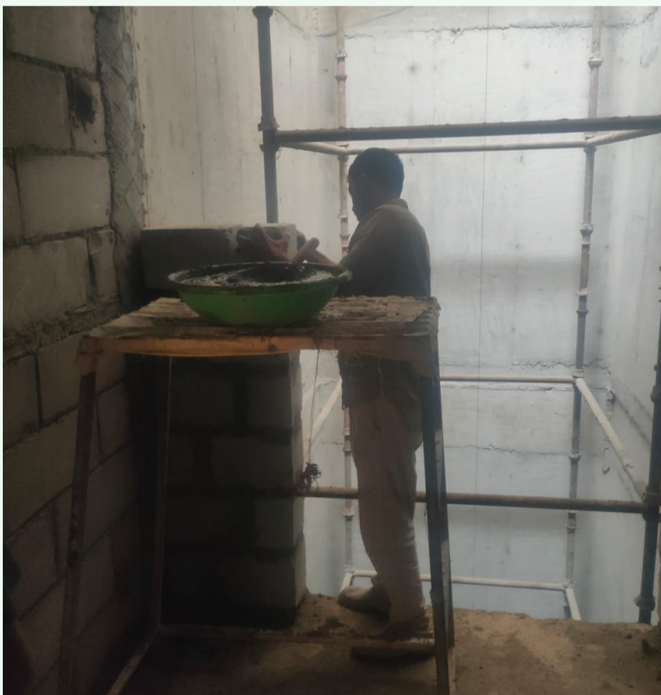
External plastering of the service elevator shaft.
