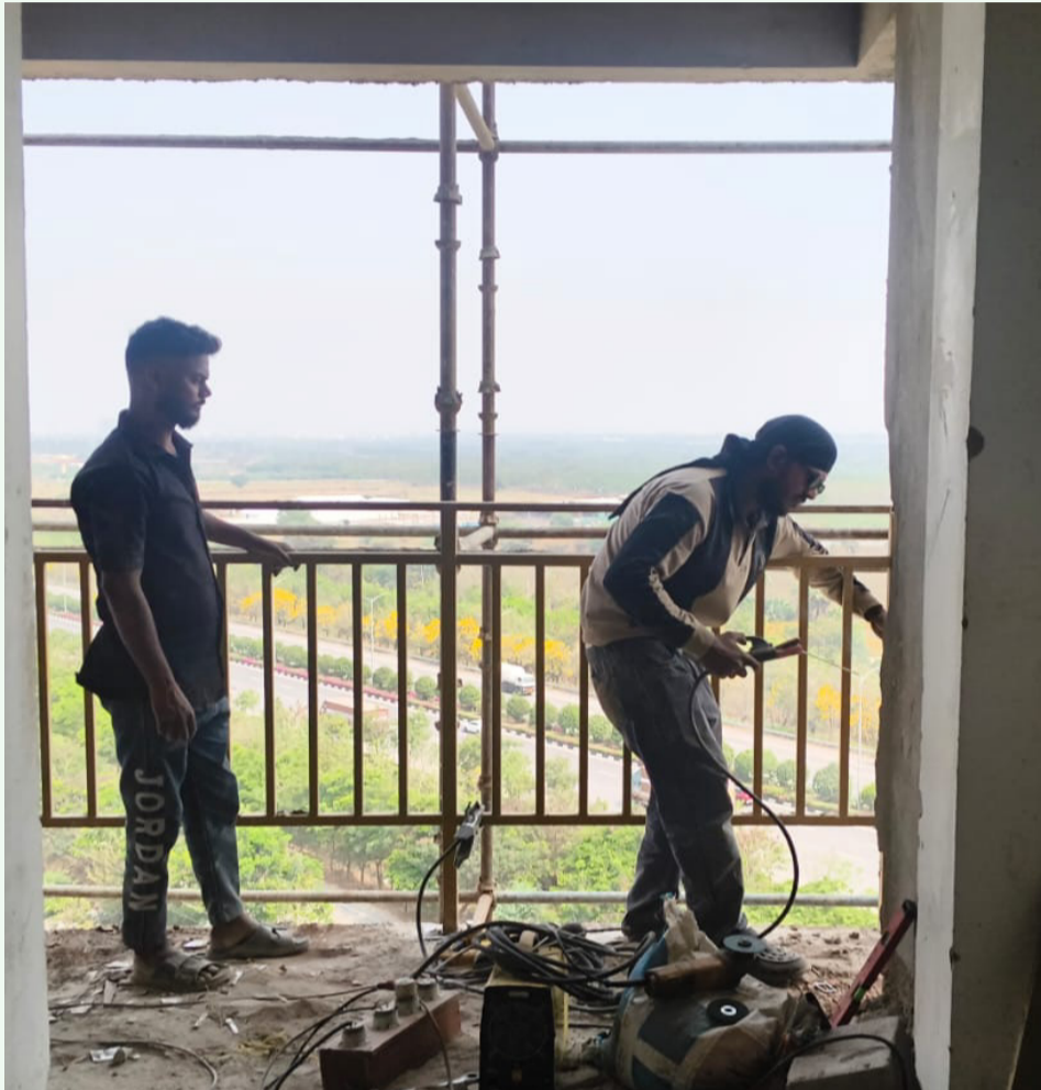
Fixing of Railing works are in progress.
