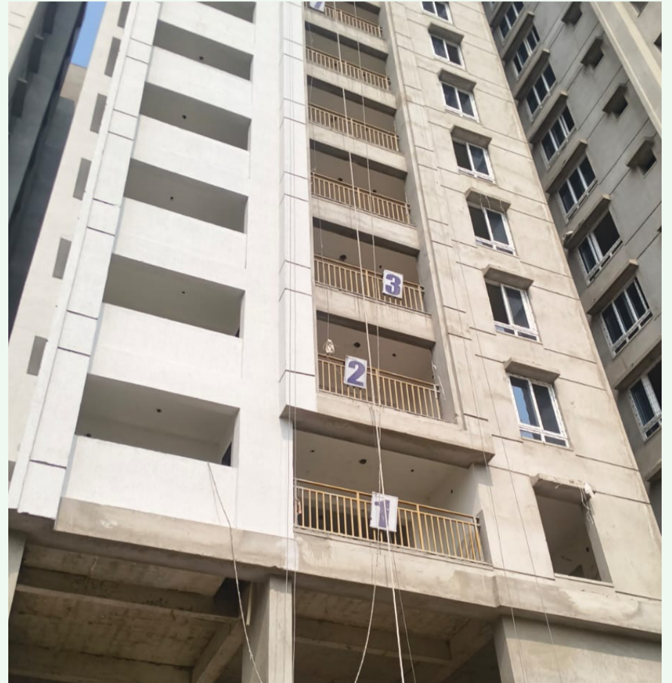
External-side granite bottom GP2 packing works are currently in progress.
