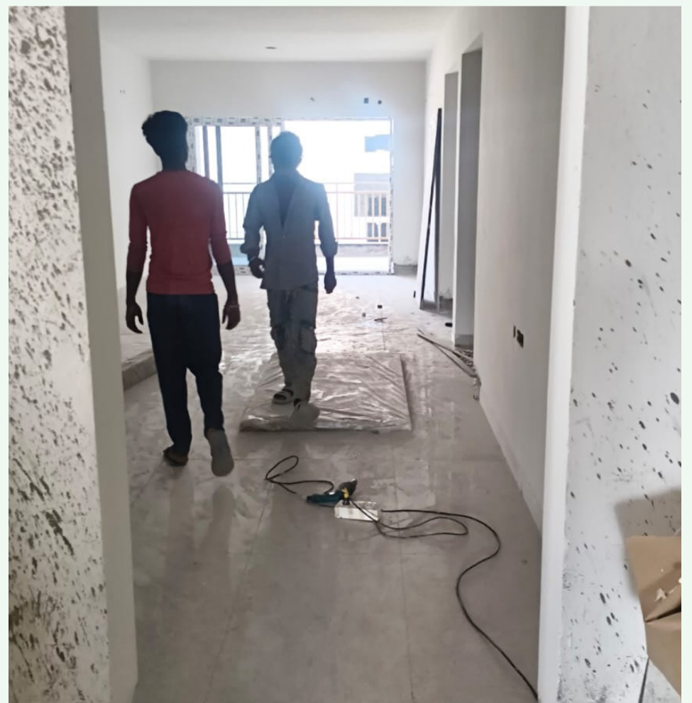
Installation of main doors is currently underway in no. 2 series flats.
