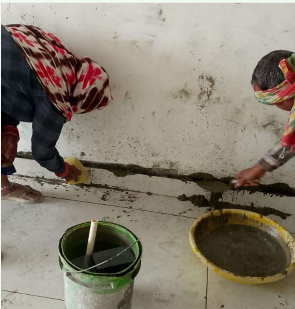
Rectification of skirting works is being undertaken following inspection.
