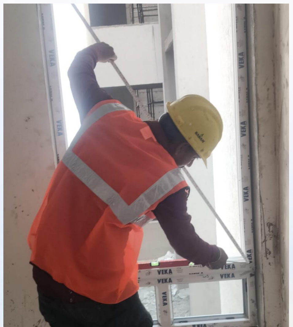
UPVC window fixing work for the 7 series is currently in progress.
