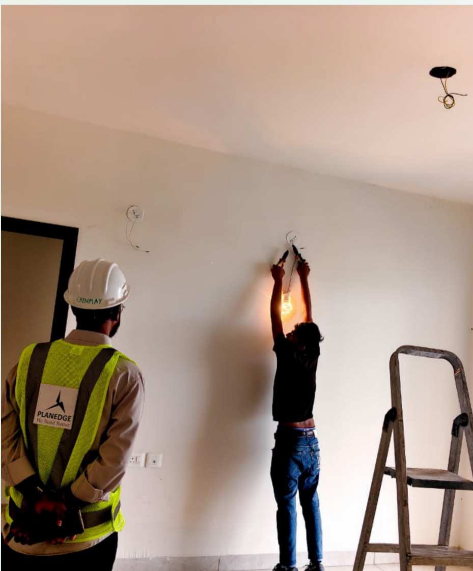
MEP points are being checked by 3rd party inspection team.
