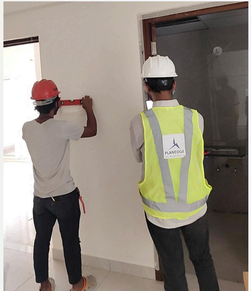
Third-party checking and snagging of electrical points in progress.
