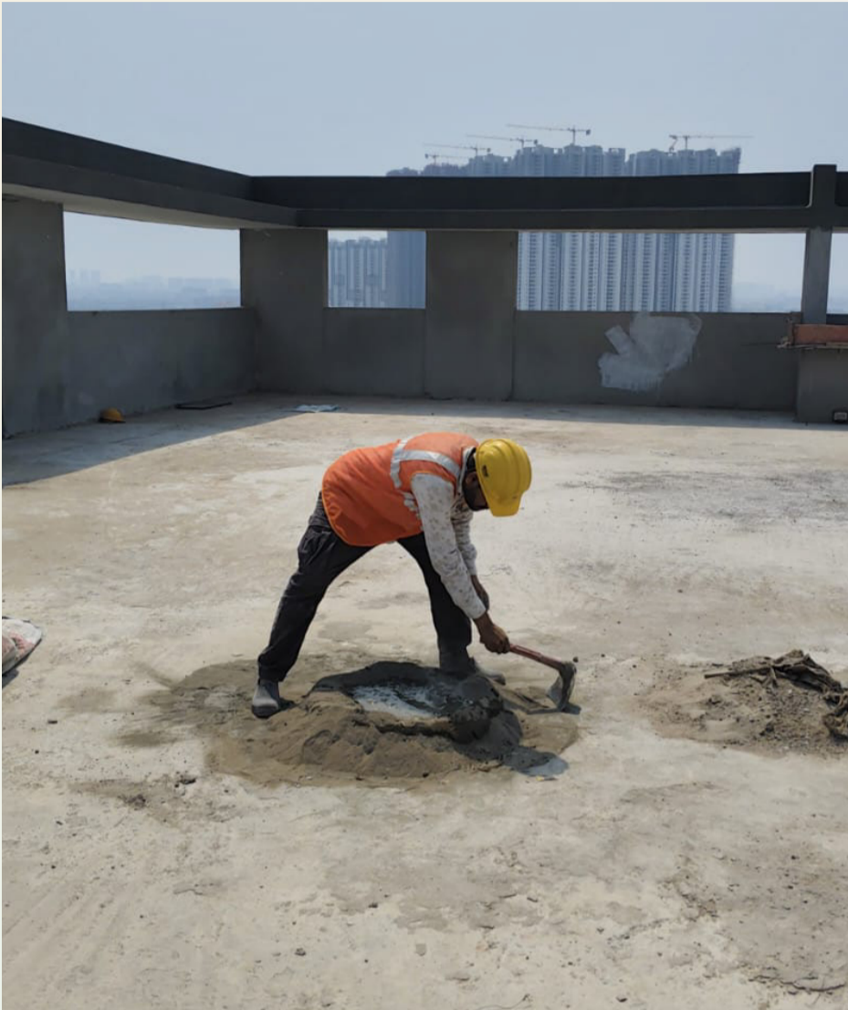
Roof Terrace : Coving works in progress for water pond testing.
