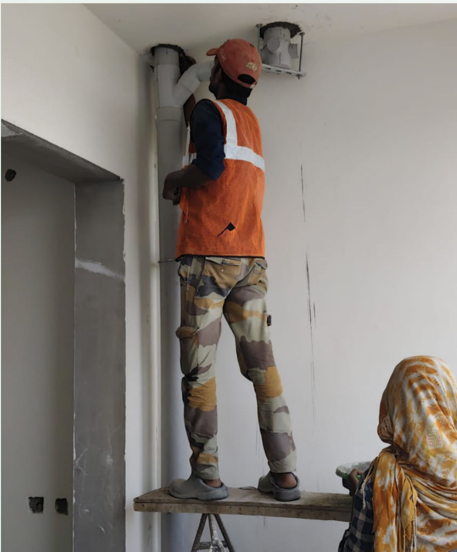
Bore packing work on the 12th floor is currently in progress.
