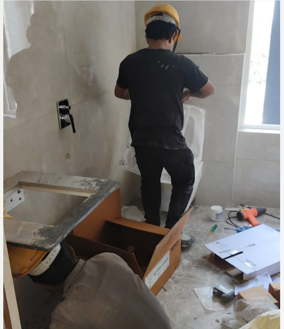
First-floor CP fittings and sanitary works are in progress.
