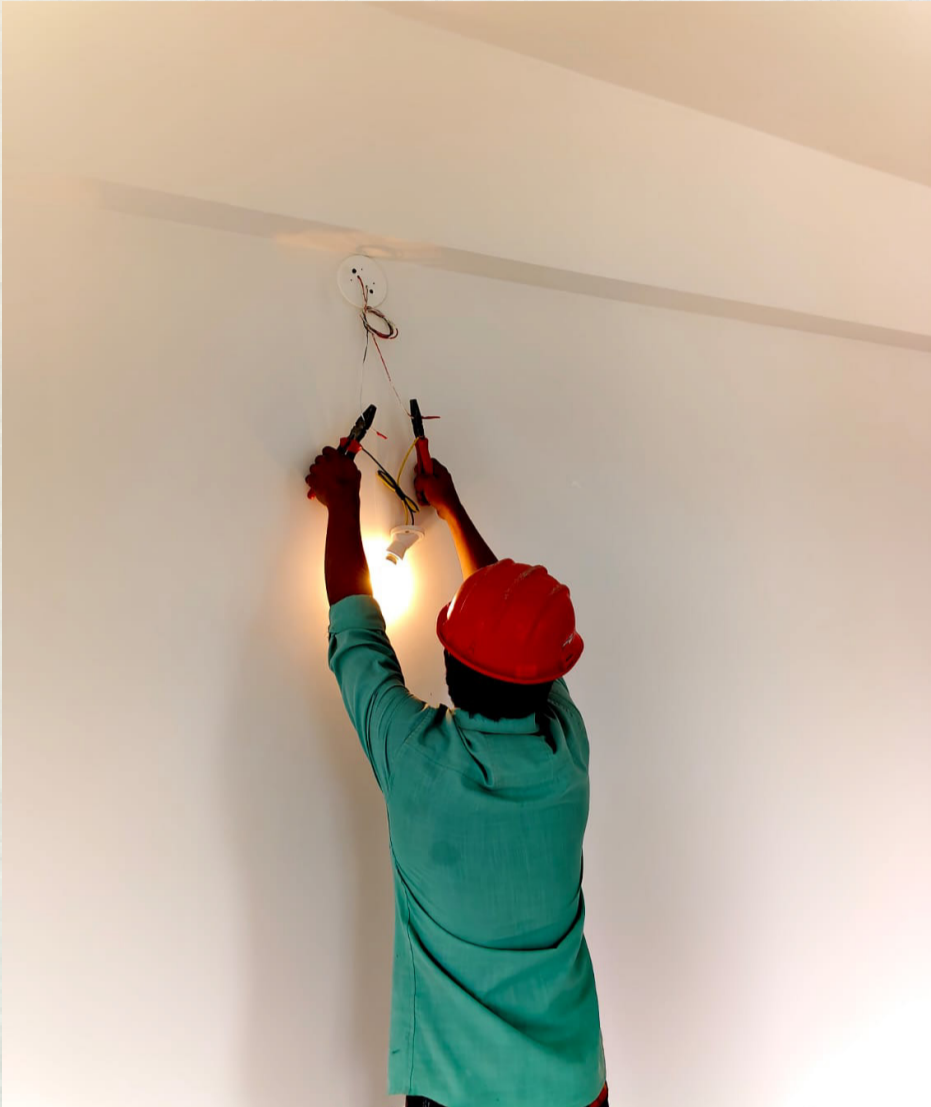
MEP finishing works' inspections are ongoing in selected flats.
