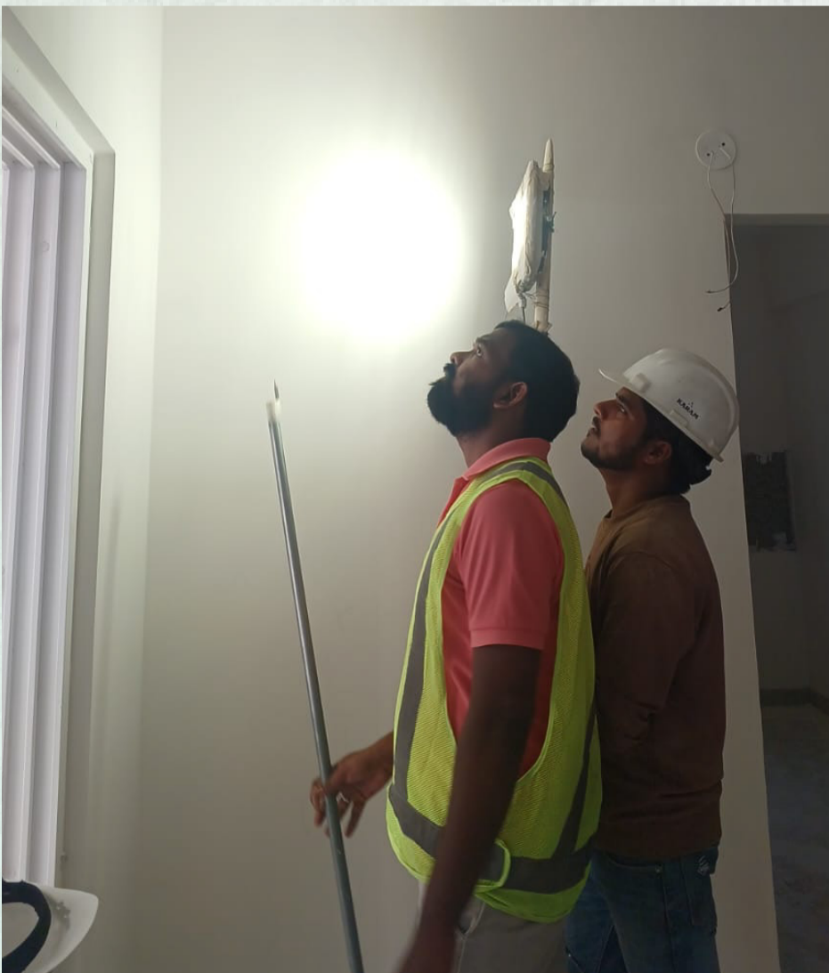
Quality checks of the second coat painting are being carried out.
