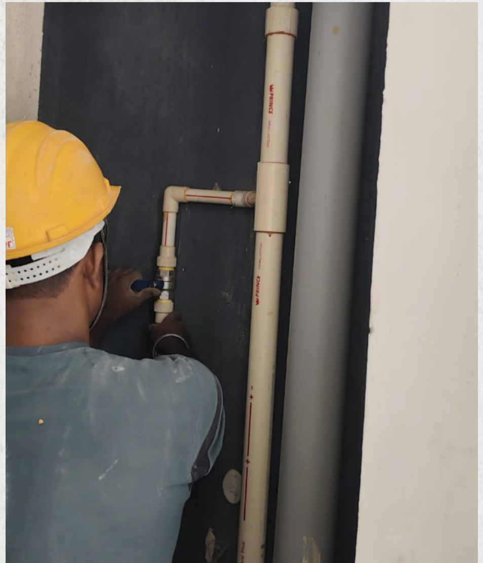
Ball valve and water meter connection works are in progress.
