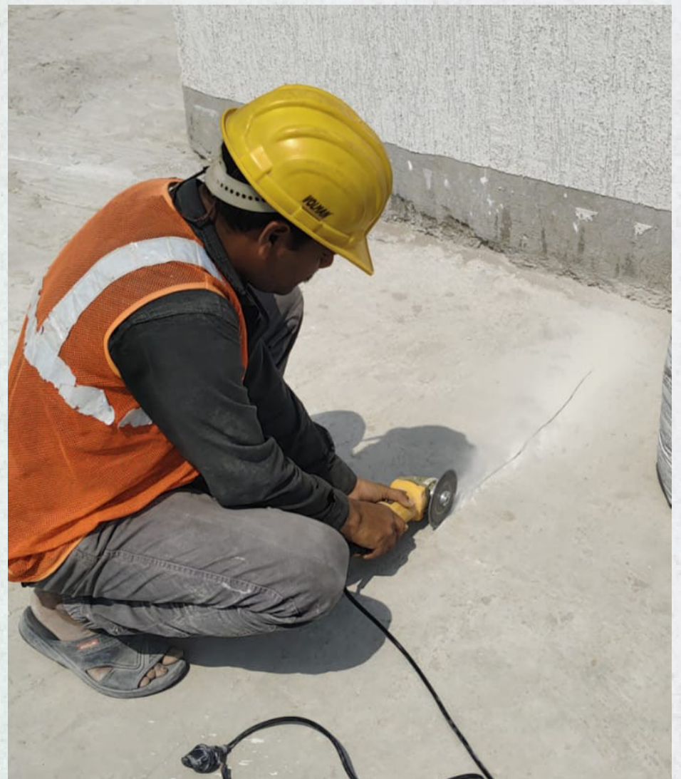
Crack treatment works are in progress on the Tower-3 roof area.
