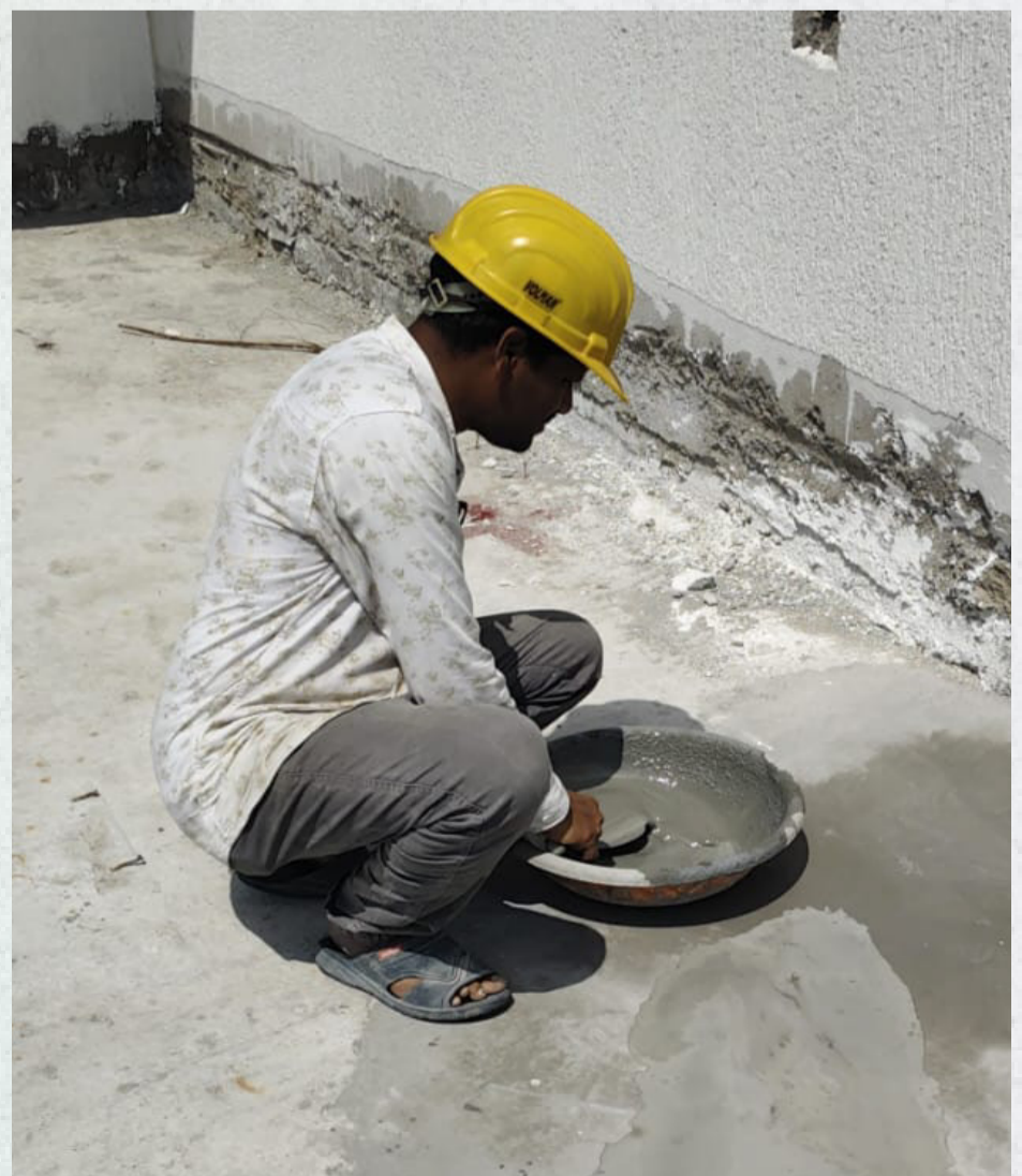
Terrace crack rectification works are in progress.
