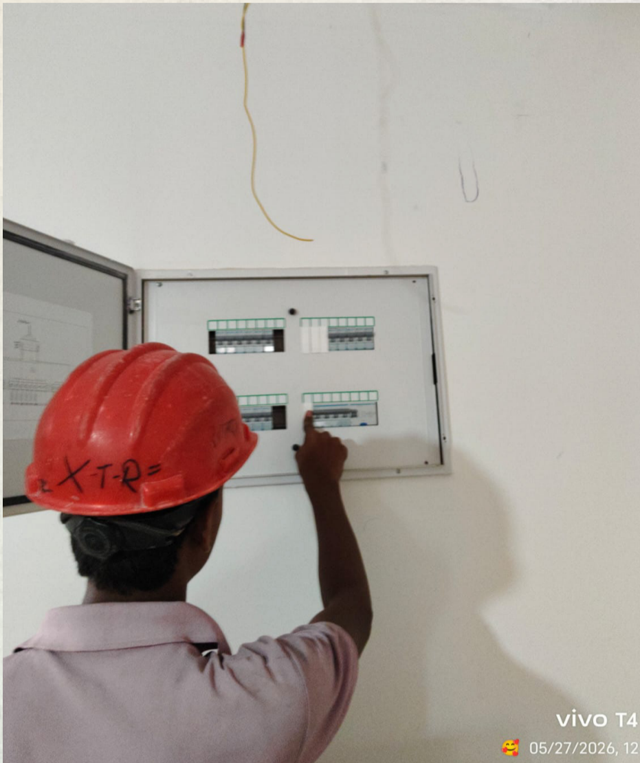
Electrical snag rectification works are in progress.
