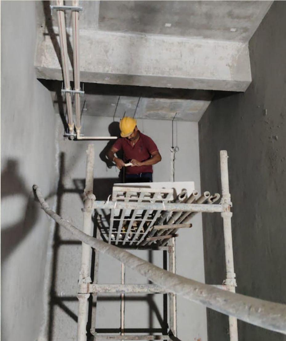
CPVC waterline works at Podium Level 2 are in progress.
