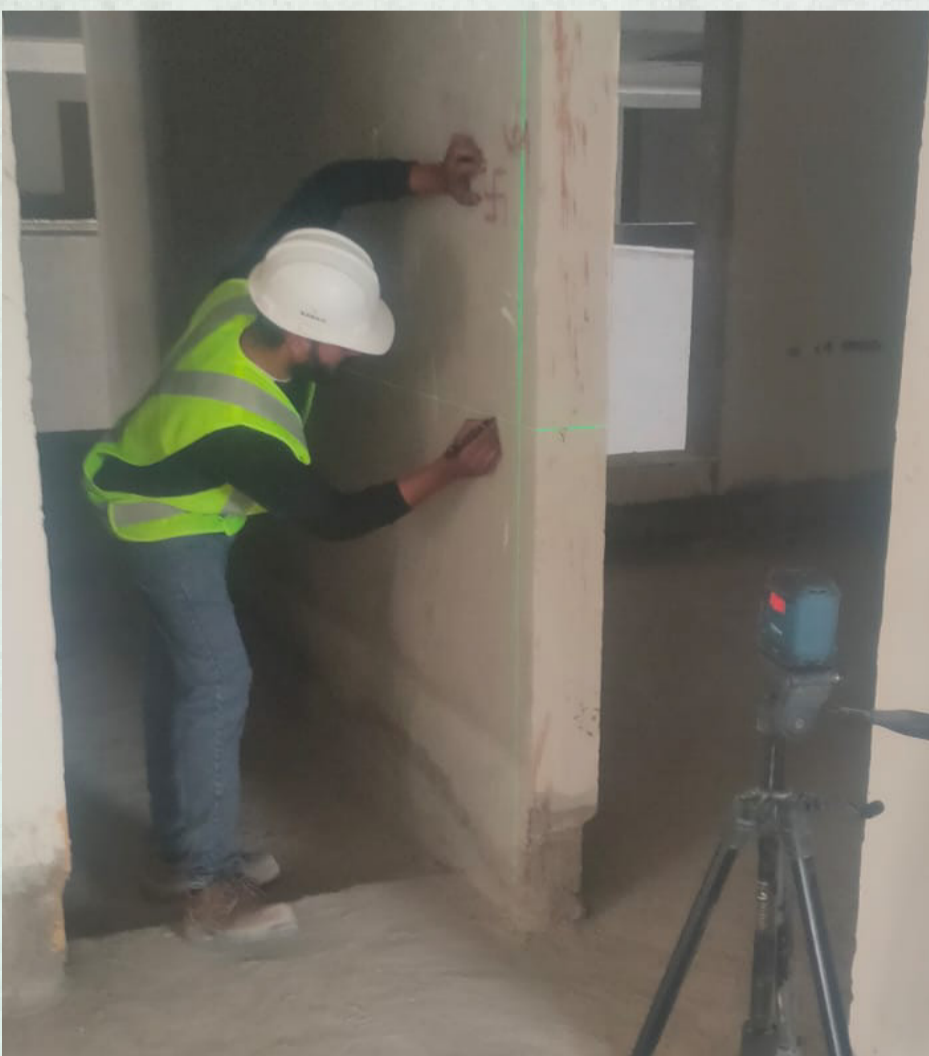
FFL(finished floor level) marking for Door measurements is underway in 5&6 series Flats.
