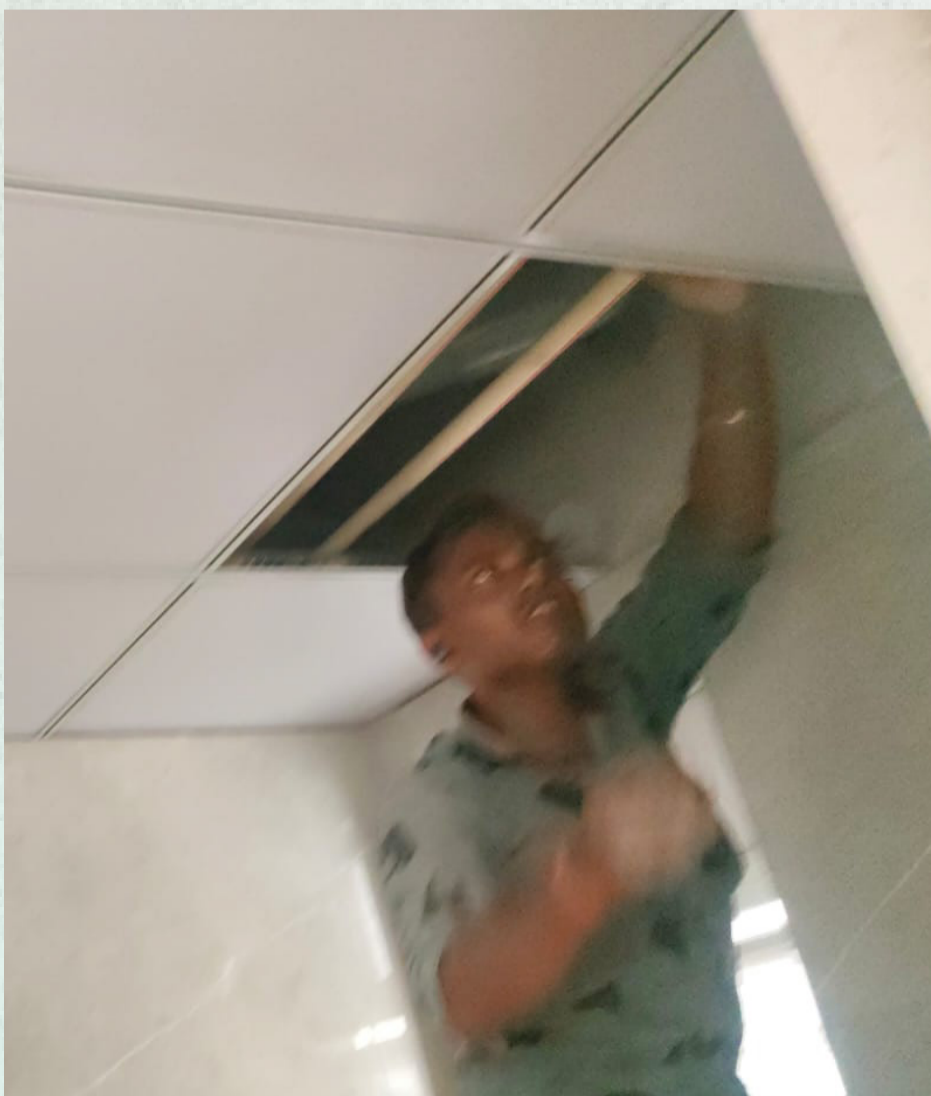
False ceiling panel fixing works are in progress.
