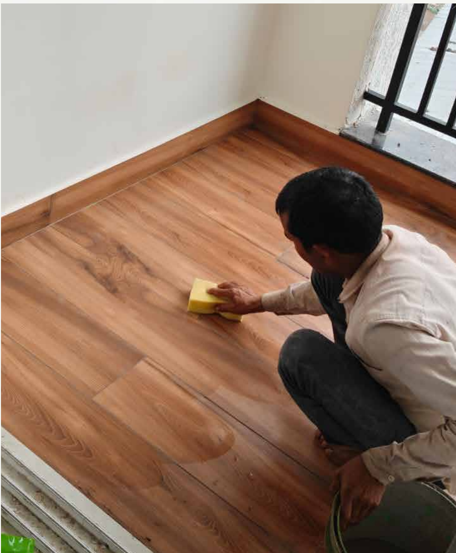
Grouting work for the tile flooring in the utility areas of the 3-series flats is in progress.
