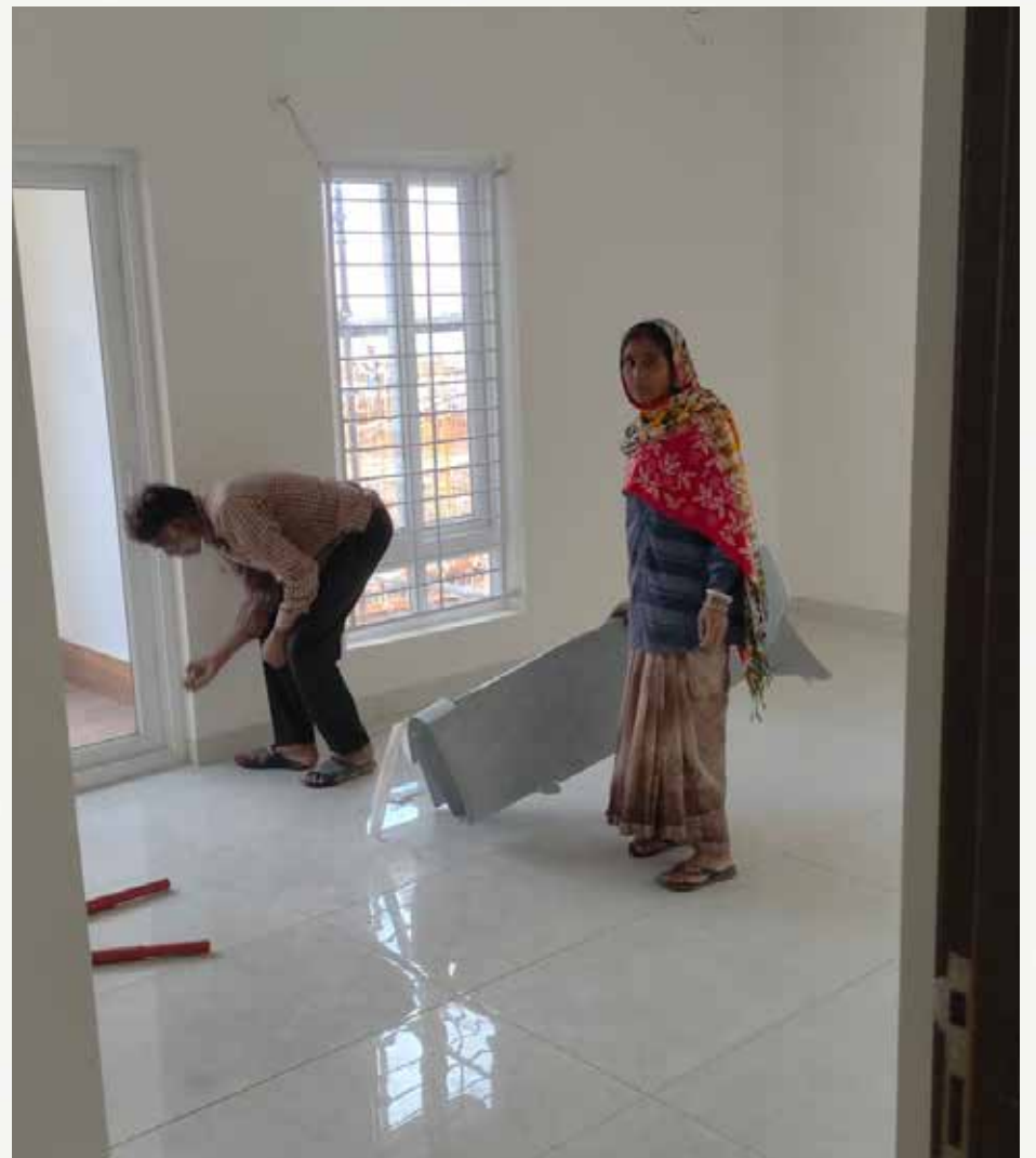
Pre-handover housekeeping works are in progress.
