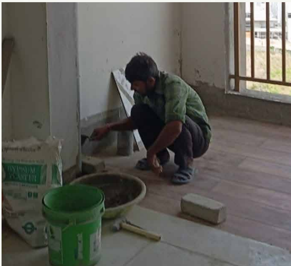
L-shaped brickwork in progress at the 6th series balcony area for V-board coping.
