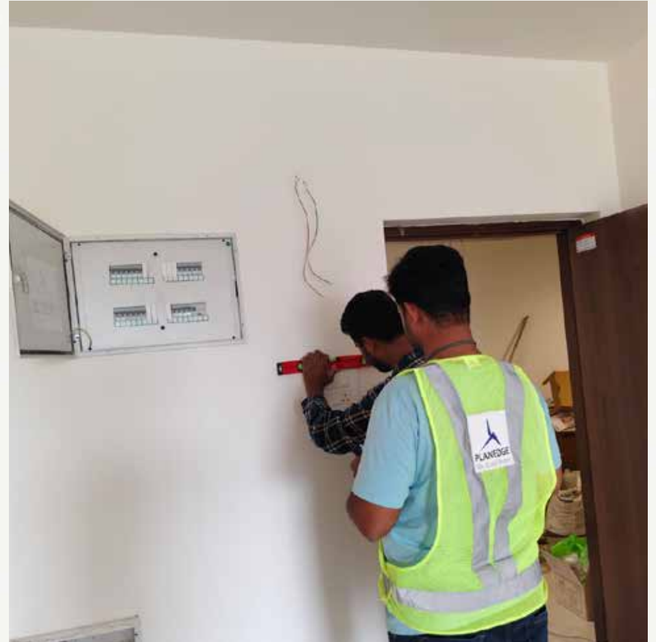
MEP snag testing is in progress in a flat on the 6th floor.
