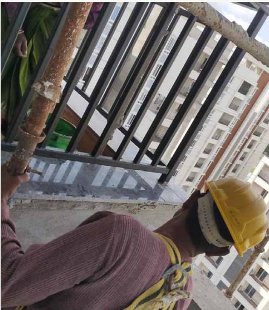
Granite bottom packing works in the west side balconies are in progress.
