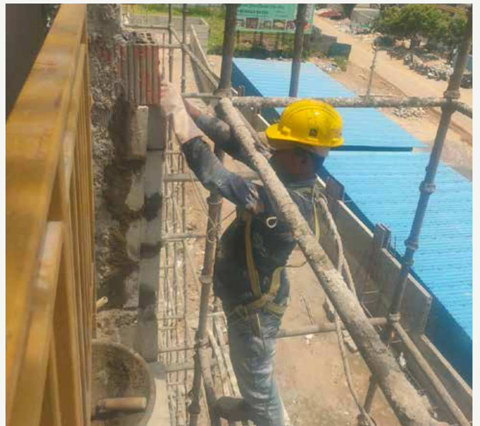
External elevation pin block works in the north side of the 13th series are in progress.
