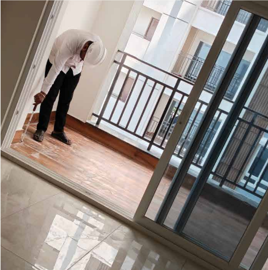
Grouting work for the tile flooring in the utility areas of the 3-series flats is in progress.
