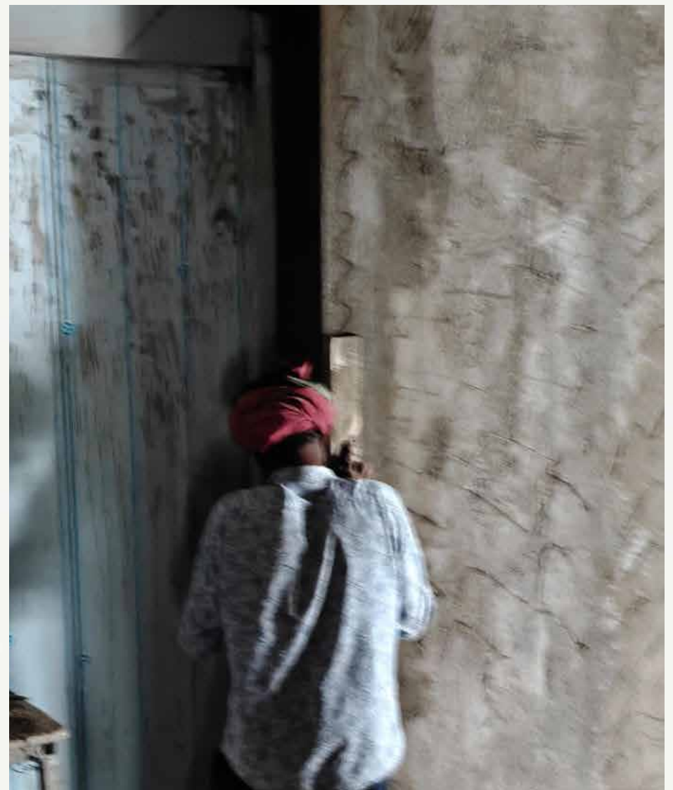
Plastering of cladding pins for Passenger Lift-2 is currently underway.
