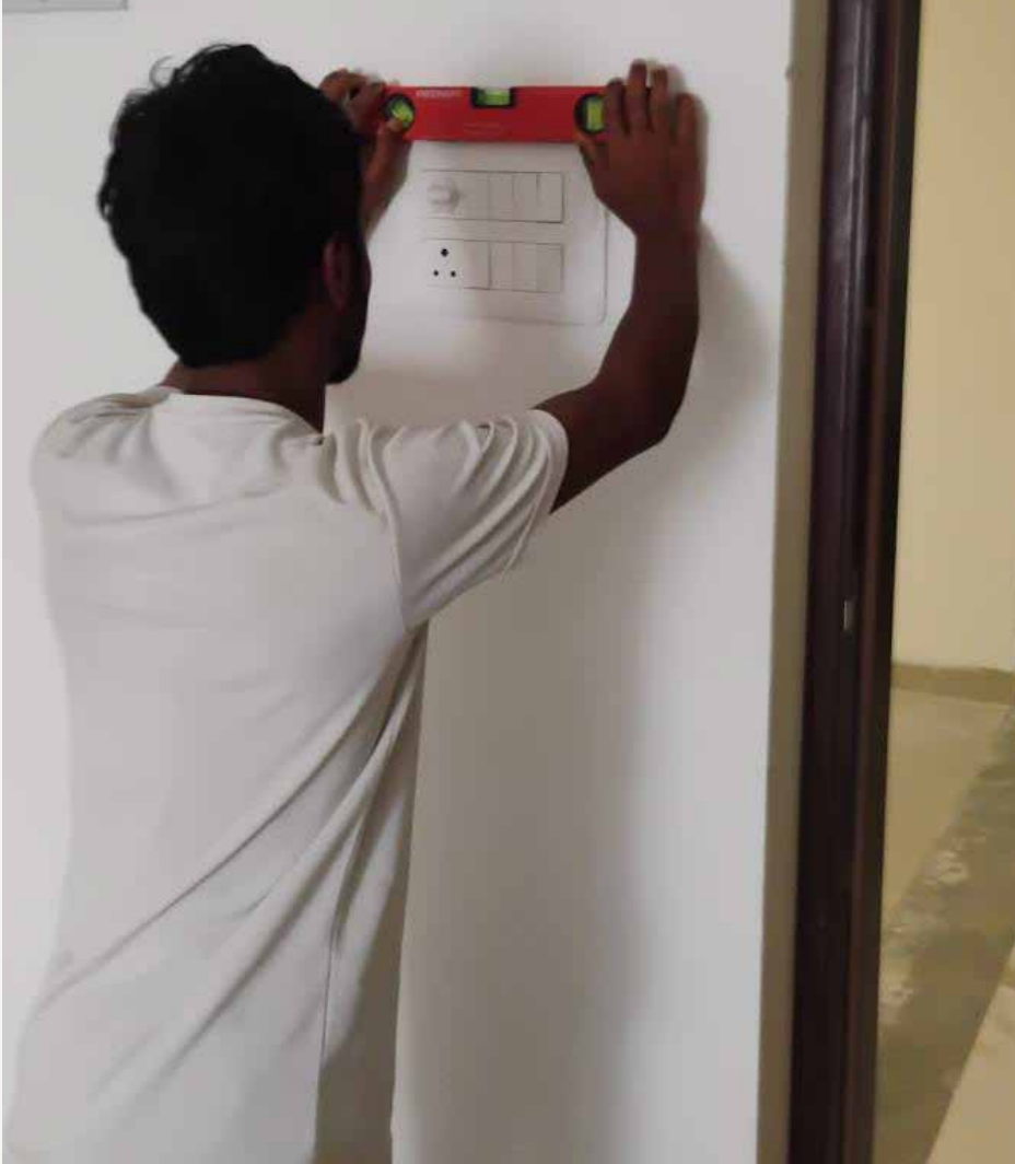
Electrical snag rectification works are in progress
