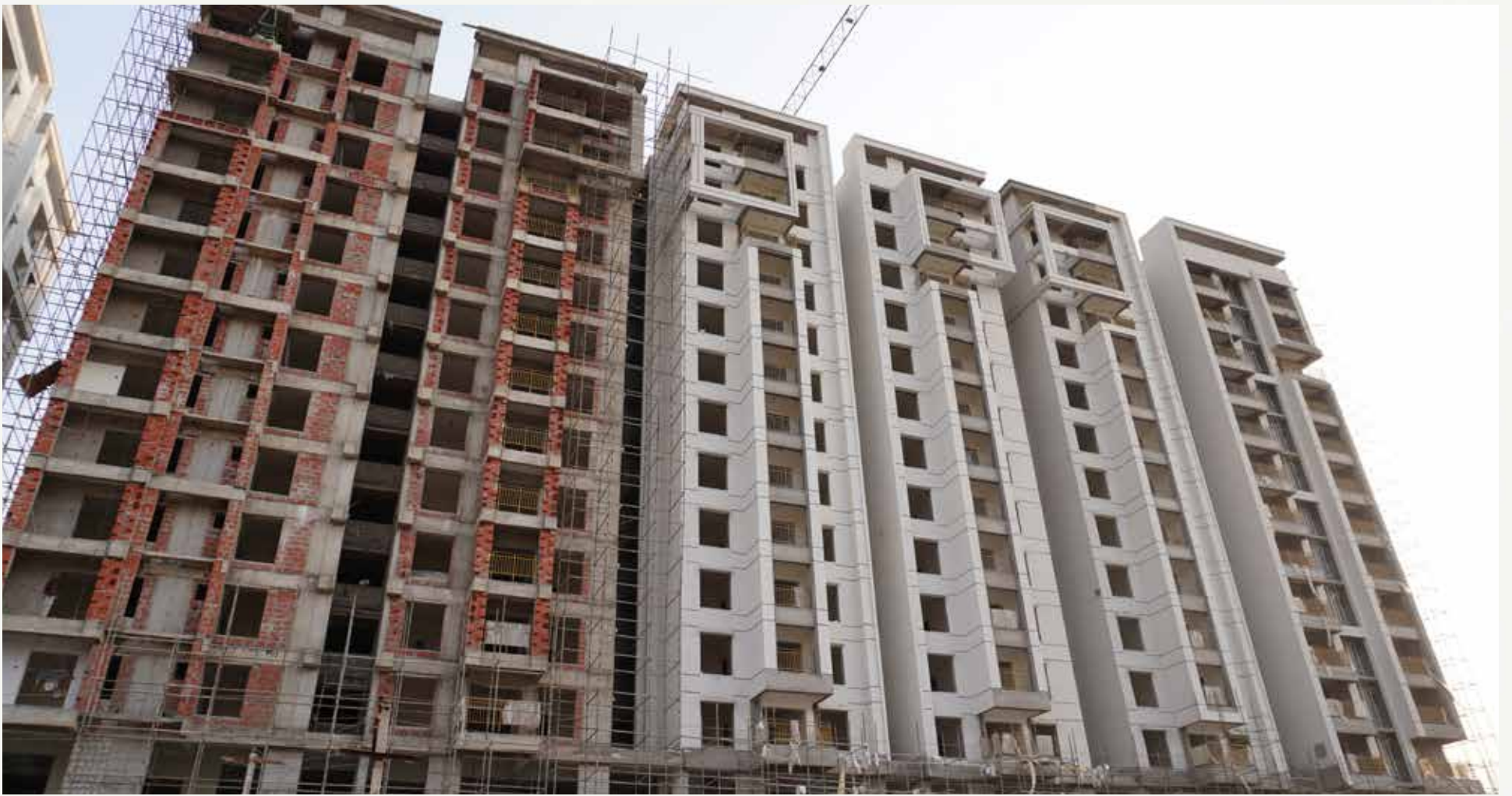
L-shaped brickwork in progress at the 6th series balcony area for V-board coping.
