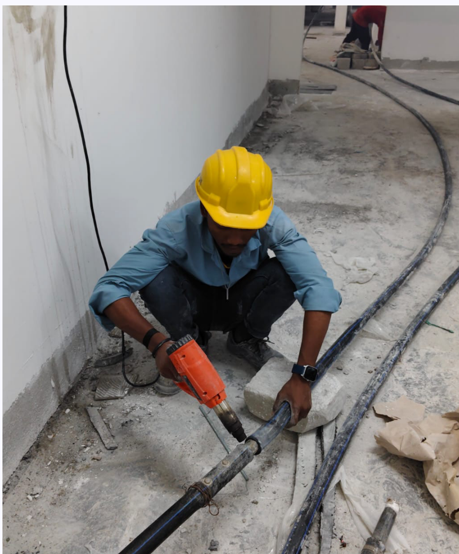
Basement 1 borewell pump HDPE pipeline joining work completed.
