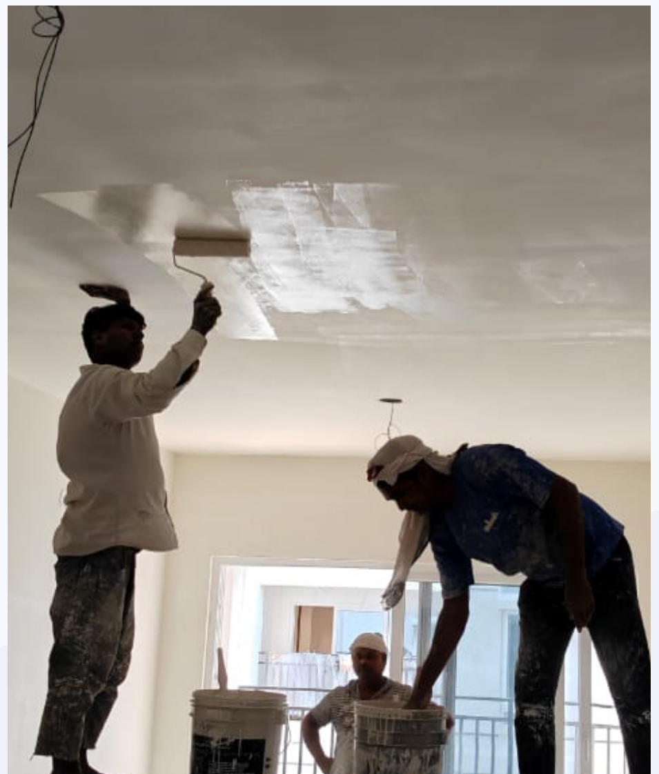
First coat painting work is in progress in the 11th series flats.
