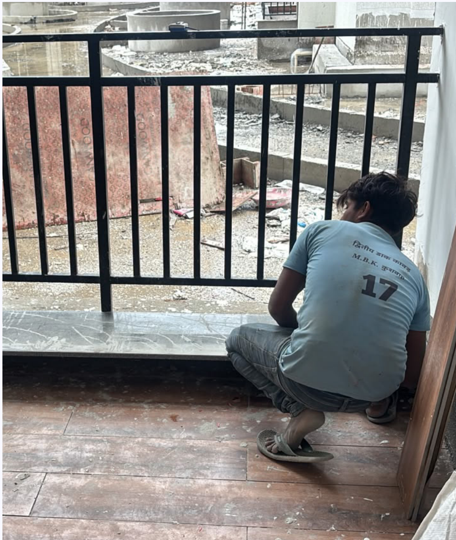
Granite installation is in progress in the 1-series flats.
