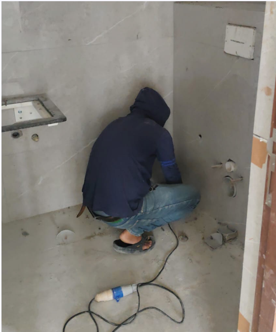
CP fittings and Sanitary fittings work is in progress.
