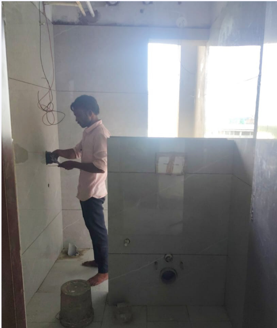
9th and 11th floor toilet, balcony and utility pipe packing works in progress.
