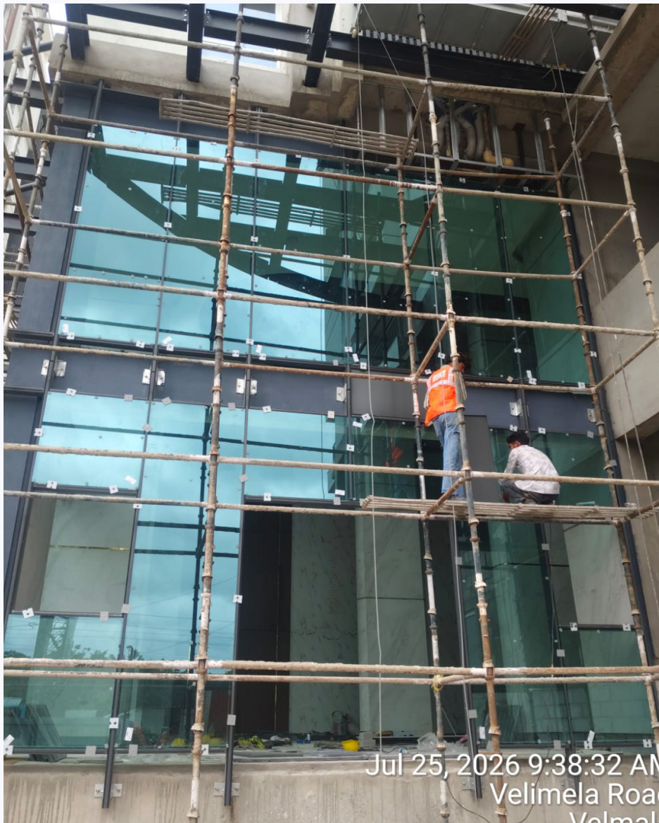
Tower - 4 entrance taking shape with glass installation works in progress.
