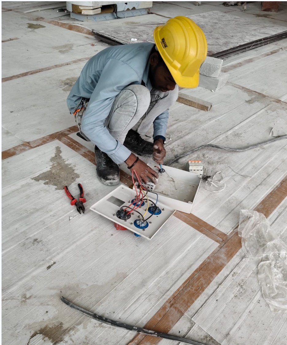
Entrance lobby area power supply board connection work in progress.
