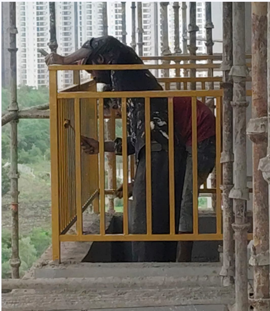
Railing sanding, surface cleaning, and primer application work in progress in a 10th floor flat.
