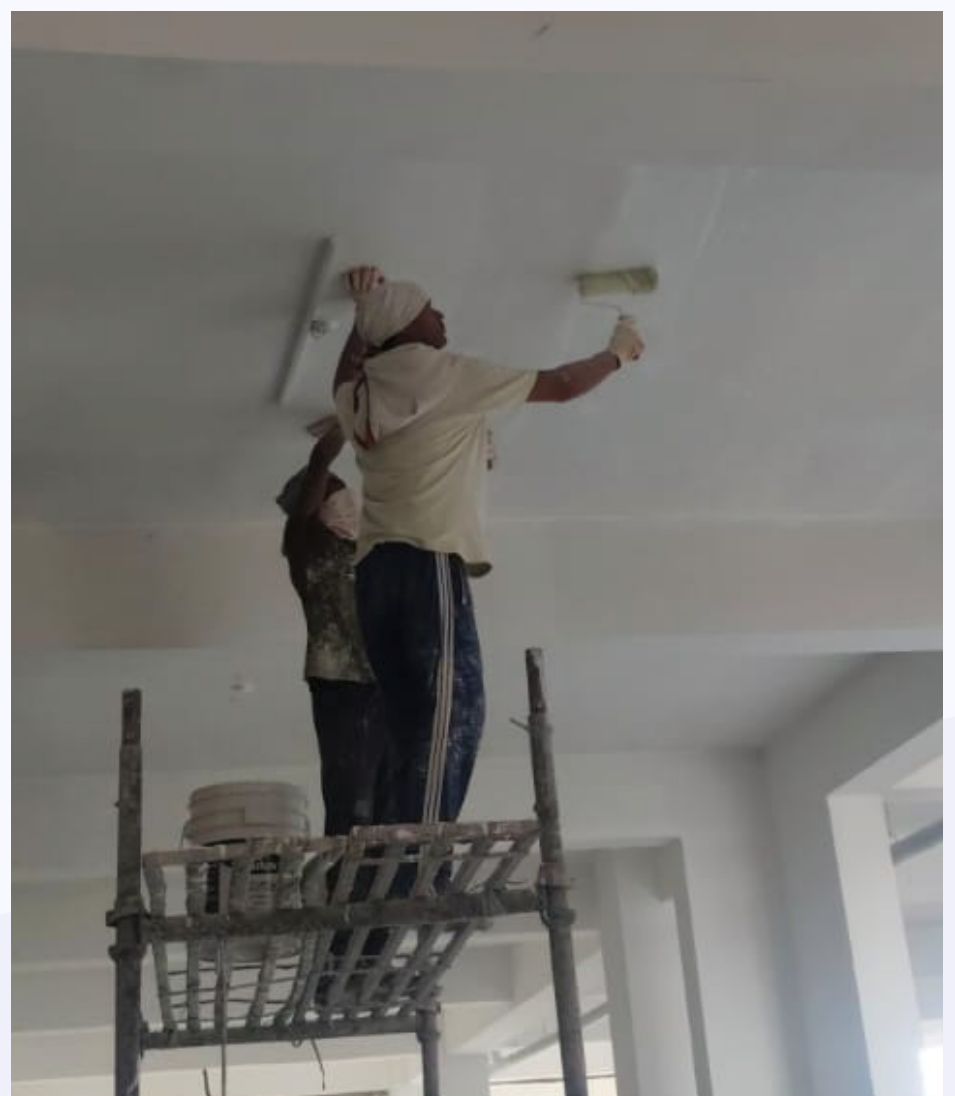
Primer application works in progress at Podium Level 1.
