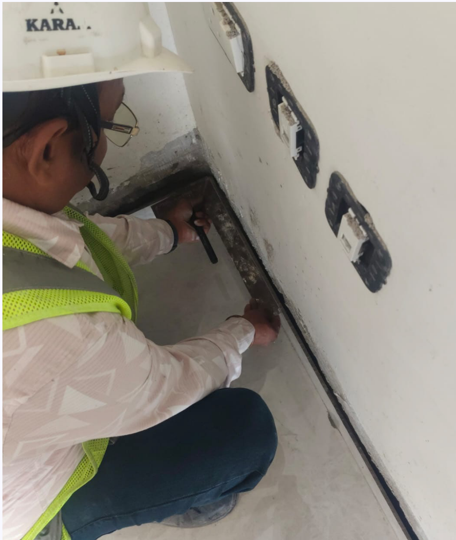
Post tile-laying inspection in progress including skirting right-angle, alignment and surface undulation checks.
