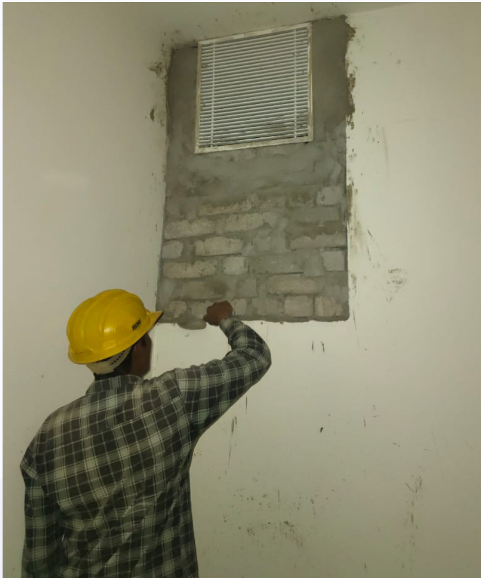
Podium shaft block masonry and plastering works underway.
