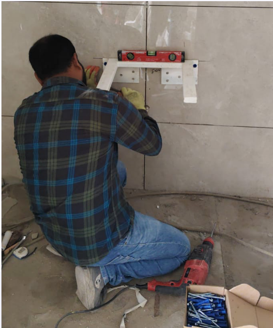
Basin Bracket Installation Underway Across Series 10 & 11 Flats.
