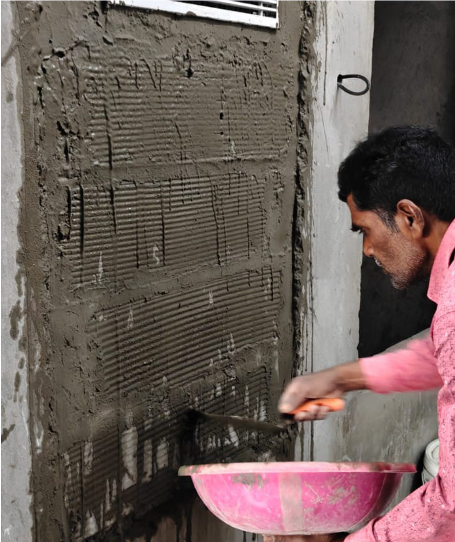
Putty touch-up works in progress in one of the 11th series flats.
