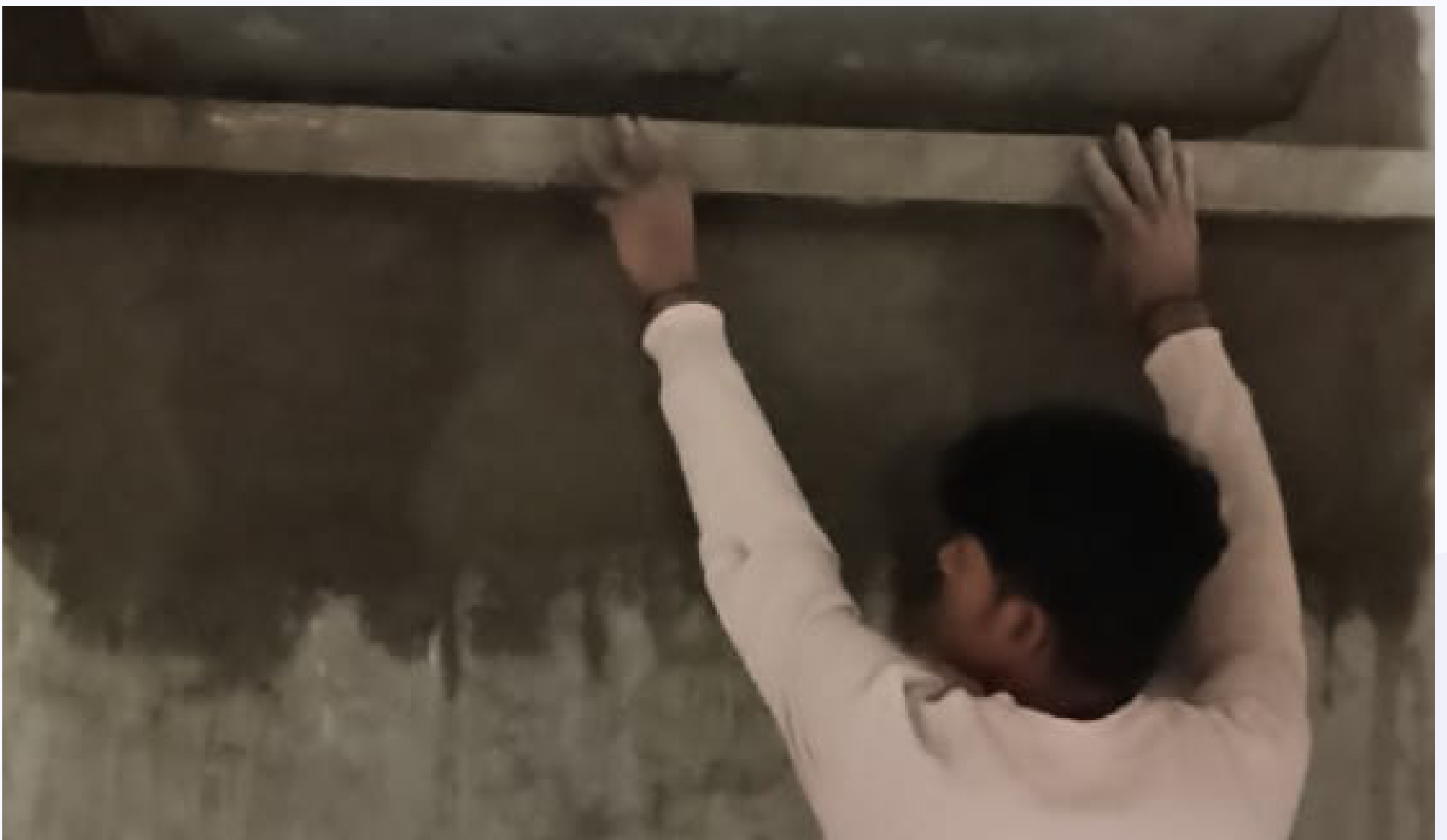
Basement 1 STP extra plumbing raft closing works and plastering completed.
