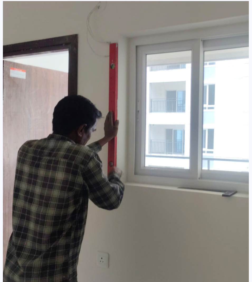
Post snag inspection, the window side rectification work is in progress.
