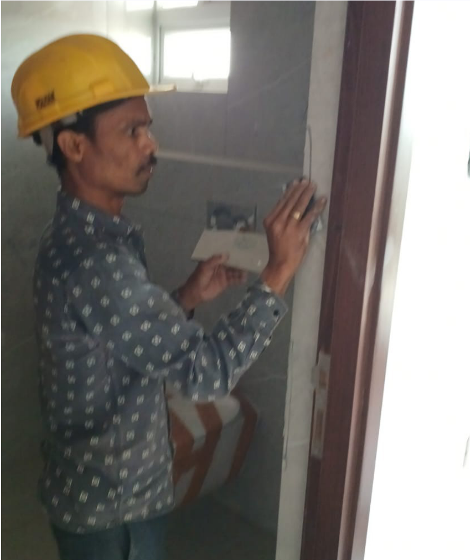
Tiles snag point rectification work in progress in a 12th-floor flat.
