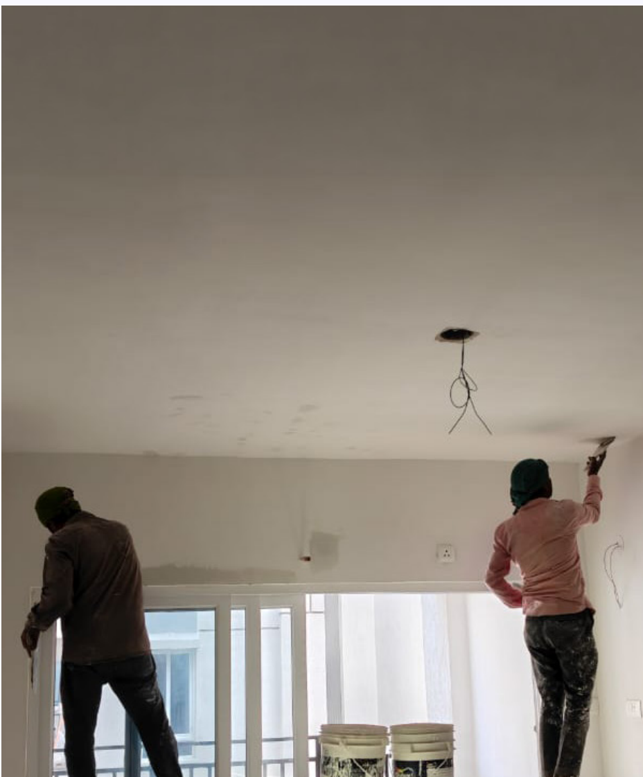
Putty touch-up works in progress in one of the 11th series flats.
