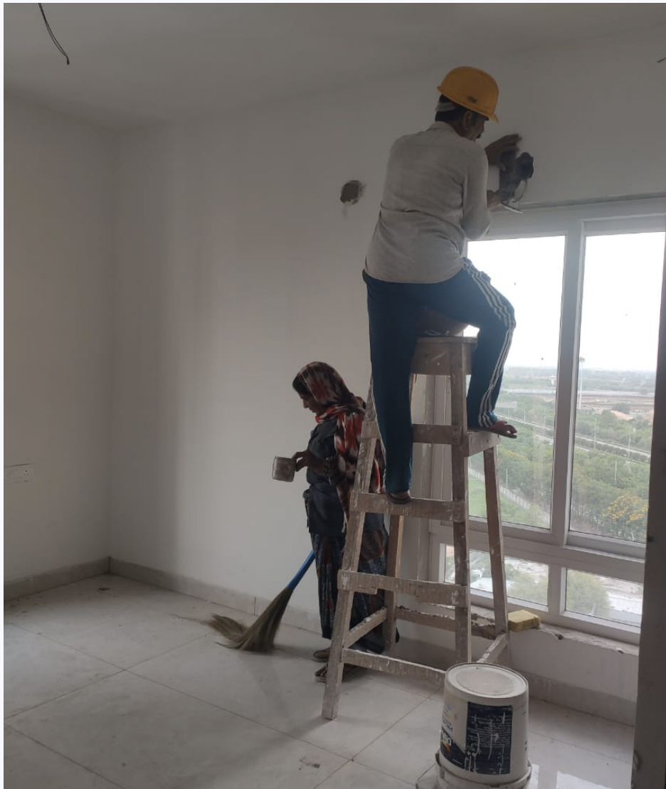
Electrical Junction Box Packing is in Progress.
