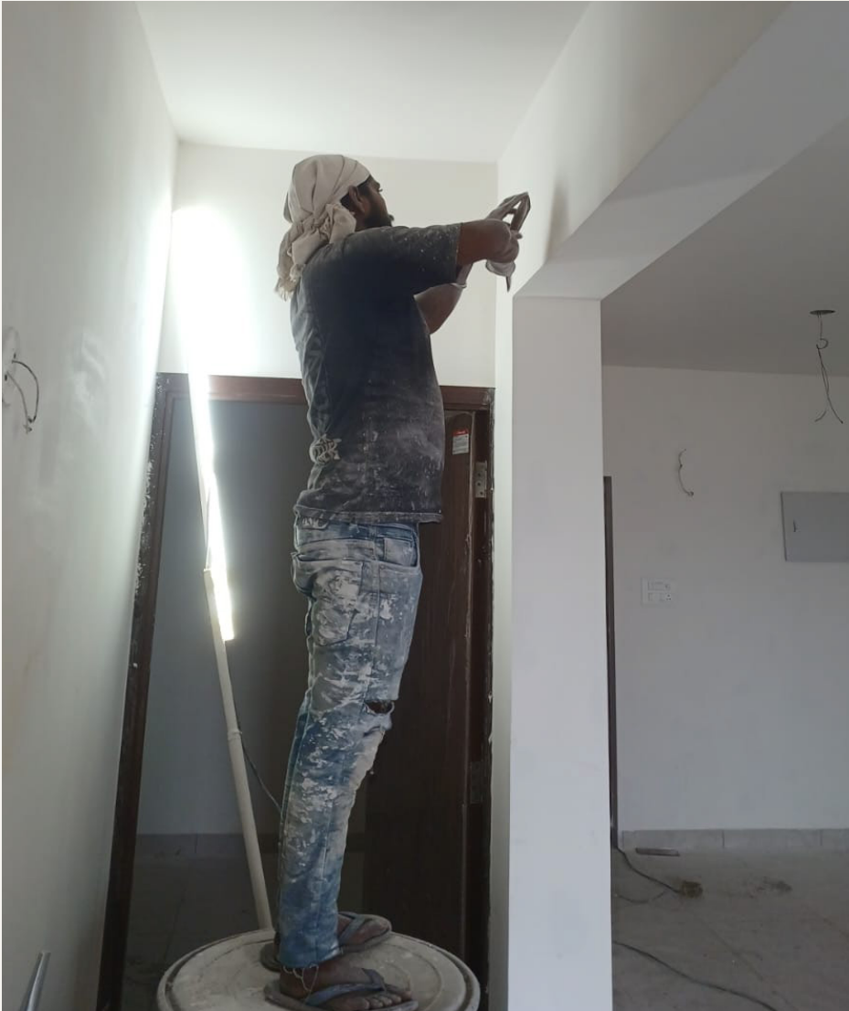
2nd coat paint touch up work is in progress.
