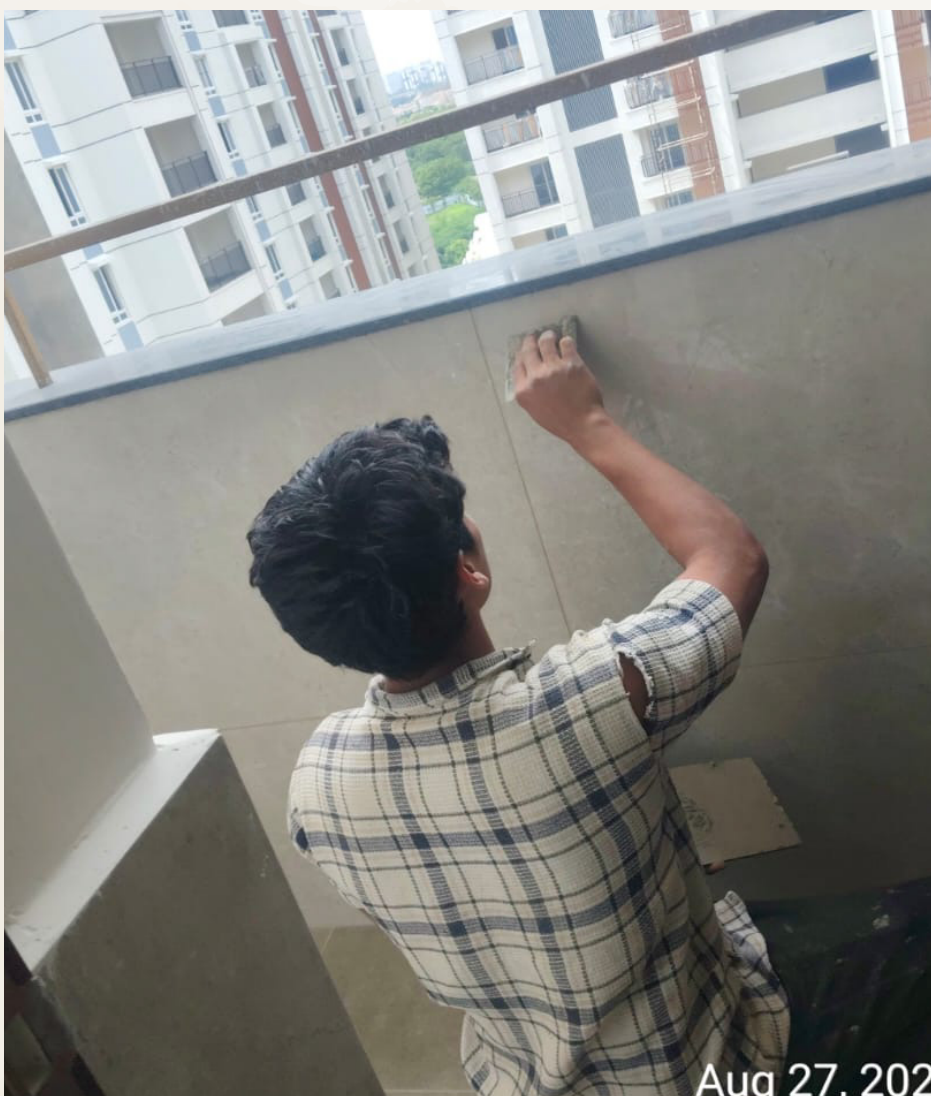
T- 4 – Tile snag point rectification work is in progress.
