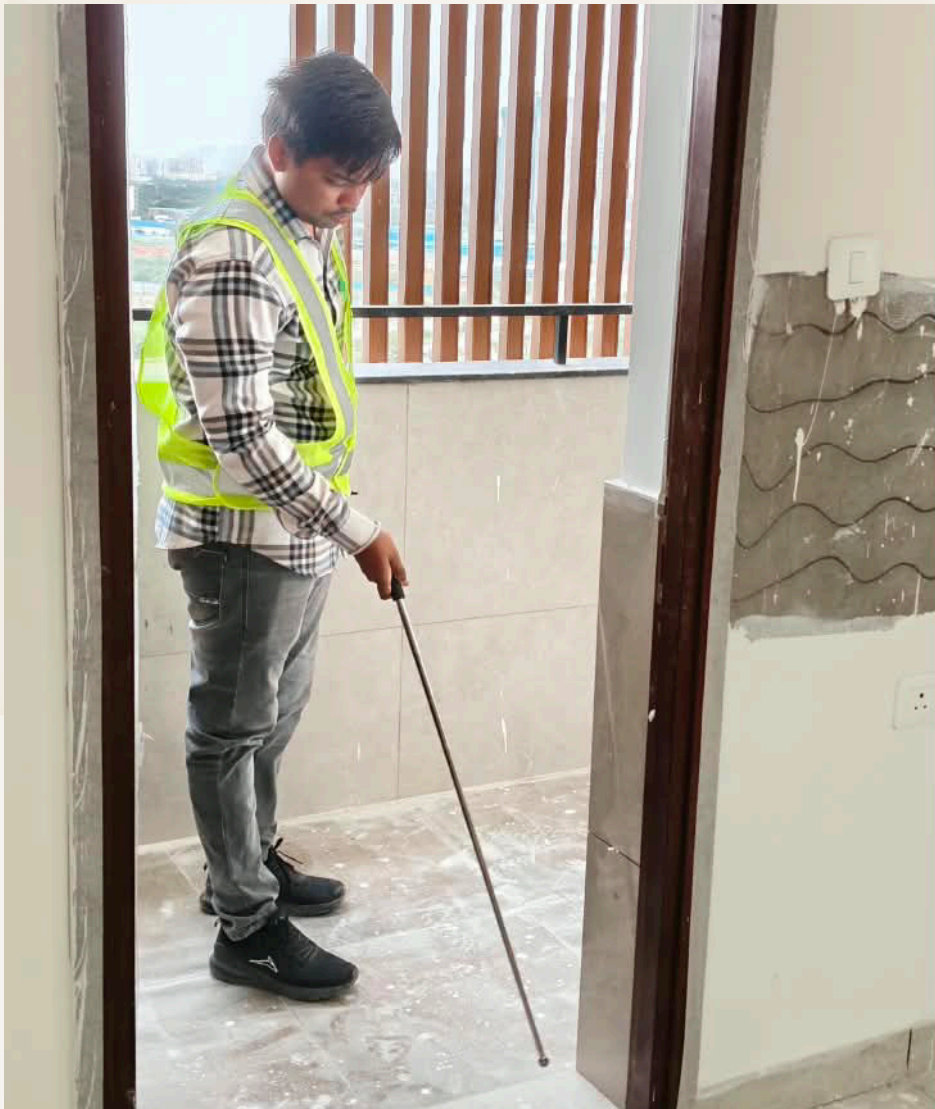
Third-party snag inspection is in progress.
