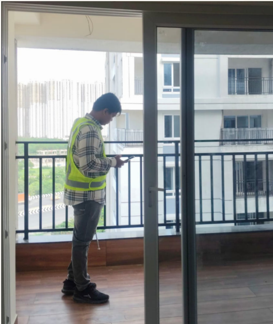
De-snagging inspection is in progress
