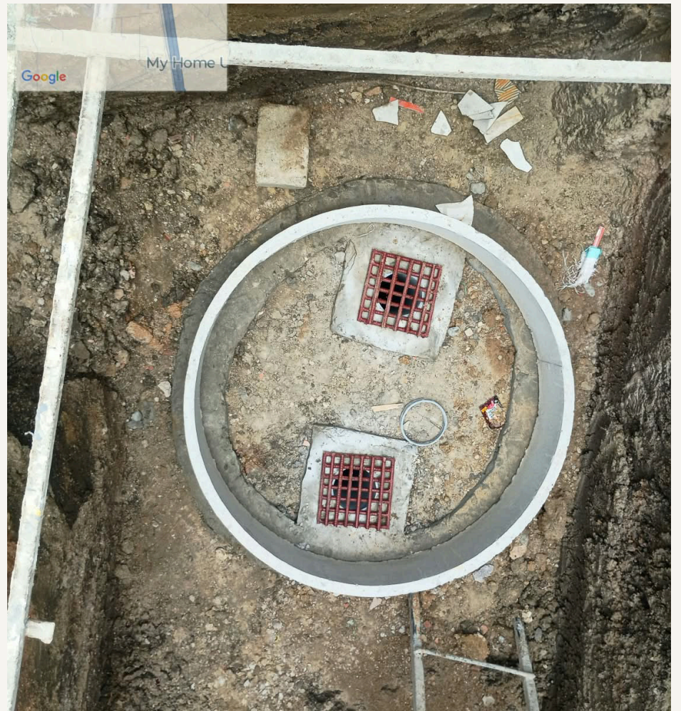
RCC recharge pit chamber with internal grating completed.
