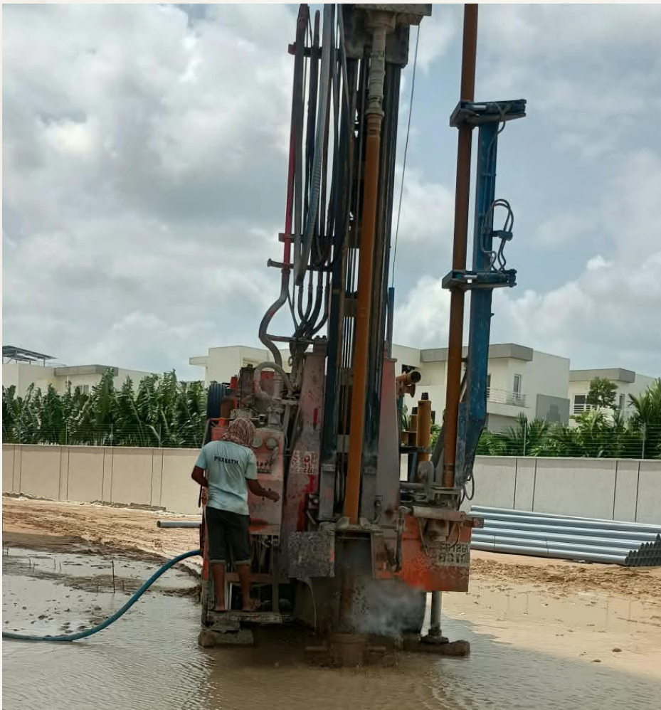
Drilling the recharge pit.
