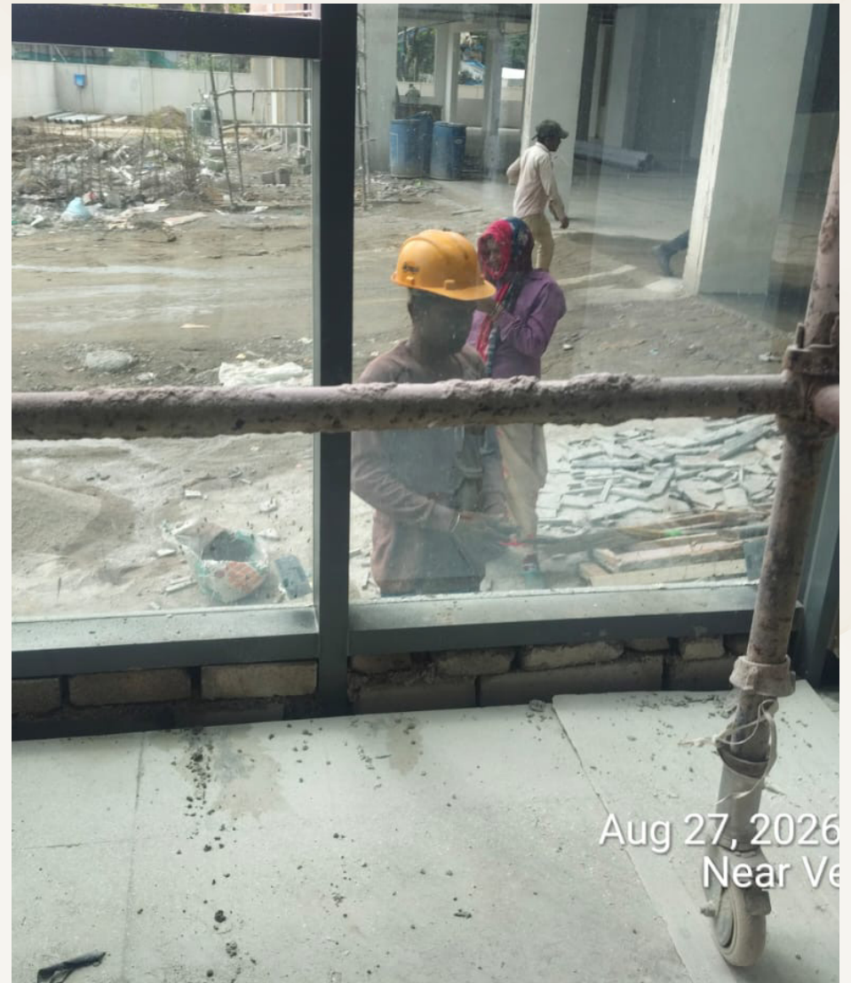
Tower 4 entrance lobby – plastering work for the Glass bottom block is in progress.
