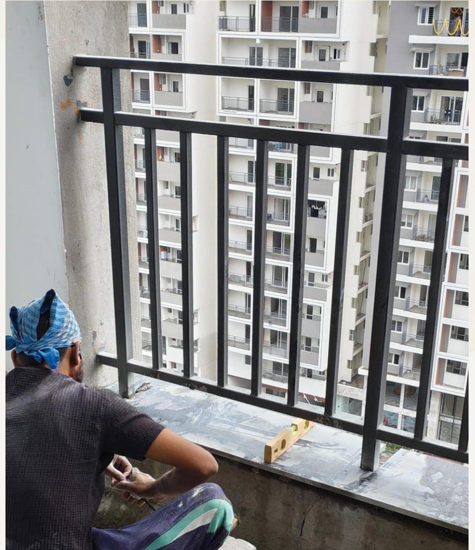
Granite fixing for the balcony railing is currently underway.
