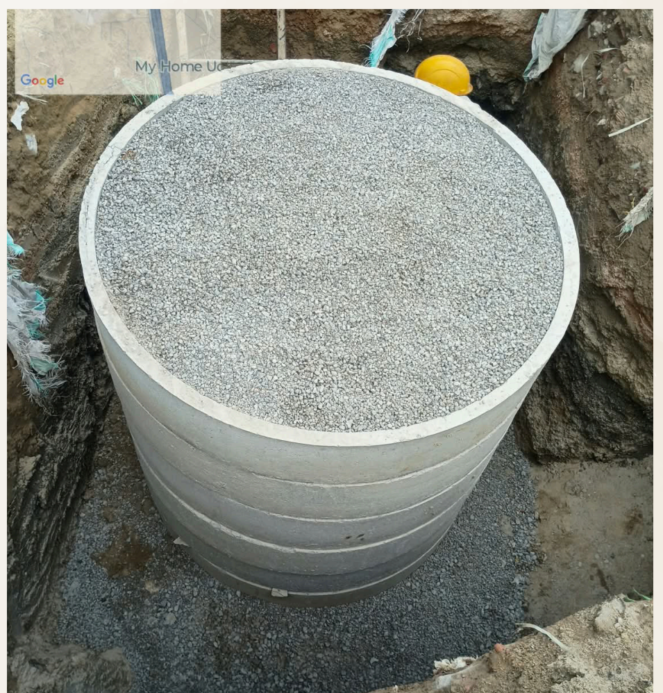
Recharge Pit – Filter Media Installation.
