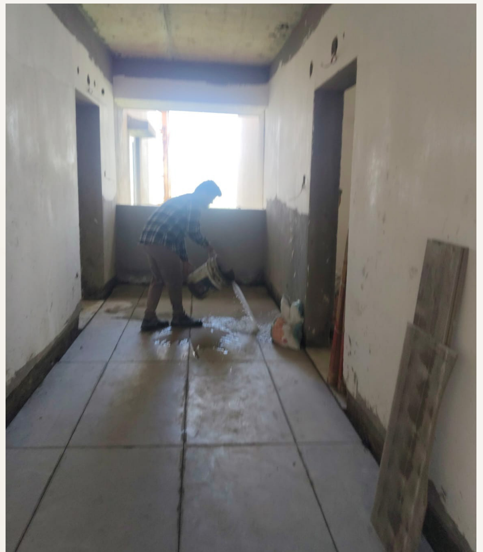
11th floor corridor tile curing work is currently underway.
