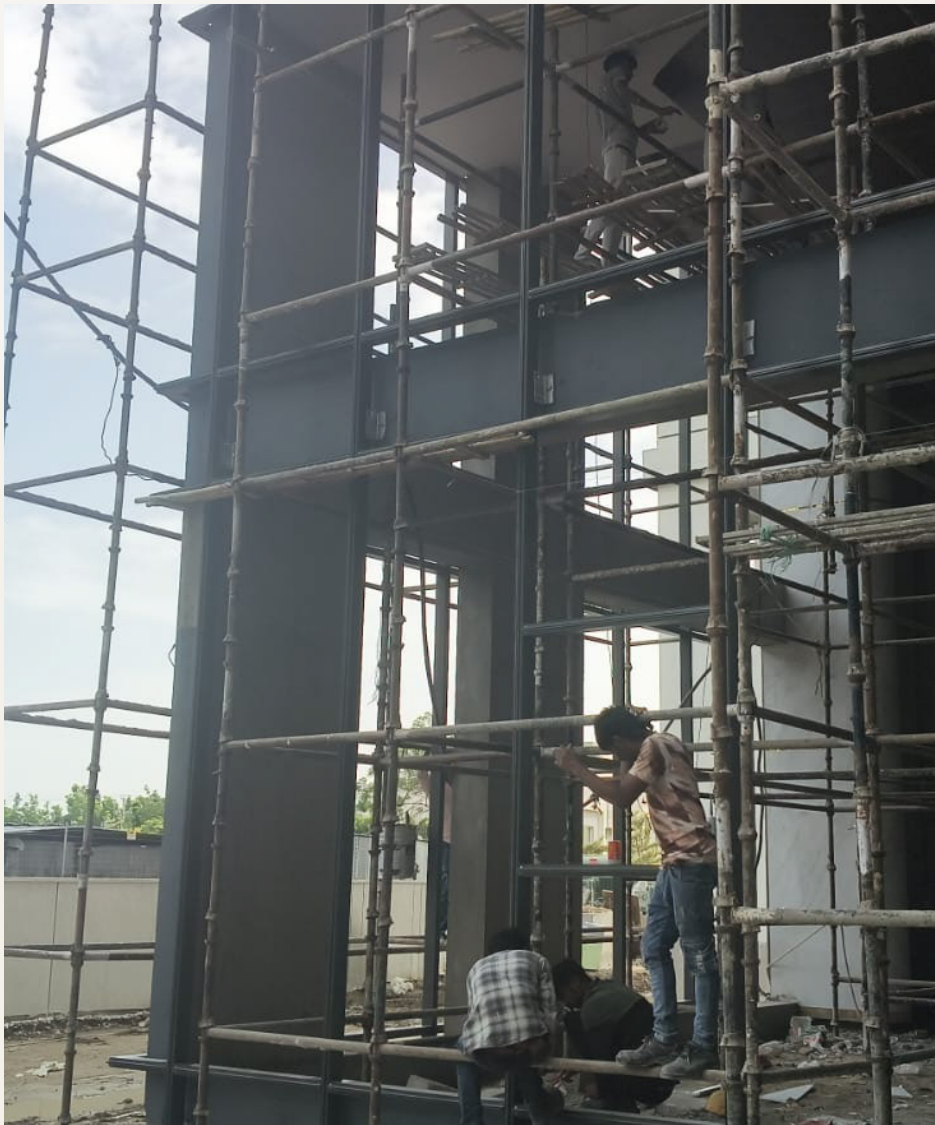
T2 entrance lobby façade work is in progress.
