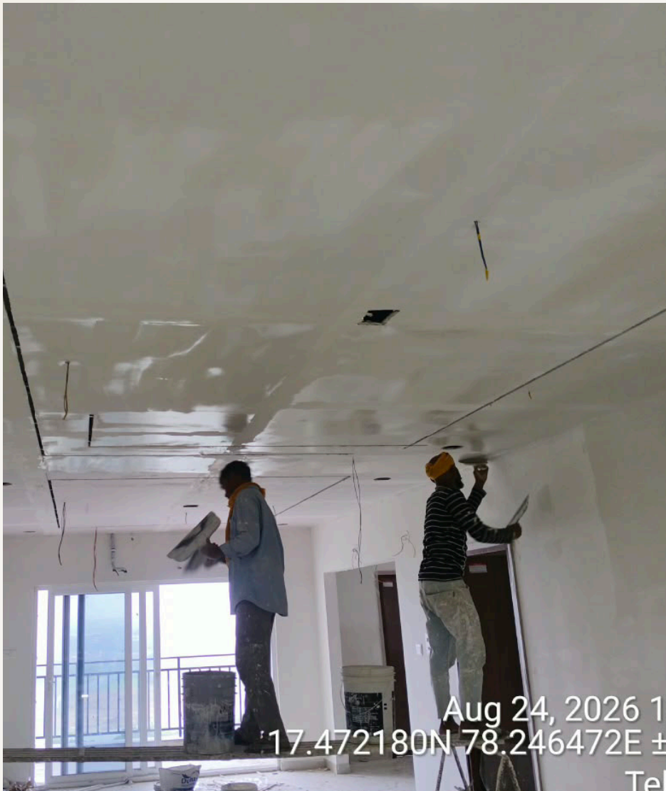
Ceiling putty application work is in progress in a 12th floor flat.
