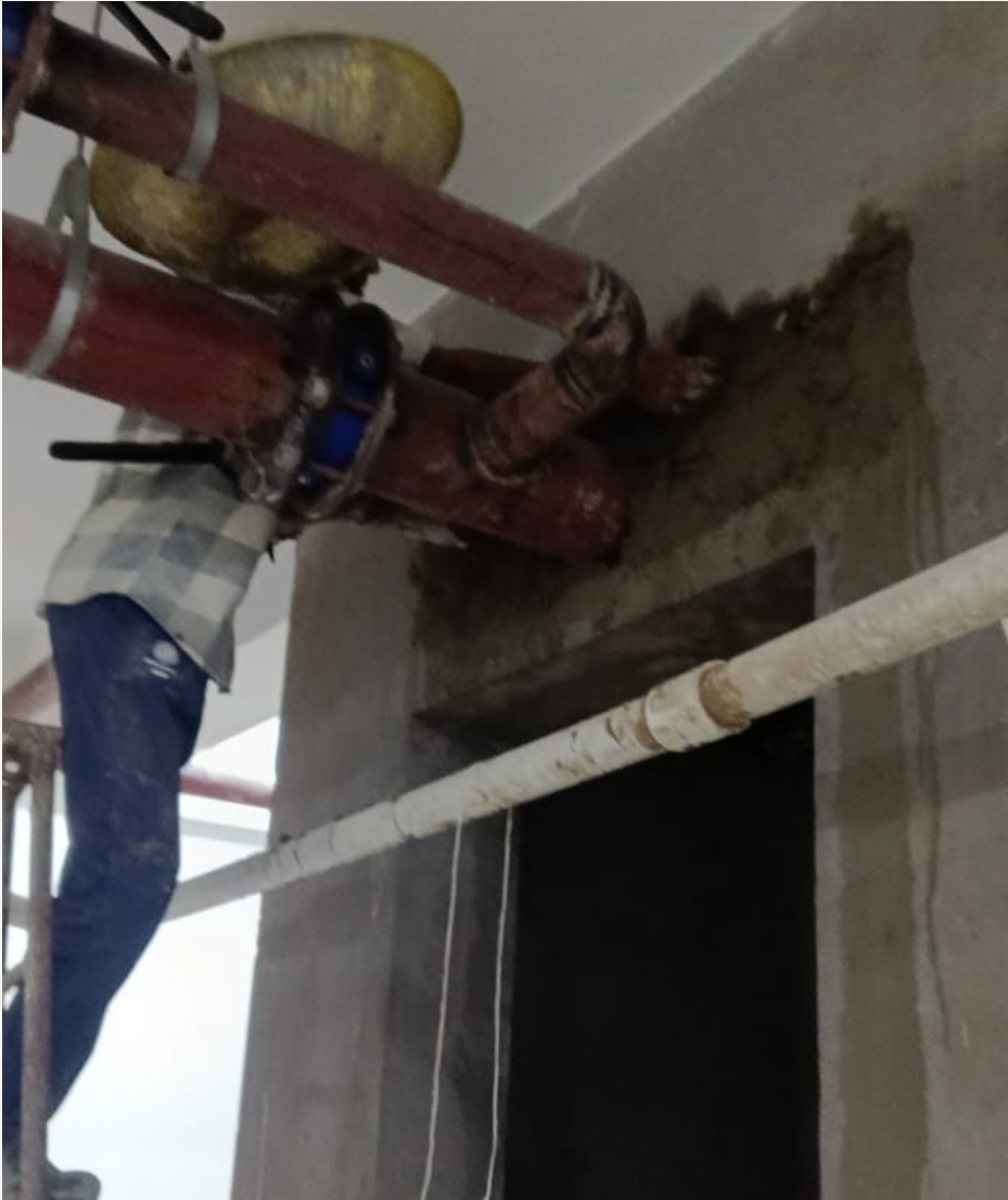
B1 – Additional plumbing shaft closure and plastering activities are underway.
