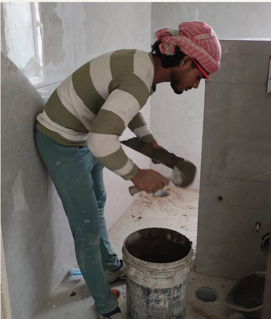
Toilet skirting tile installation is currently underway.
