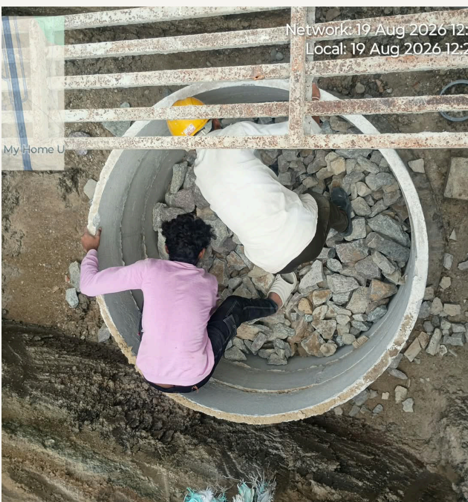
Stone aggregate filling in the recharge pit is in progress.
