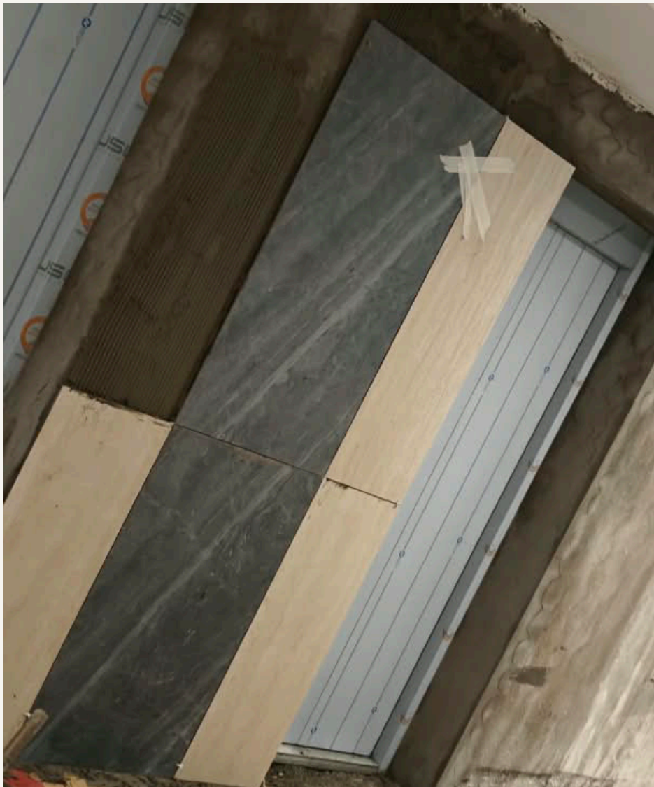
T2 passenger lift cladding tile laying work is in progress.
