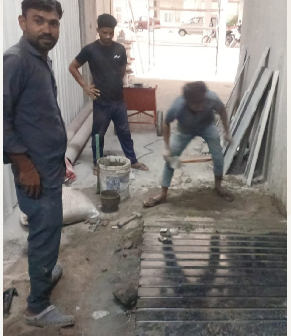
P1 floor entrance ramp area – granite laying work is in progress.
