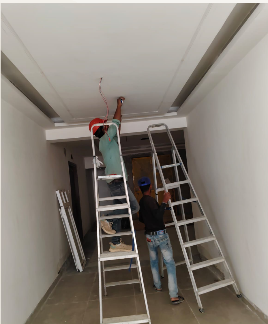
11th-floor corridor lighting point marking work is in progress.
