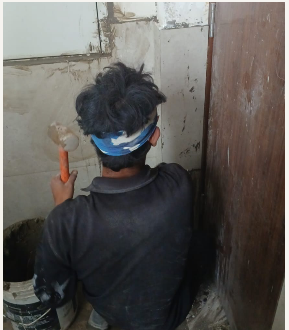
Tile snag rectification work is in progress in a first floor flat.
