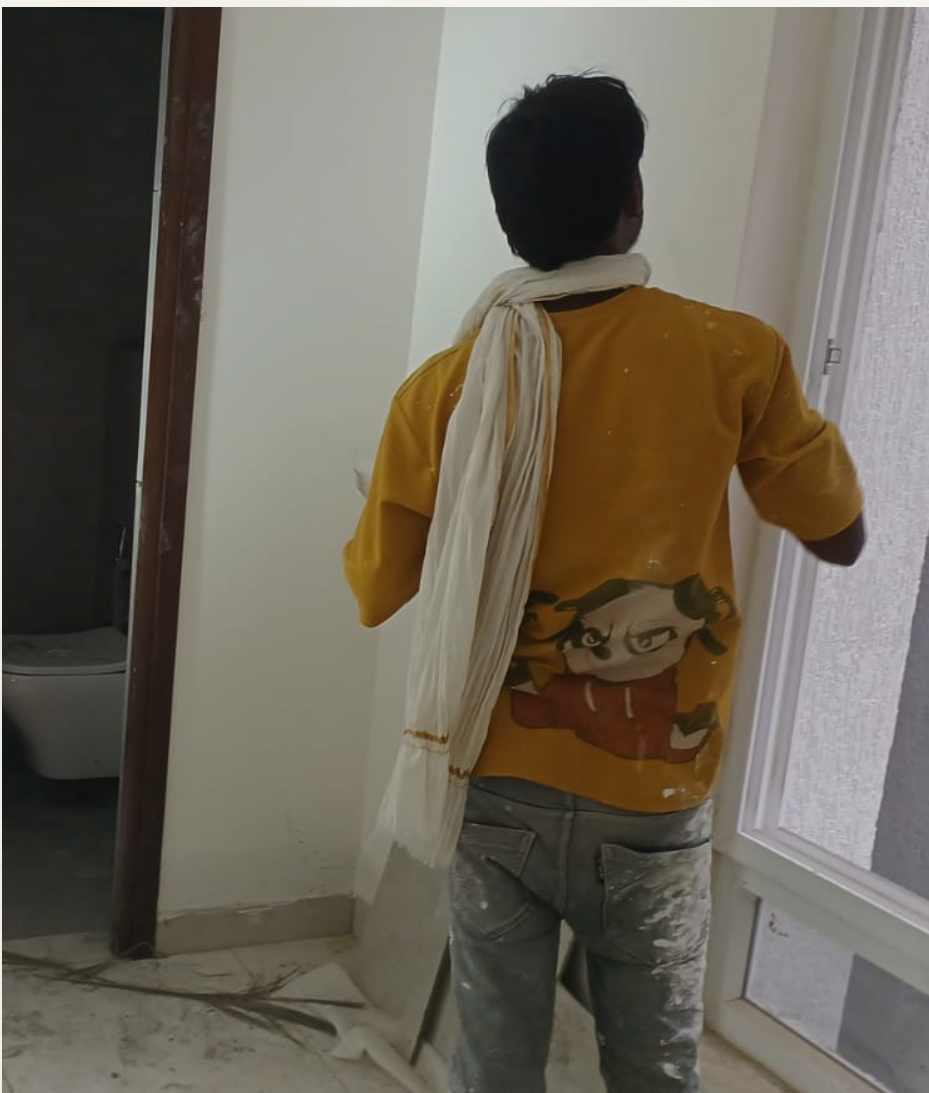
2nd coat painting work is in progress in a flat in the 7th floor.
