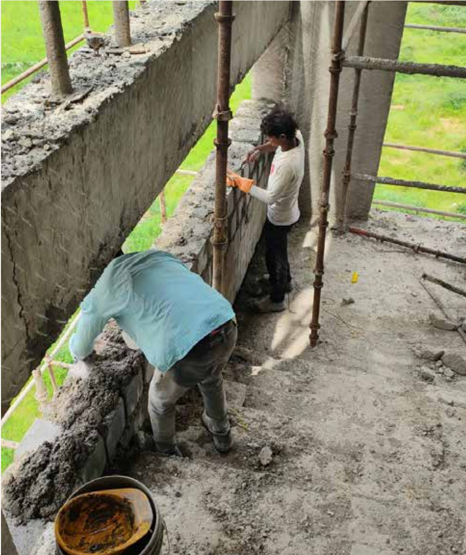
5th Floor-brick work is in progress.
