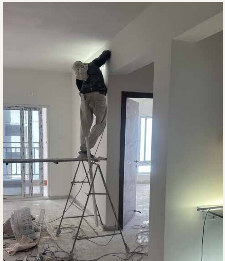
Surface sanding work in progress following the first coat of painting.
