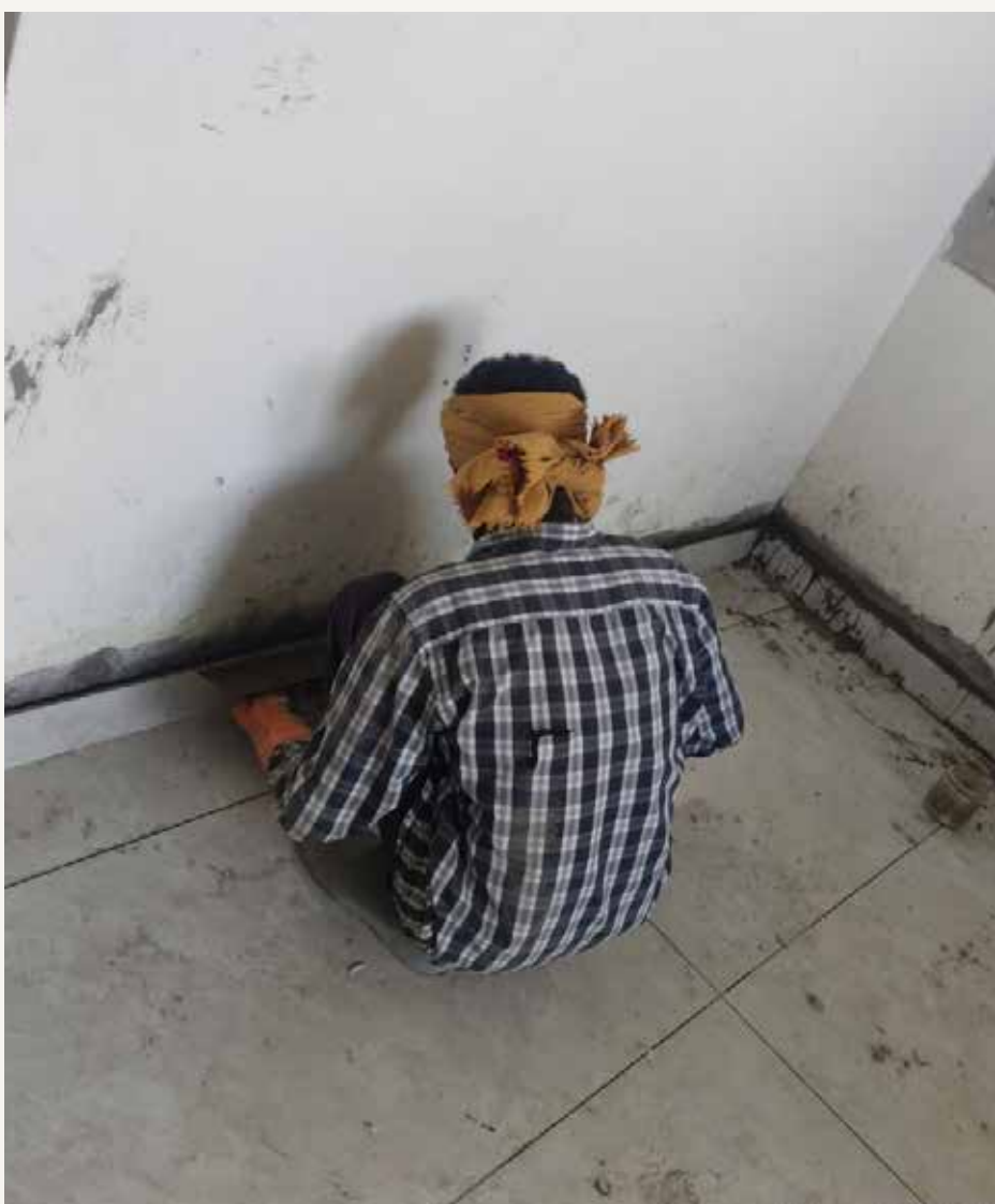
Cement slurry filling above the skirting - is in progress in a flat on the 7 floor.
