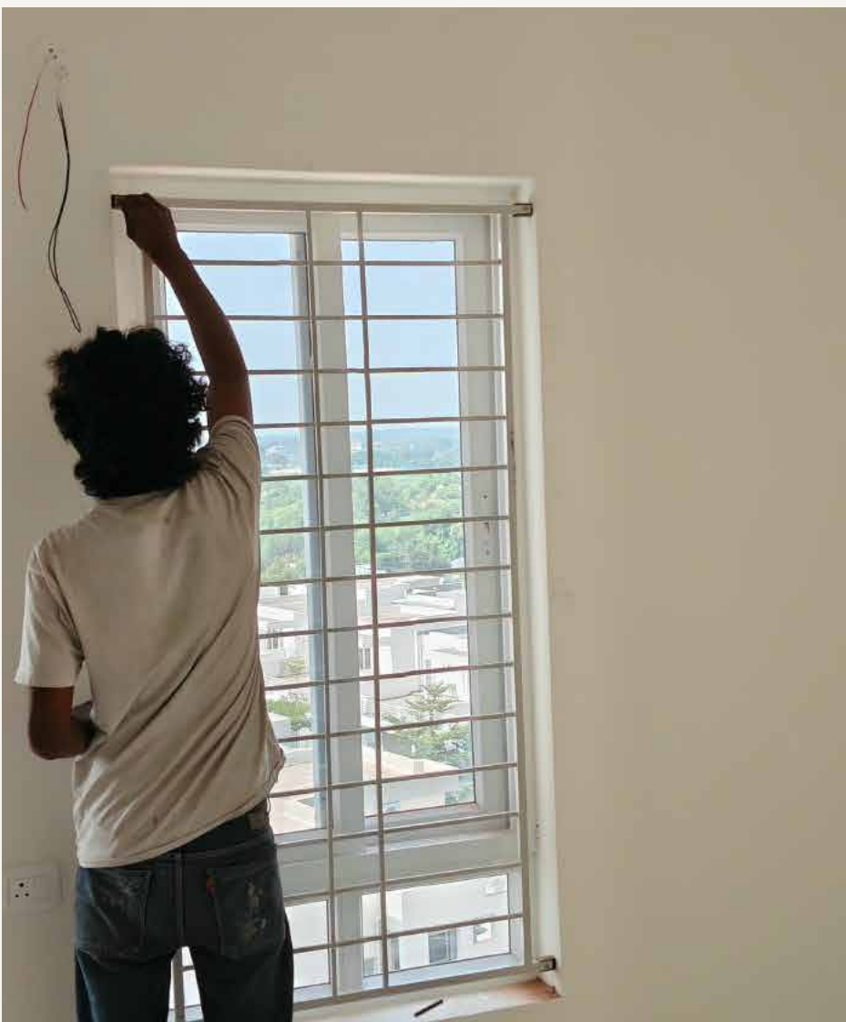
Fixing of grills for the windows is in progress in a flat on the 4th floor.
