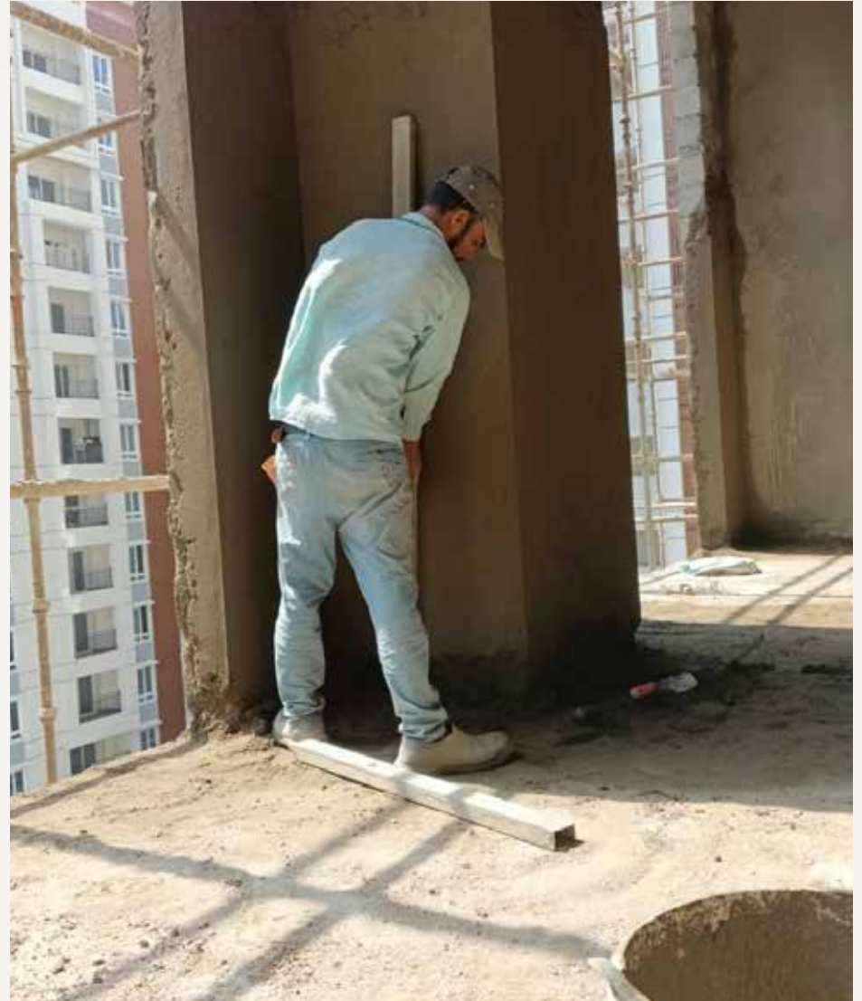
Wall marking for the passenger lift area is in progress.
