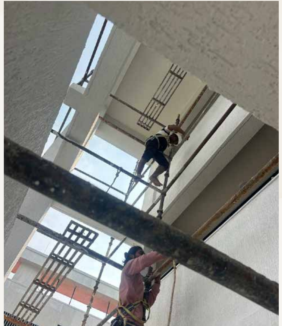
Surface sanding work in progress following the first coat of painting.
